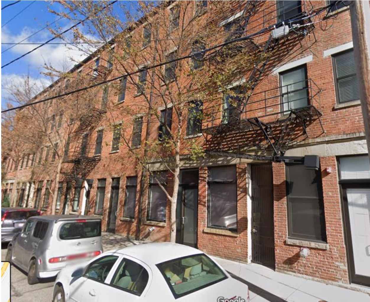
Figure 2. Street view of 1120 Broadway Street. Image from Google.
