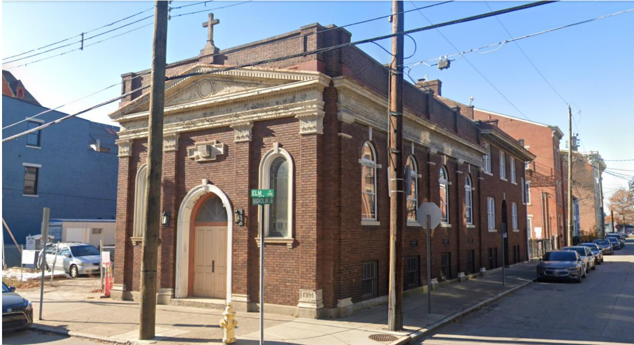
Figure 1: View of 1419 Elm Street. Google Street Views Nov 2020.
