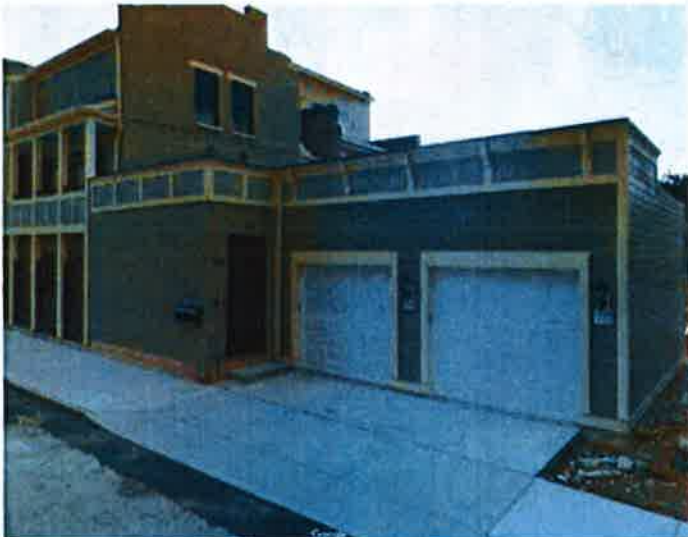
Alley facing garage Addition [Example from Odean Street building]
