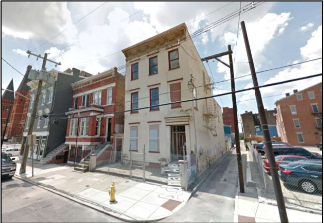
Figure 2. Image of subject property facing southwest ca. 2017. Image from Google.
