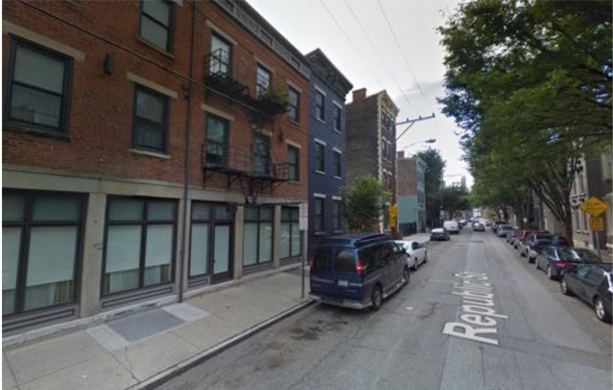
Street view looking south east
