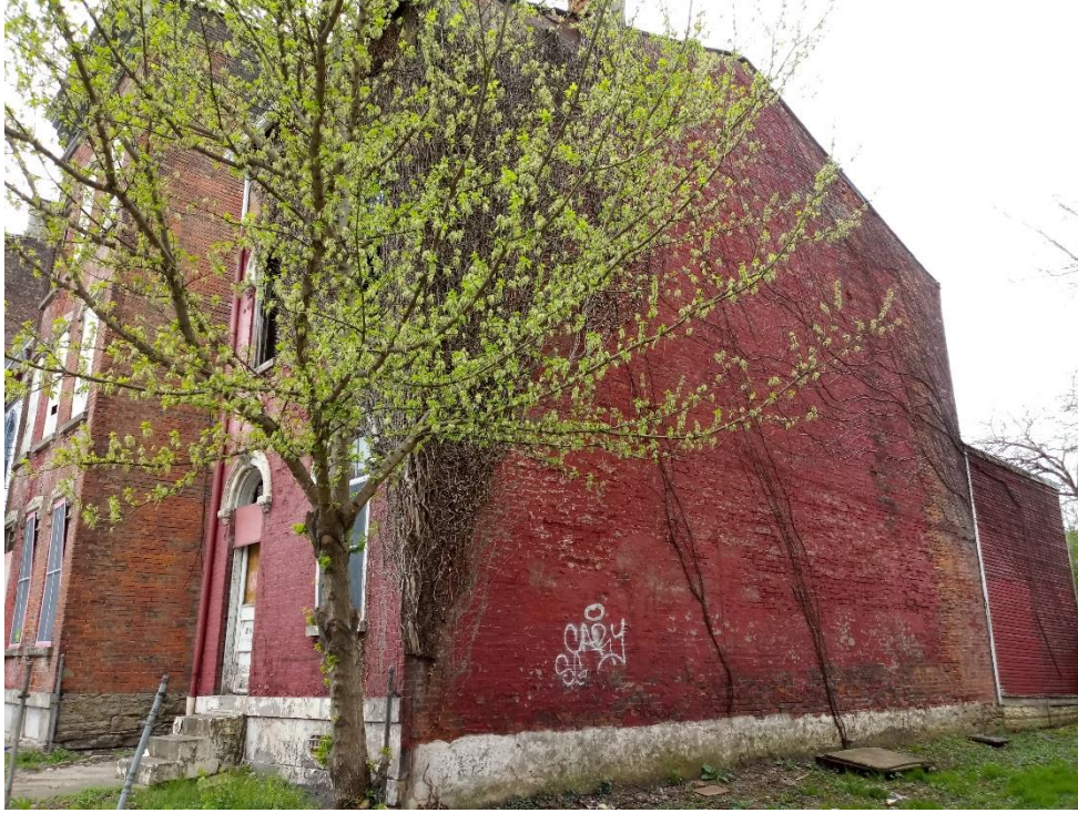
Figure 4 North facing wall showing back addition
