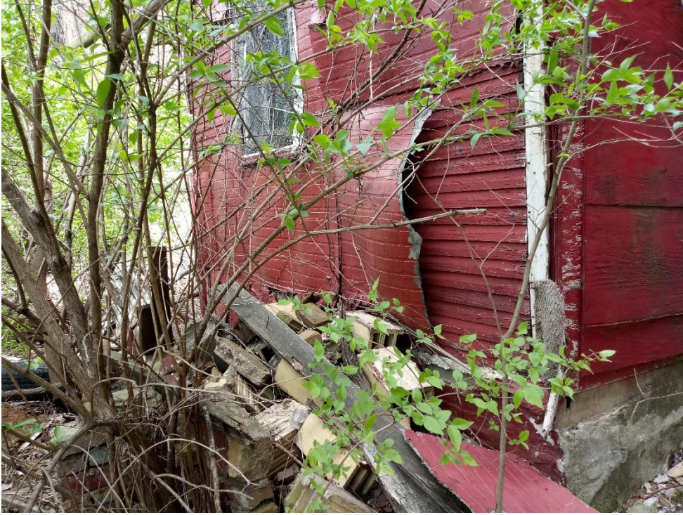
Figure 8 West facing rear of addition
