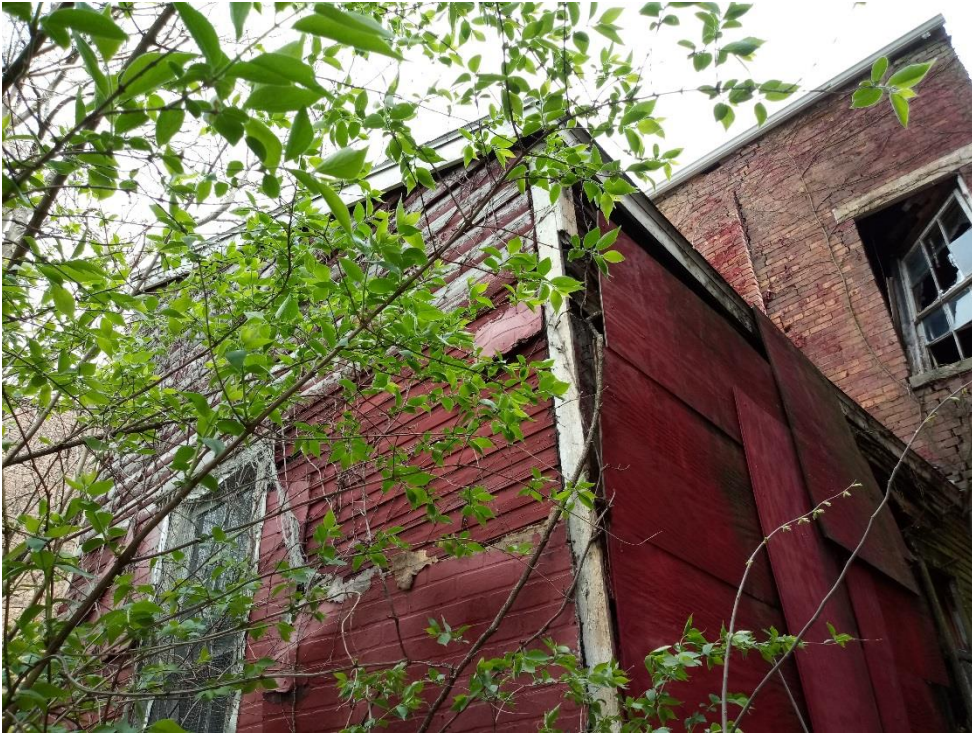
Figure 9 West facing rear of addition
