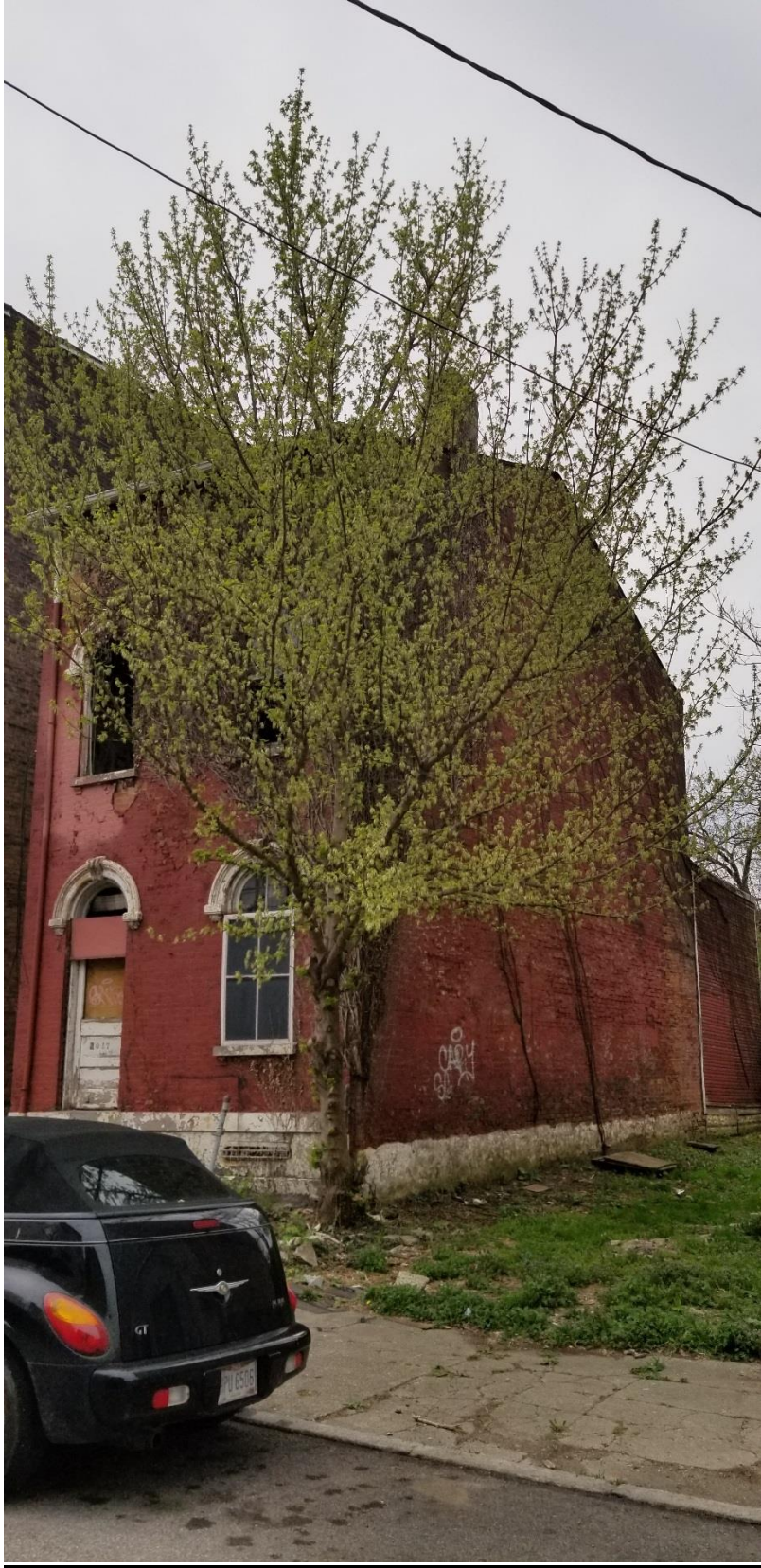
Figure 2 East and North facing walls
