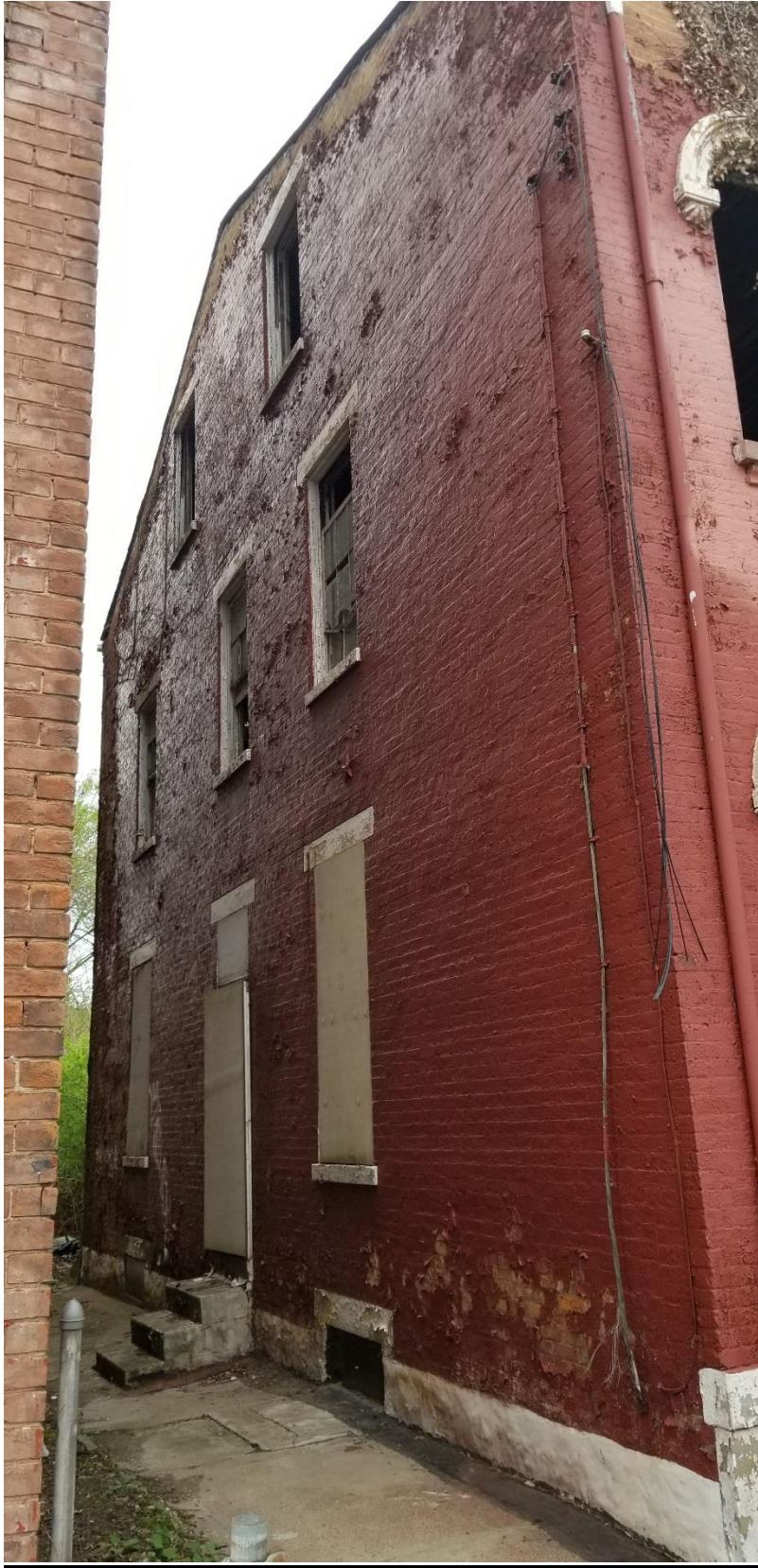
Figure 3 South facing wall, neighboring 2015 Colerain
