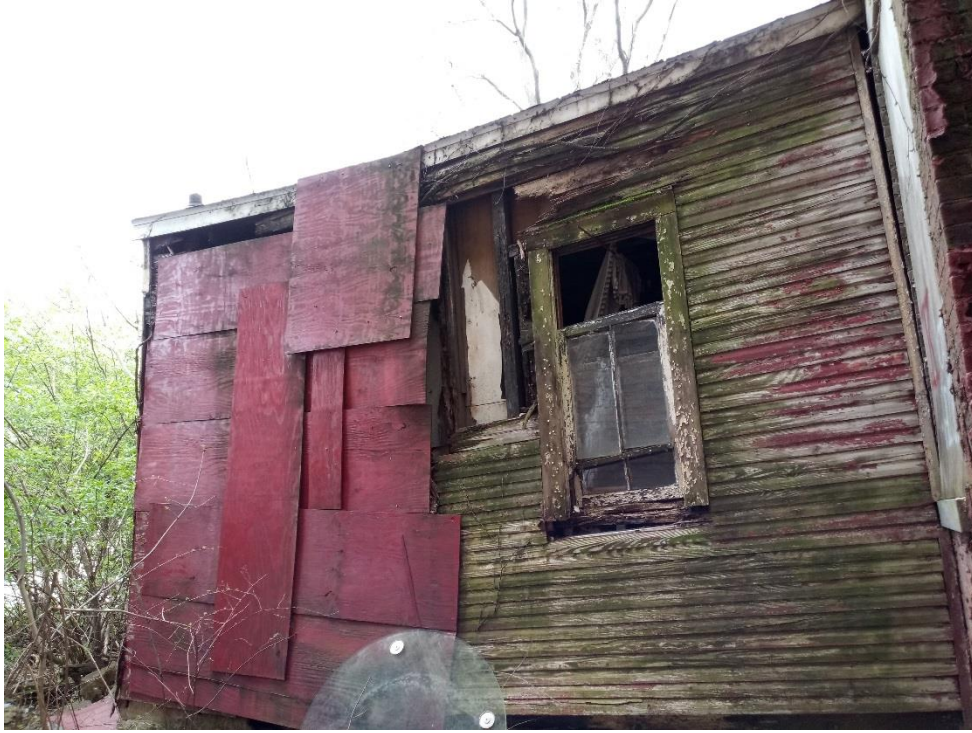
Figure 6 South facing side of rear addition
