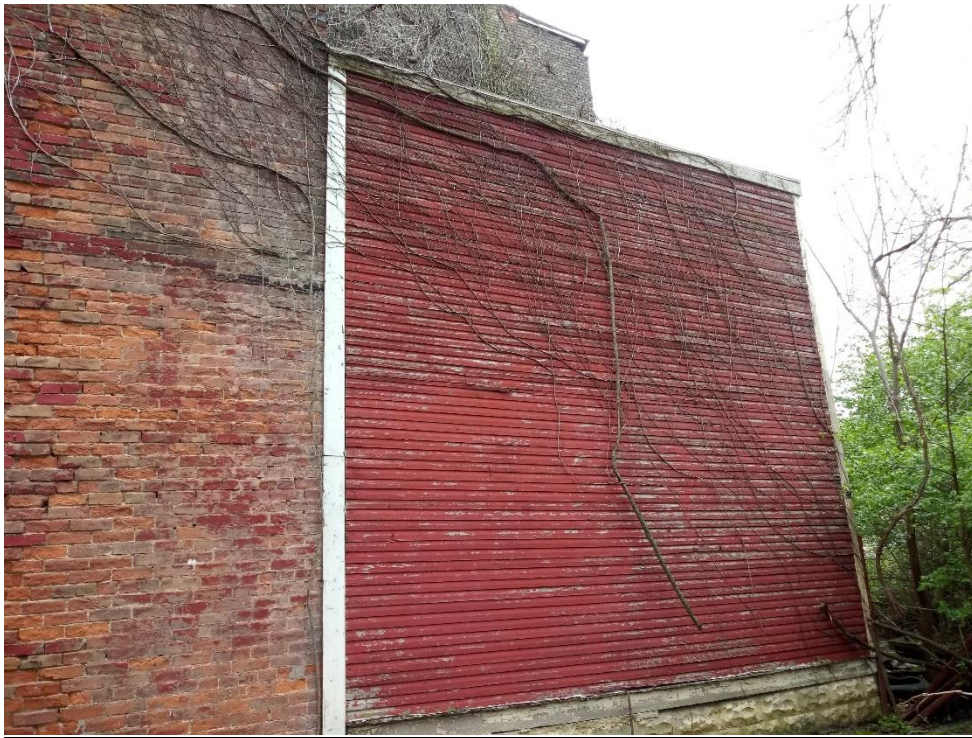
Figure 5 North facing side of rear addition
