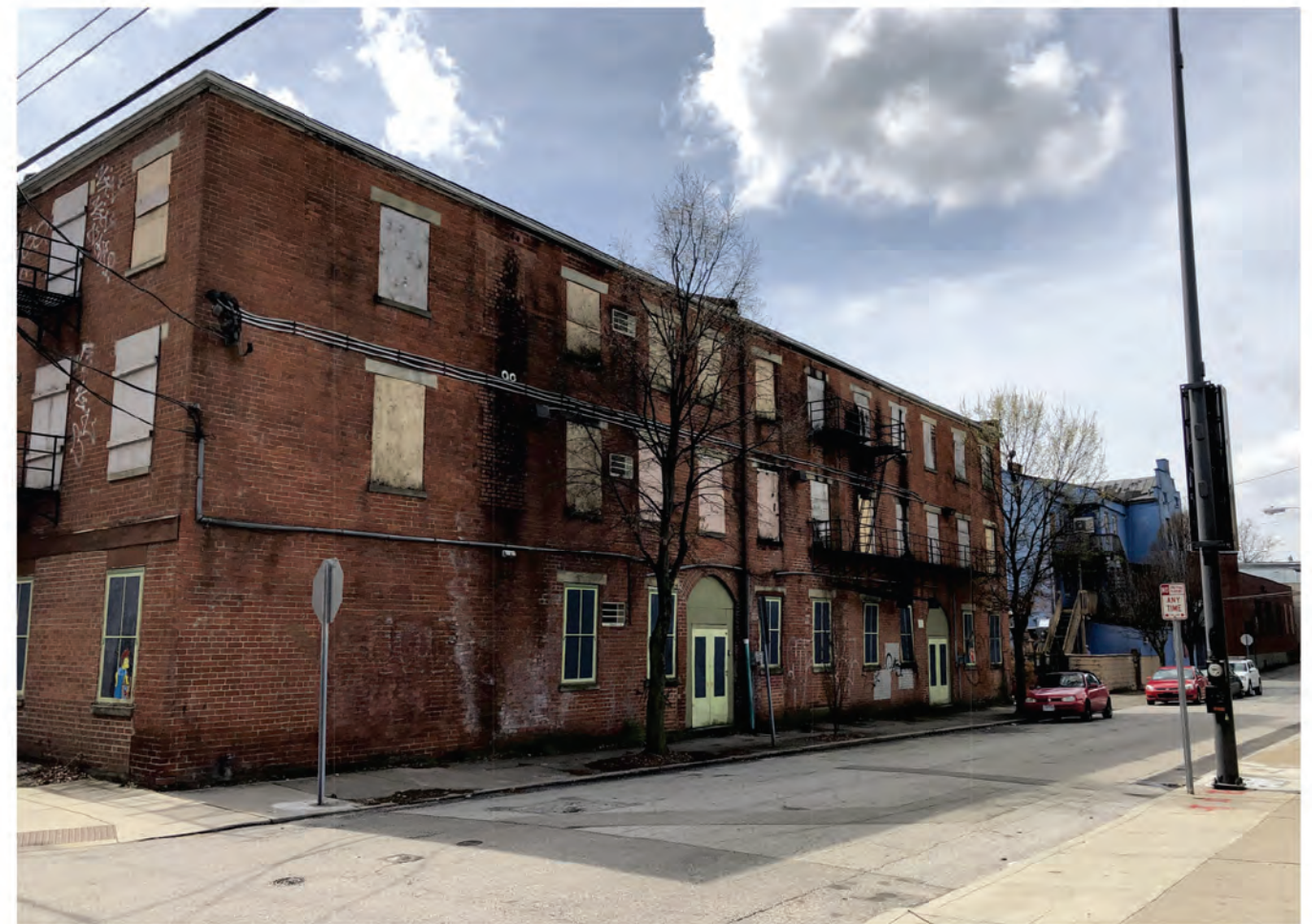
HENRY STREET FACADE
