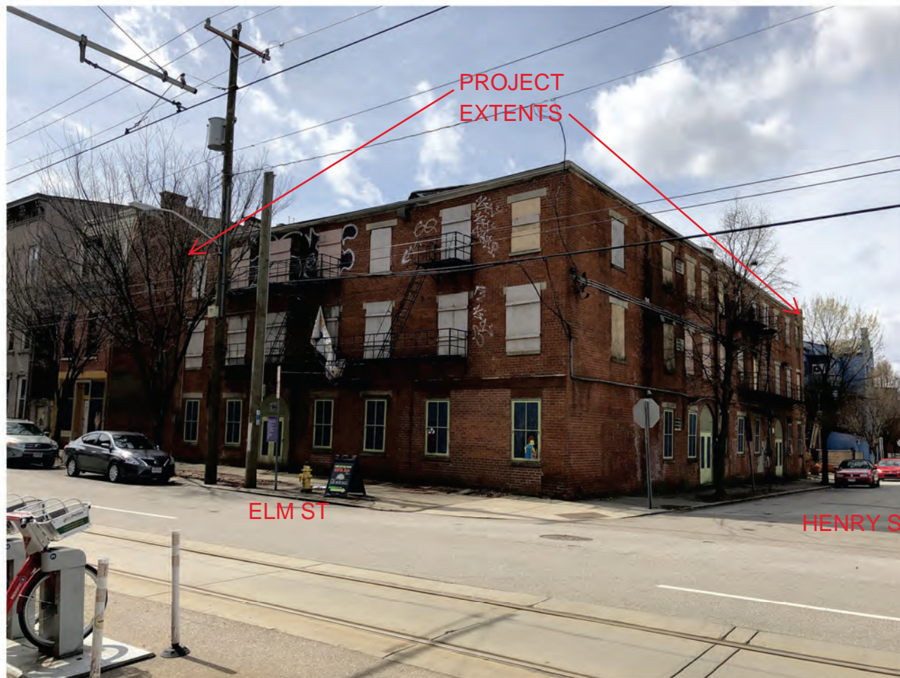
ELM STREET & HENRY STREET FACADES (DEMO NOT VISIBLE)
