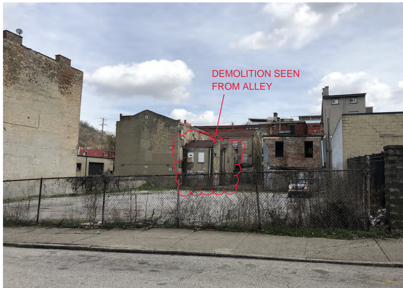
VIEW FROM DUNLAP STREET, ACROSS PARKING LOT & COLBY ALLEY
