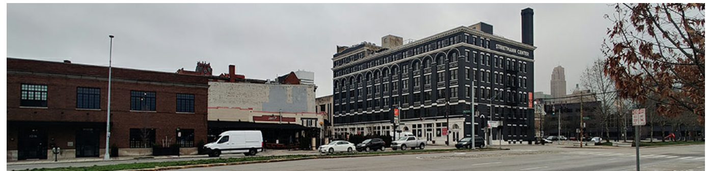
STREETSCAPE - LOOKING SOUTH
