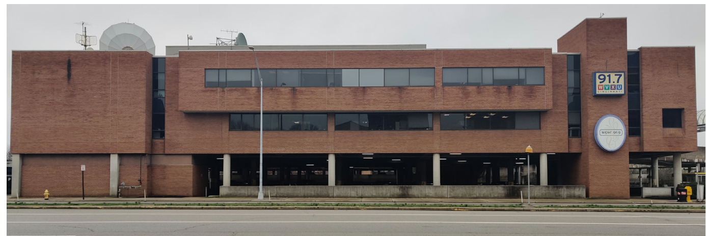
1223 CENTRAL PARKWAY- ACROSS CENTRAL PARKWAY FROM FROM SITE
