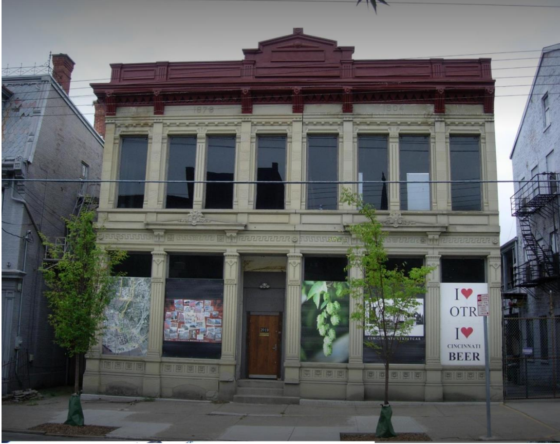
Figure 1: Image of 2019 Elm Street. Image from Google.
