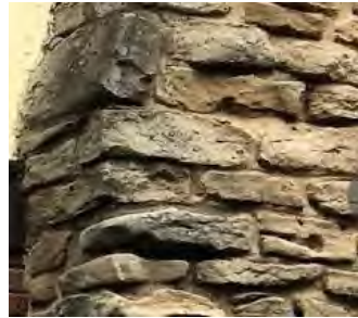
Masonry in fair condition
