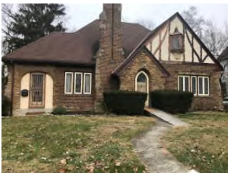
1722 Bella Vista Street March 3, 2019
