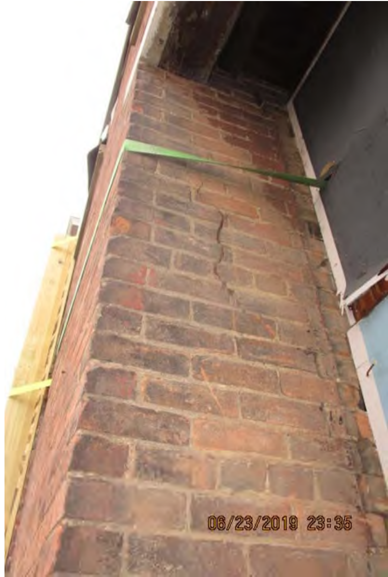
1725 Elm Rear Bldg West Facade
