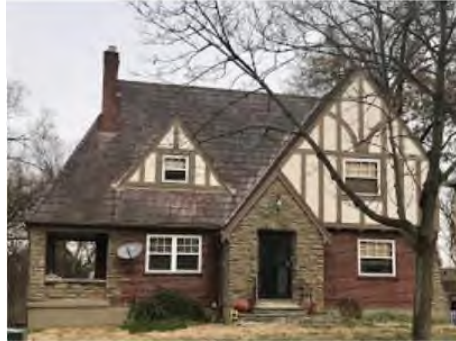
1730 Bella Vista Street March 3, 2019
