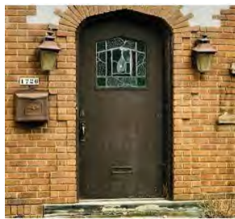
Wood door in fair condition
