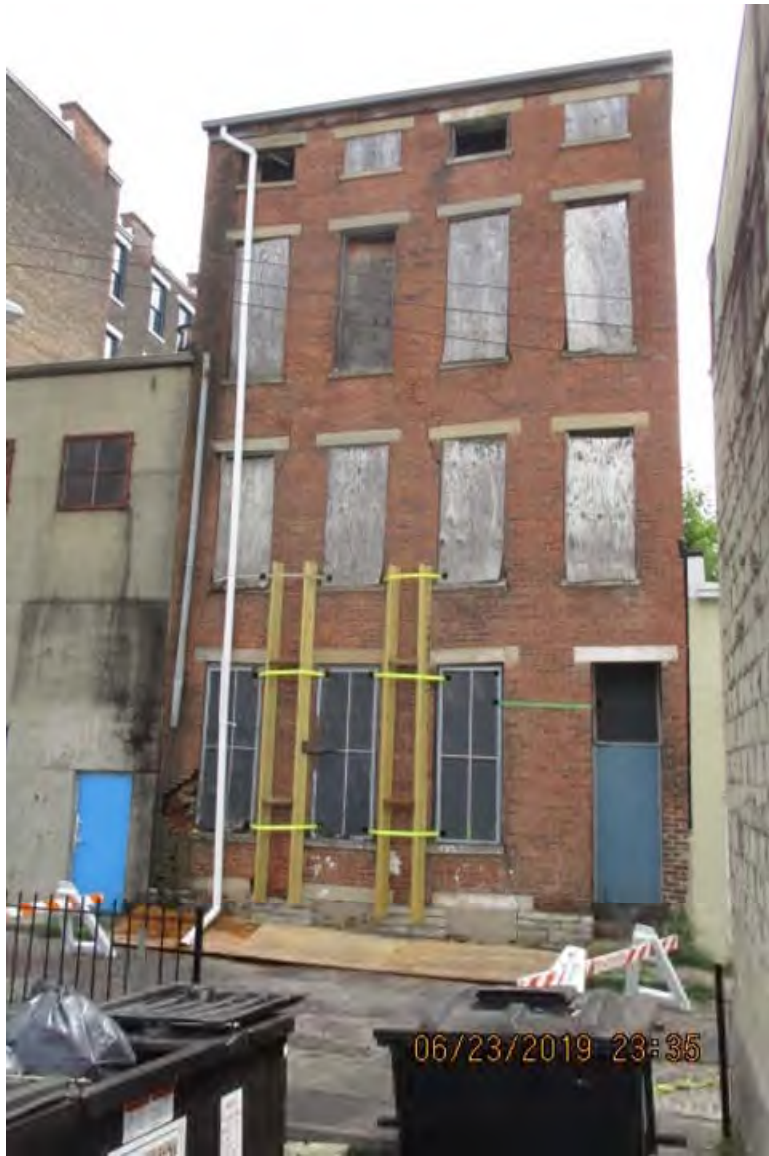
1725 Elm Rear Bldg West Facade
