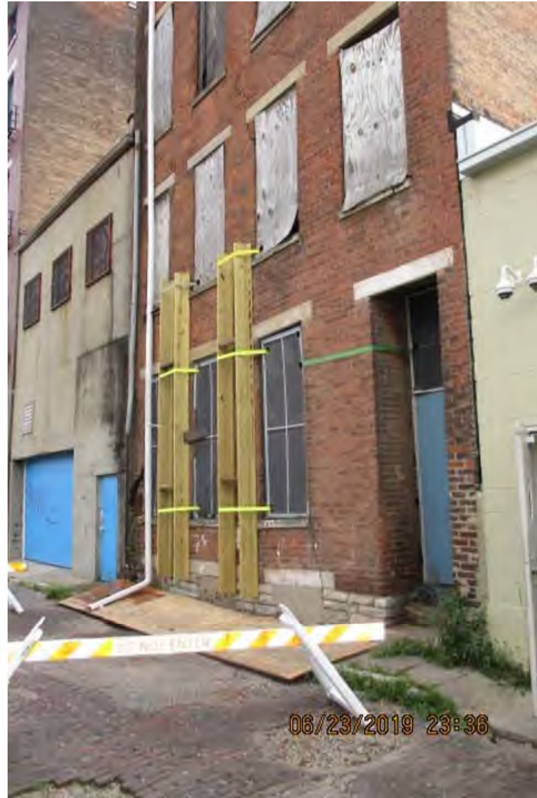
1725 Elm Rear Bldg West Facade
