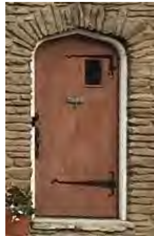
Tudor arch door with original decorative cast iron straps
