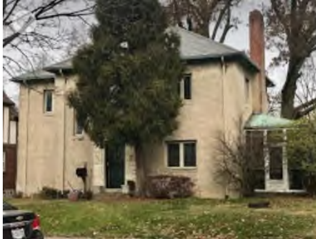
1734 Bella Vista Street March 3, 2019
