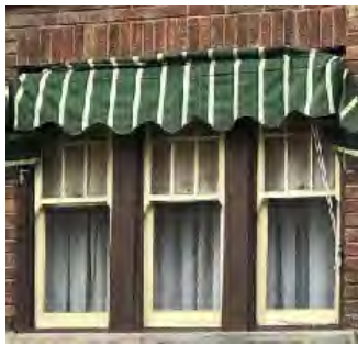
Wood windows in good condition
