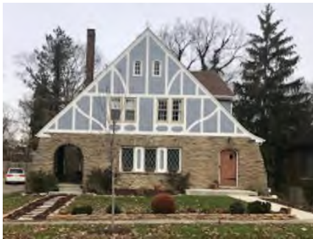
1718 Bella Vista Street March 3, 2019
