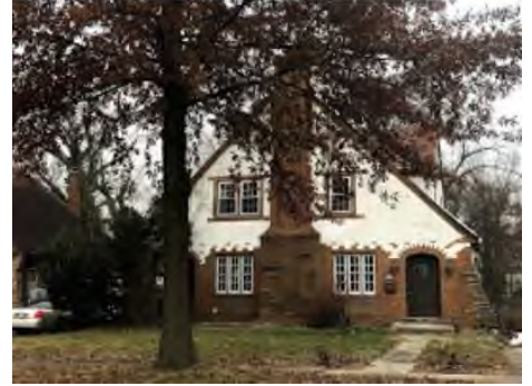
1726 Bella Vista Street March 3, 2019
