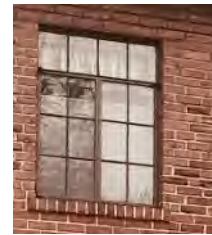
Steel casement windows
