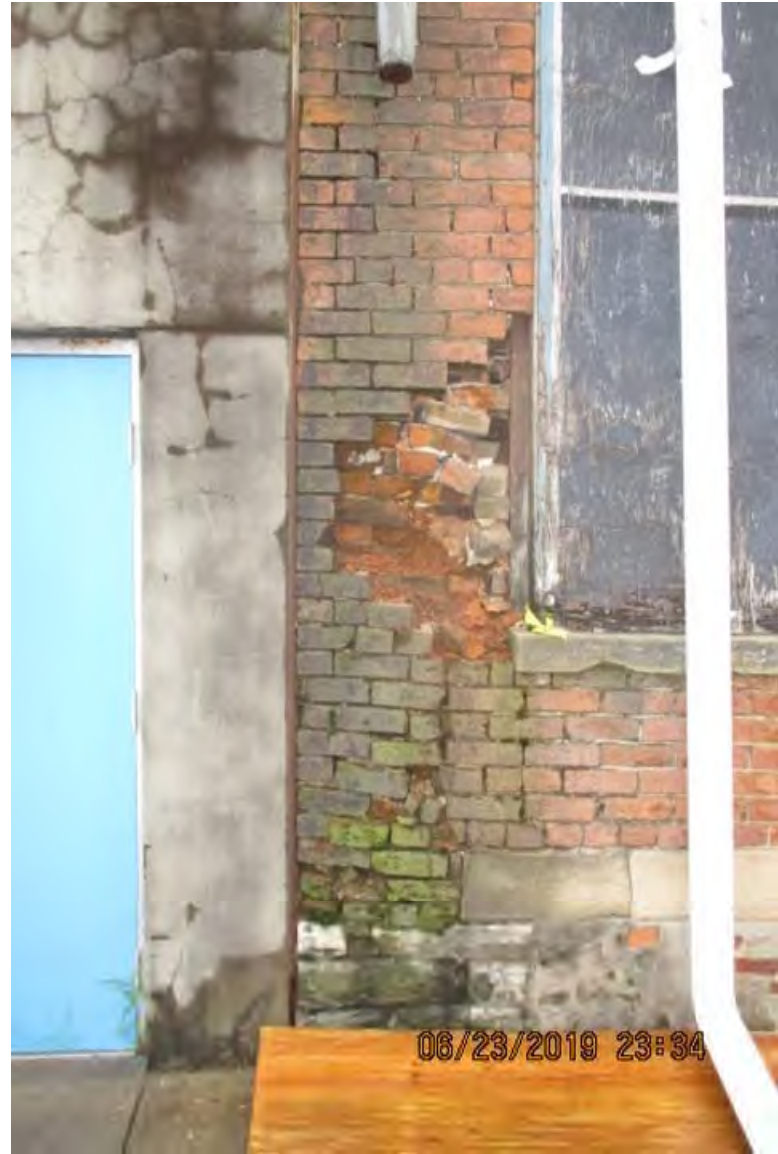
1725 Elm Rear Bldg West Facade
