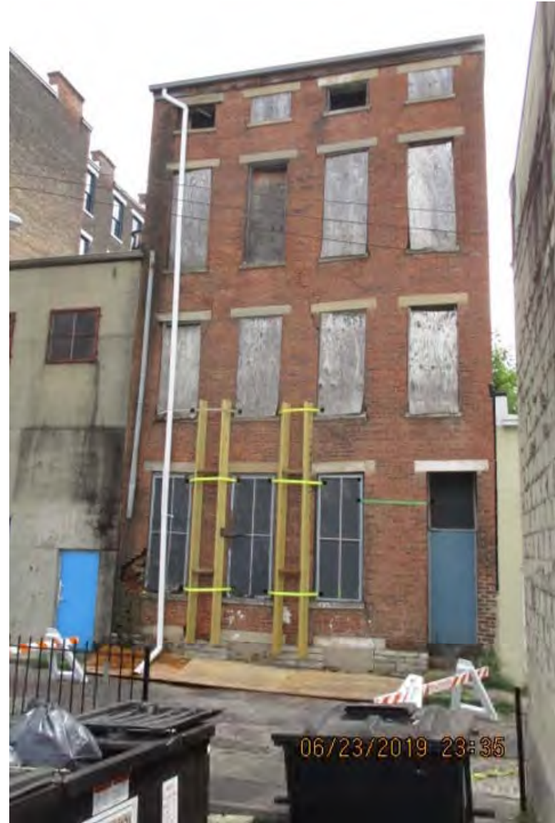
1725 Elm Rear Bldg West Facade
