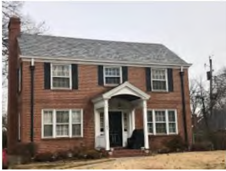
1740 Bella Vista Street, March 3, 2019
