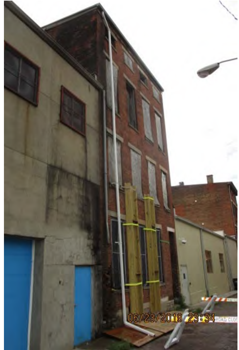
1725 Elm Rear Bldg West Facade
