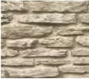
Masonry in good condition
