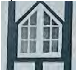
Wood casement windows
