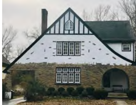
1715 Bella Vista Street March 3, 2019
