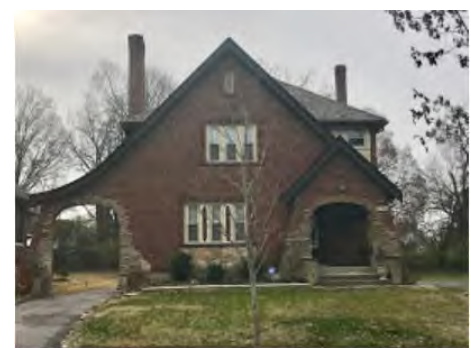
1723 Bella Vista Street March 3, 2019
