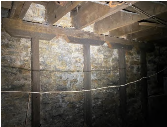
Photo 3 – Existing Floor Shoring, Left Foundation Wall
