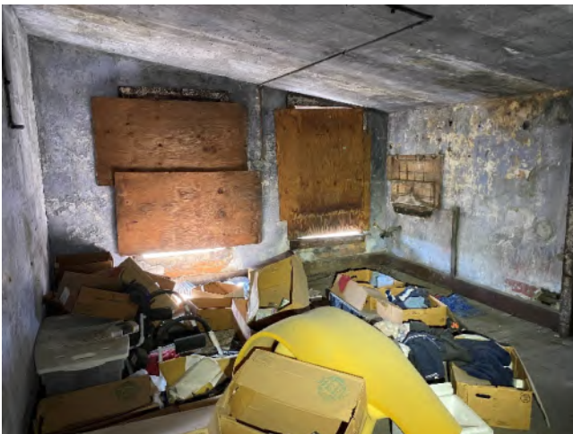
Photo 23 – Typical Attic Space
