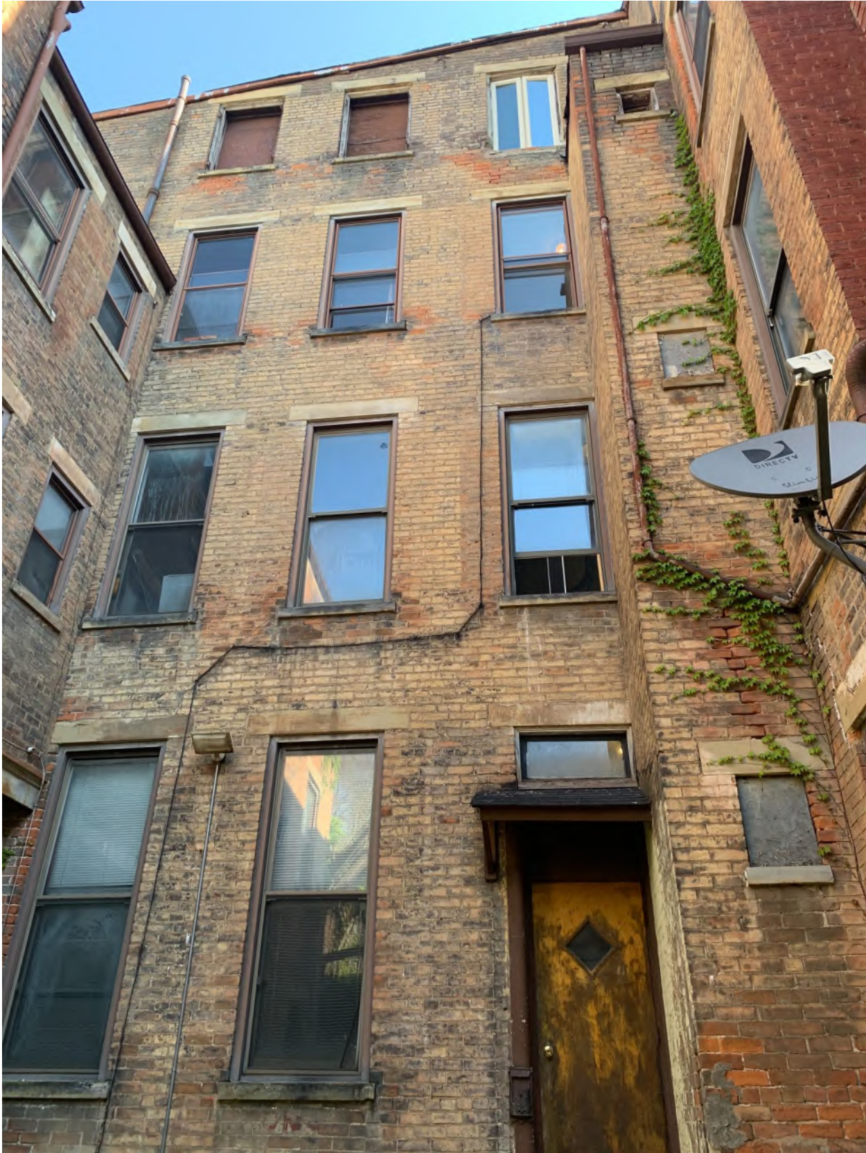
2016 Ohio Ave - South Side
