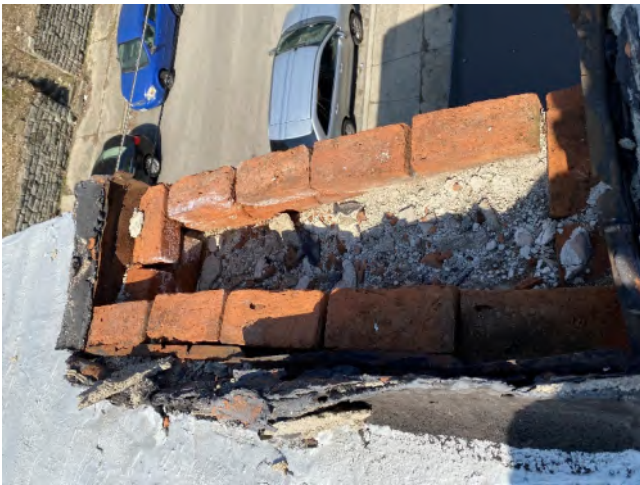
Photo 31 – Exposed Chimney, Demolished Down to Roof Level
