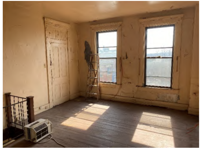
Photo 16 –Third Level, Mid Building
