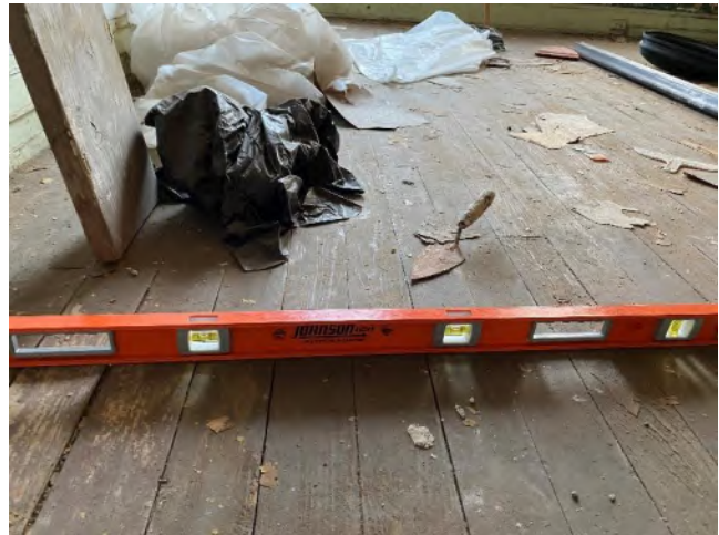
Photo 8 – Typical Floor Levelness Check
