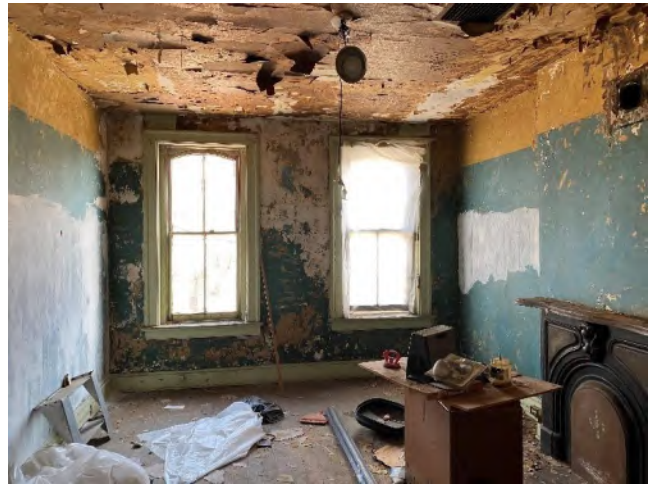
Photo 12 – General Second Floor Level
