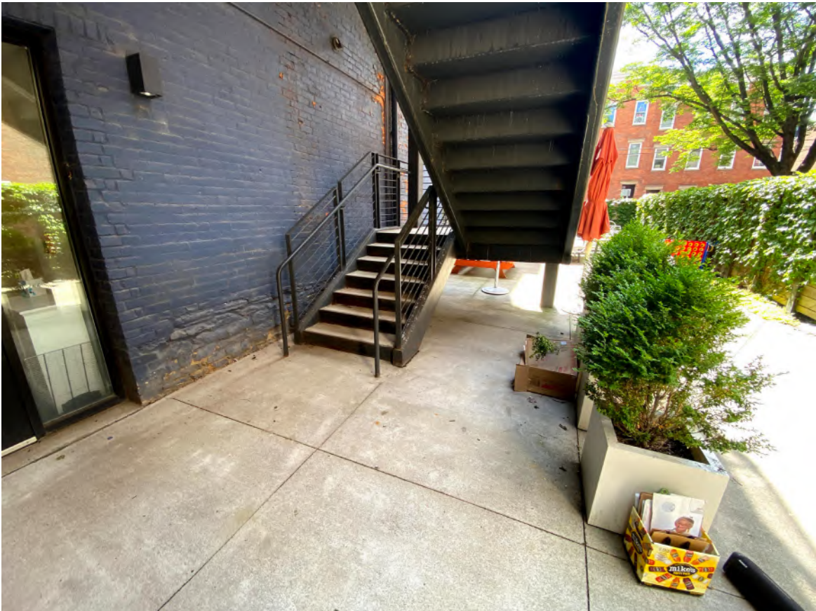
View of patio, beneath existing stair, looking west.
