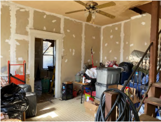
Photo 13 – Second Level, Mid Building
