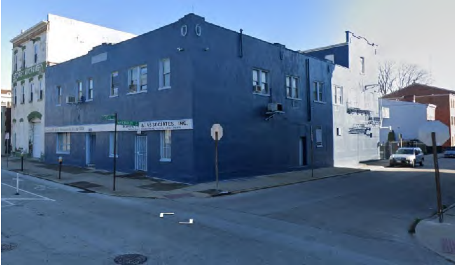
Figure 3: 1416 Central Parkway. Google Street views
