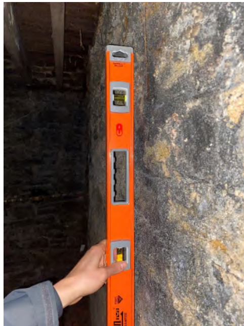
Photo 4 – Typical Foundation Wall Plumbness and Straightness Check
