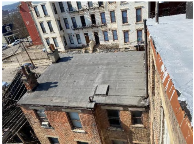
Photo 32 – Roof View from Above
