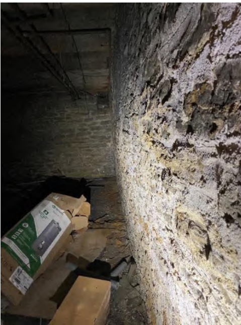
Photo 3 – Typical Perimeter Foundation Wall Condition
