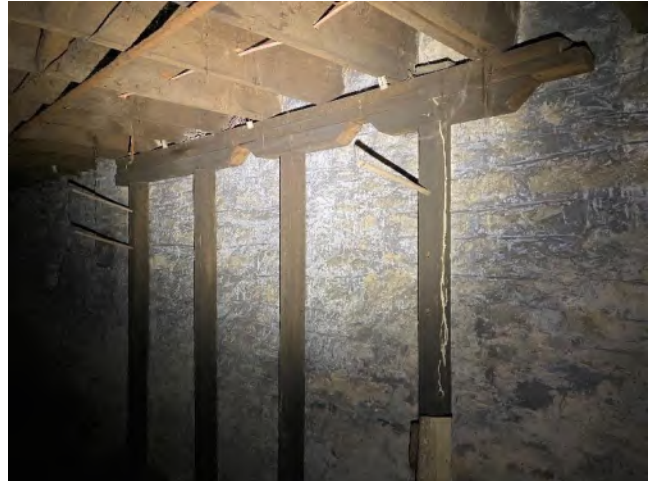
Photo 2 – Existing Floor Shoring, Right Foundation Wall
