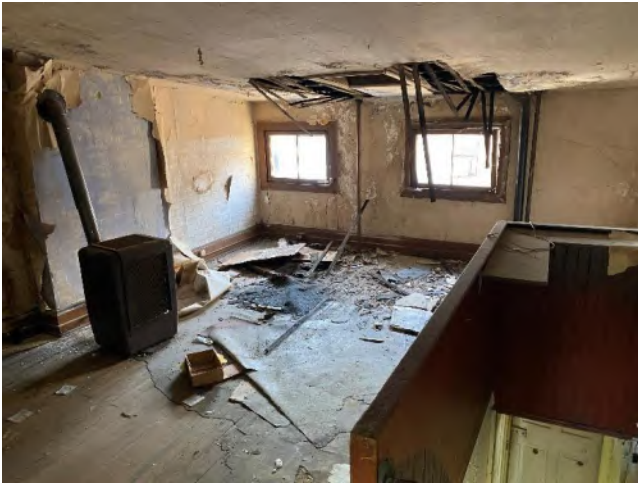
Photo 13 – General Third/Attic Floor Level
