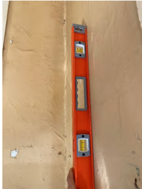
Photo 22 – Typical Wall Plumbness Check
