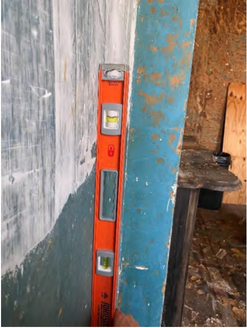
Photo 9 – Typical Wall Plumbness Check
