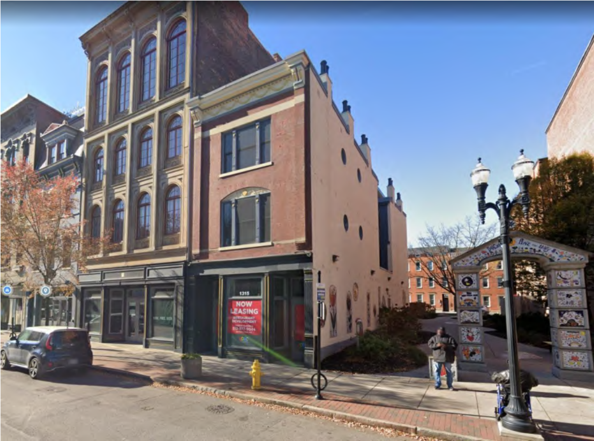
Figure 2. Street view of 1313 Vine Street. Image from Google.
