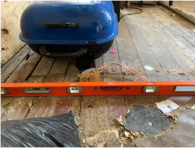
Photo 21 – Typical Floor Levelness Check
