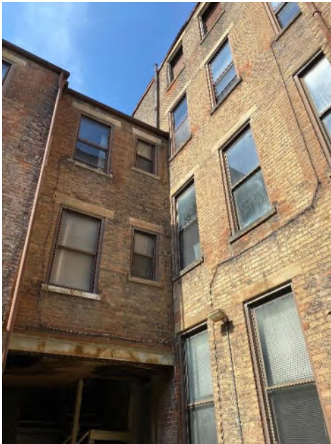
Photo 19 – Rear Exterior Where Building Meets 2016 Ohio Ave
