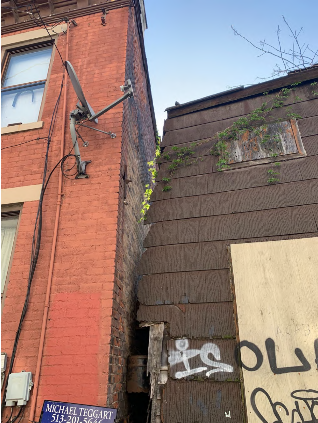
2014 Ohio Ave - South Side
