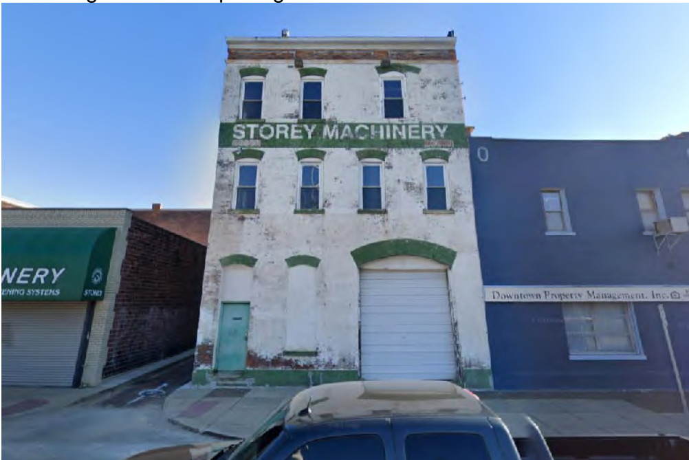
Figure 4: 1420 Central Parkway. Google Street views
