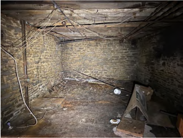
Photo 1 – Right Basement Area
