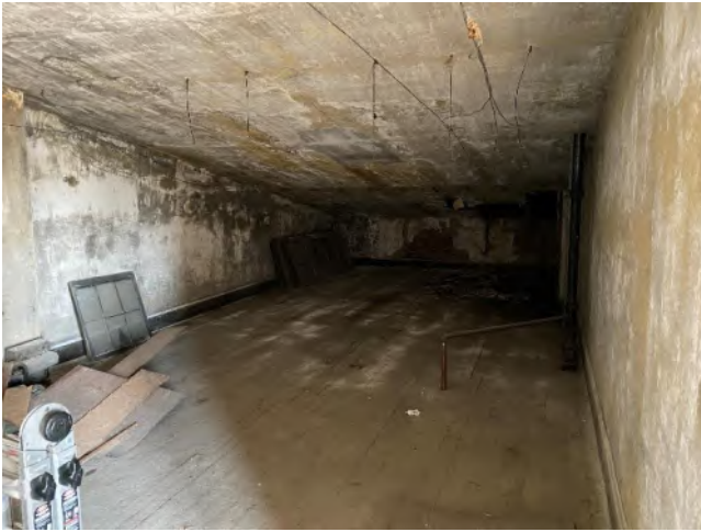
Photo 17 – Attic Space, Front Right
