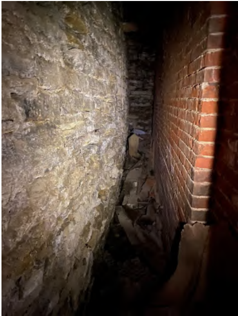
Photo 9 – Front Retaining Wall Below Street Level
