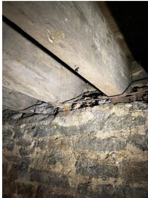
Photo 8 – Typical Joist Bearing, Right Foundation Wall
