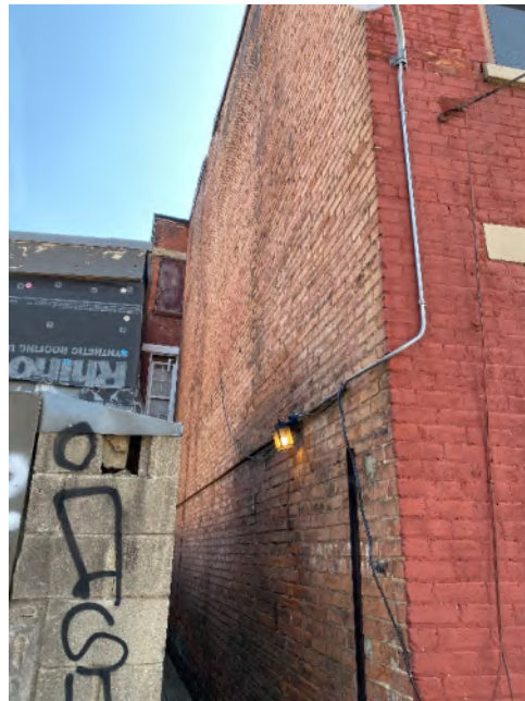
Photo 31 – Left Exterior Building
