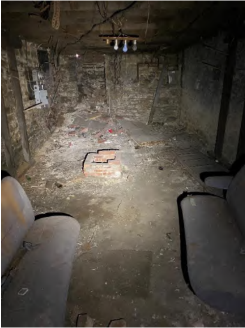
Photo 1 – General Basement Area
