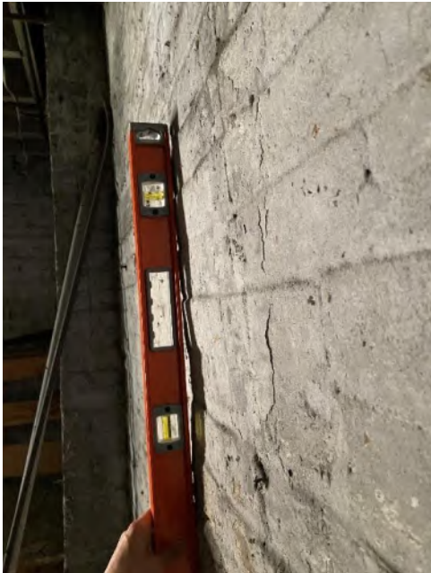
Photo 3 – Wall Plumbness Check, Basement
