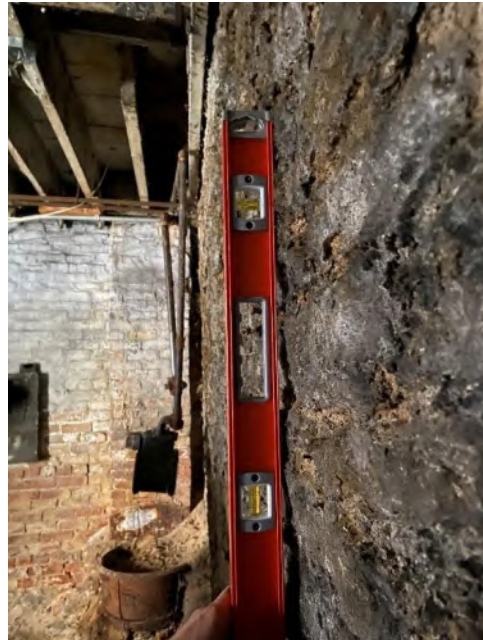
Photo 4 – Wall Plumbness Check, Basement
