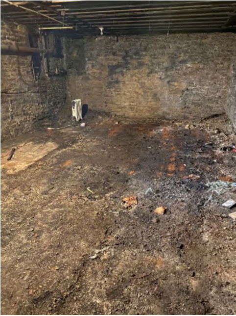
Photo 1 – Basement Area, Earthen Floor
