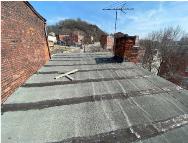
Photo 15 – General Roof and Built-Up Membrane
