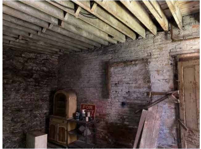
Photo 2 – Basement Area Looking Towards Left Wall
