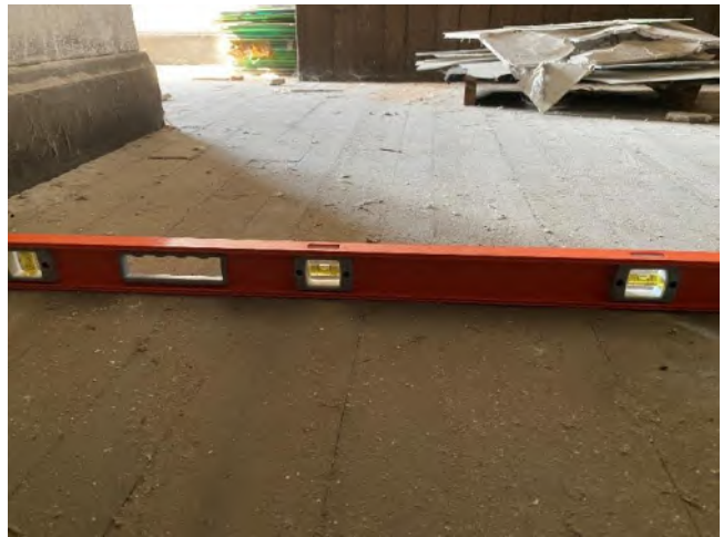
Photo 16 – Floor Levelness Check
