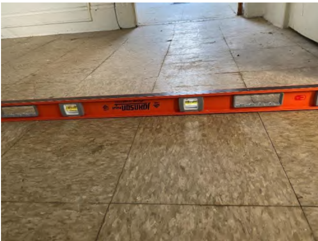
Photo 31 – Typical Floor Levelness Check
