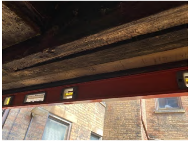
Photo 14 – Floor Beam Sag Check
