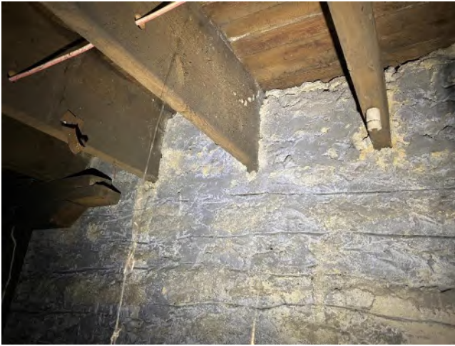
Photo 5 – First Floor Joist Bearing Ends at Left Foundation
