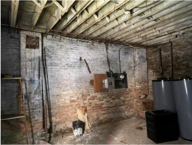
Photo 1 – Basement Area Looking Towards Right Wall
