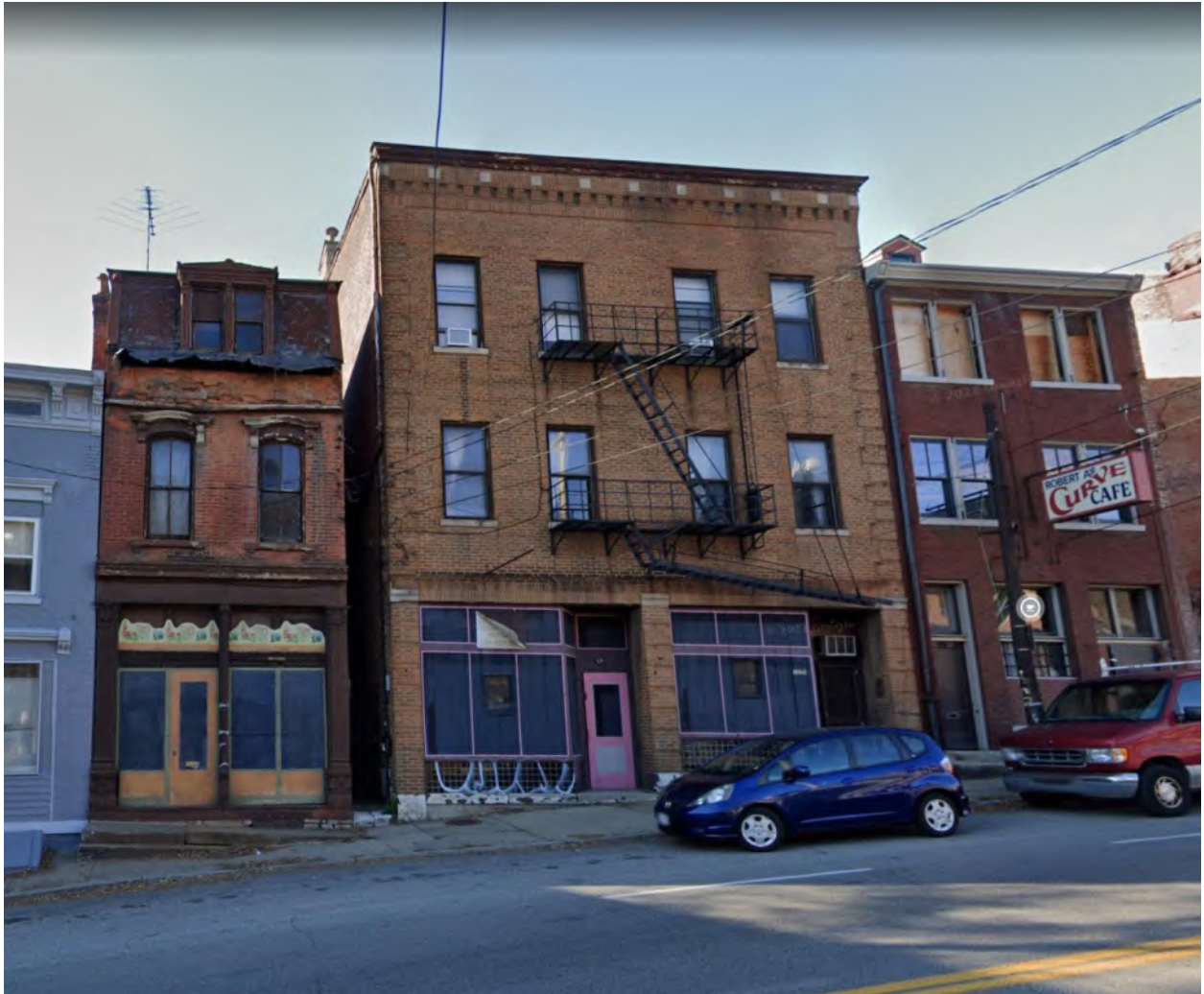
Figure 3. Street view of 2025-2029 Vine Street. Image from Google.
