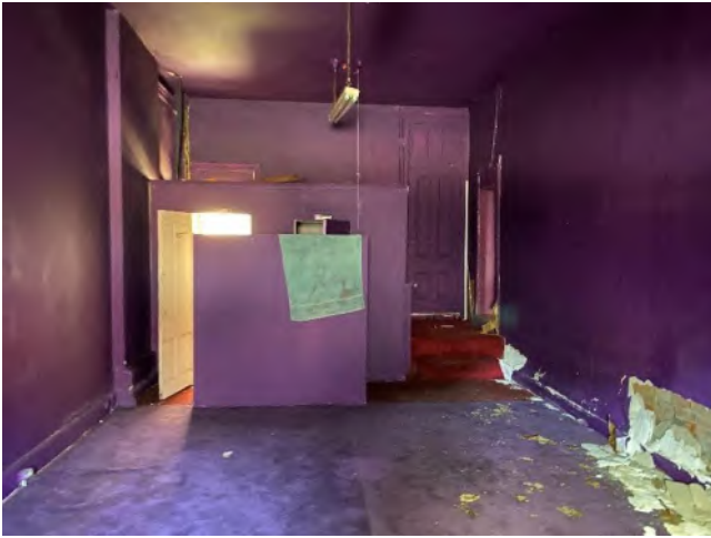
Photo 13 – Abandoned Church, Left First Level
