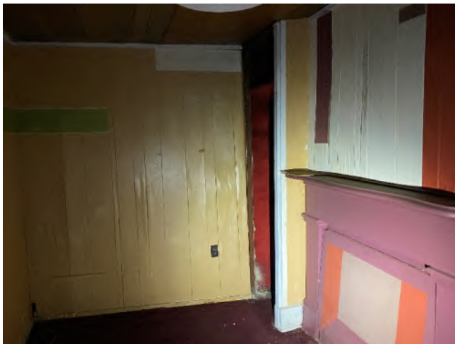
Photo 11 – First-Level, Front Building
