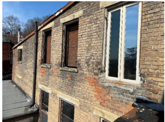
Photo 28 – Right Exterior Building
