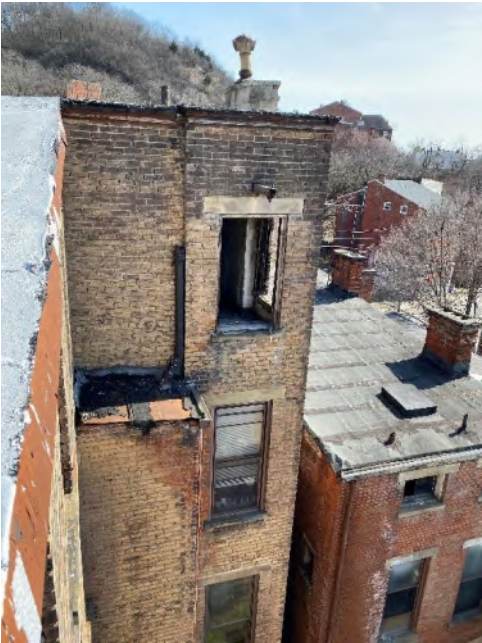
Photo 25 – Brick Exterior, Rear Face of Building
