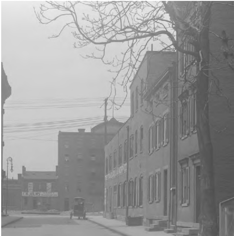
Figure 8: 1921 Picture of the south façade of 1416 Central Parkway
