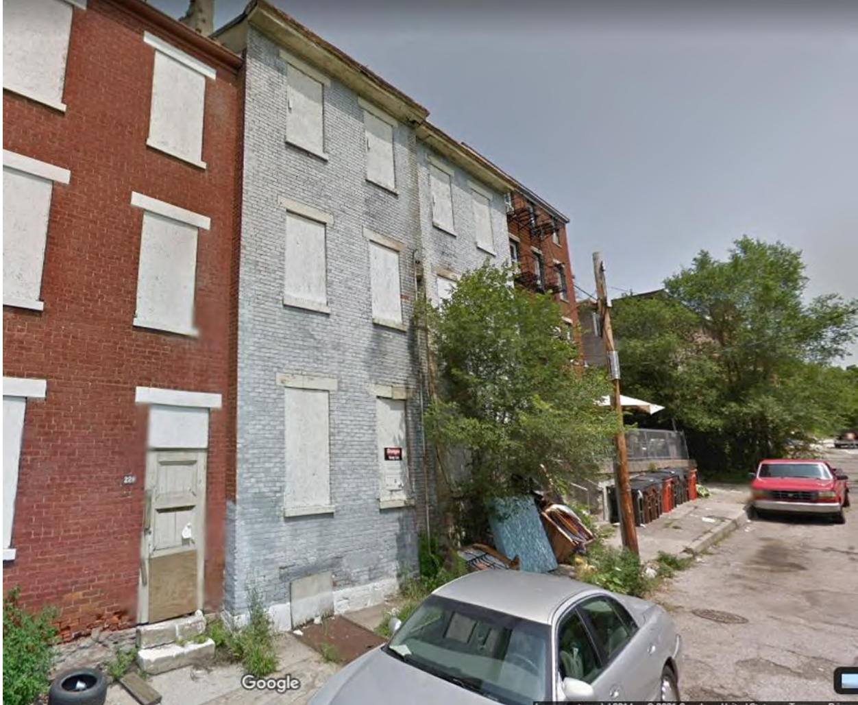
Figure 2. Street view of 222 Mohawk Street. Image from Google.
