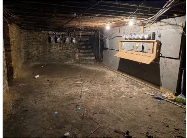
Photo 2 – Left Basement Area
