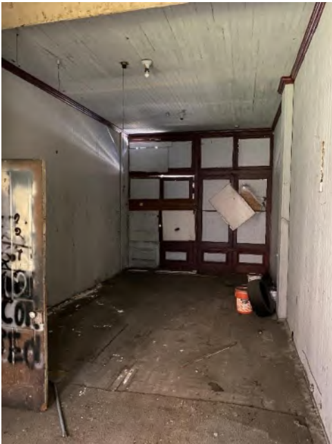
Photo 7 – First Floor Level
