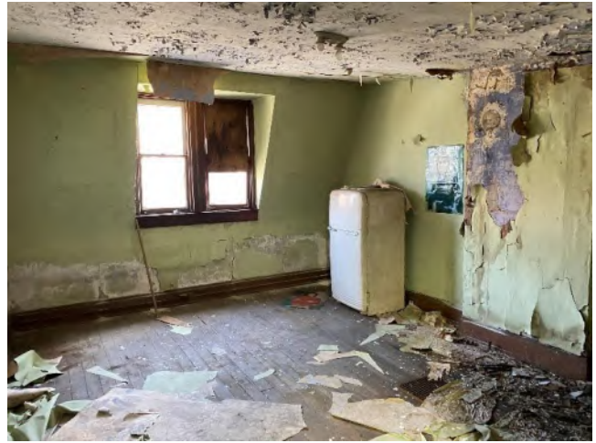
Photo 14 – General Third/Attic Floor Level
