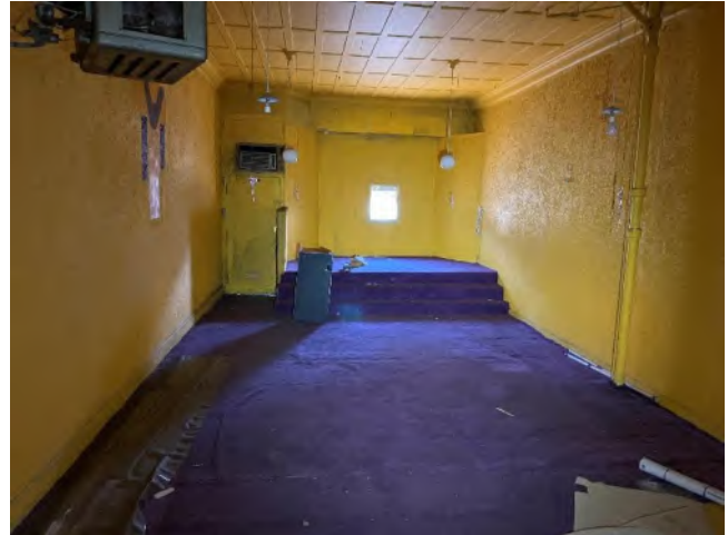
Photo 12 – Abandoned Church, Right First Level
