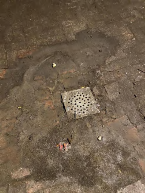
Photo 11 – Basement Floor Drain
