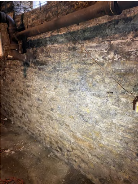
Photo 3 – Typical Grouted Fieldstone Foundation Wall
