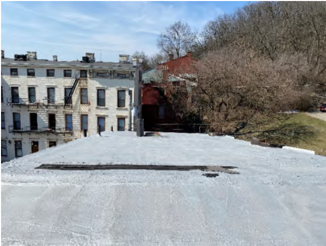
Photo 29 – General Roof and Membrane
