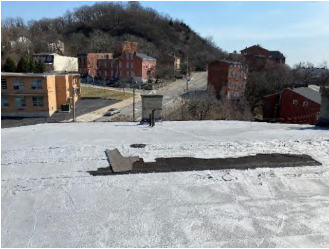
Photo 21 – General Roof and Condition
