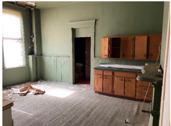
Photo 12 – First-Level, Mid Building
