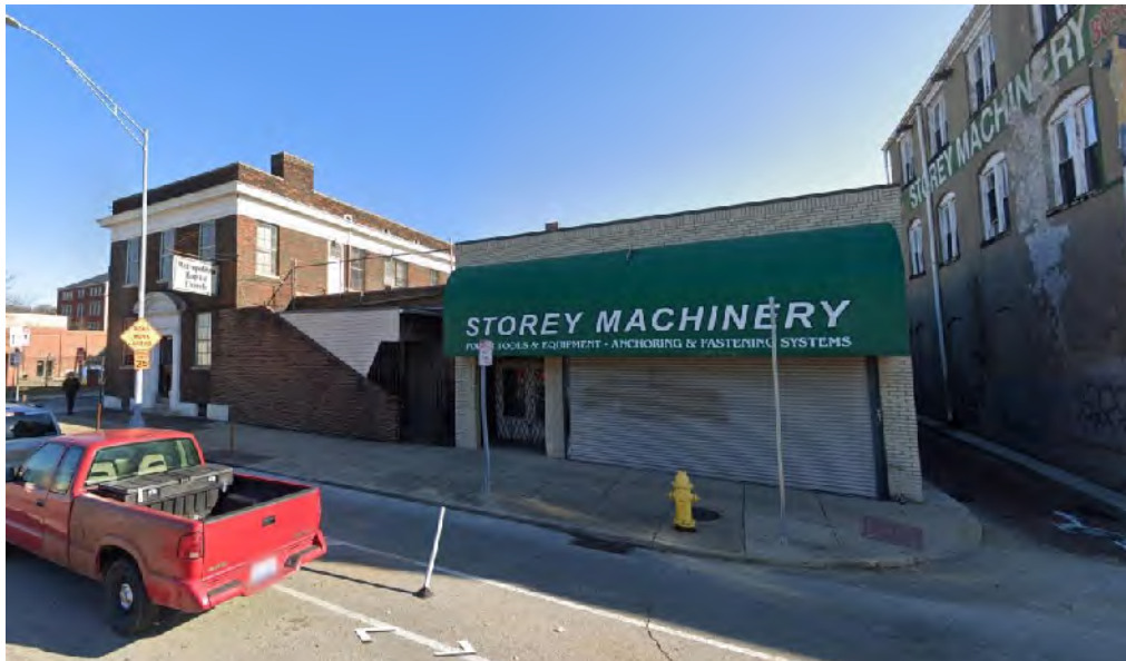
Figure 5: 1424-1430 Central Parkway. Google Street views
