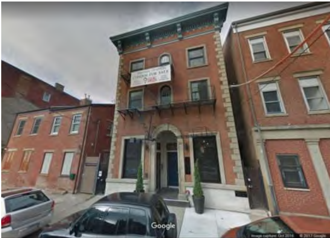
Figure 2. View of 1523 Republic Street. Image courtesy of Google.
