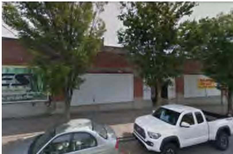
Figure 2: Front facade of existing 2014 Elm Street
