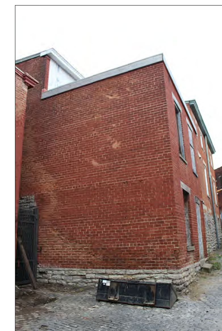
1921 VINE REAR/ SIDE FACADE
