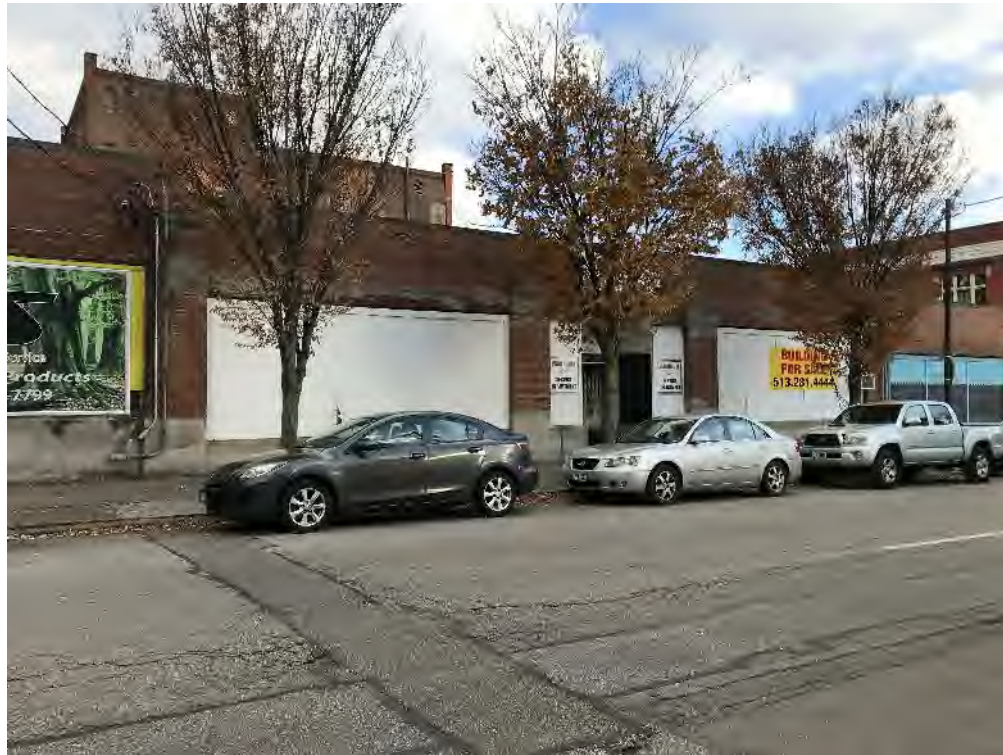
1. FRONT VIEW - NW
