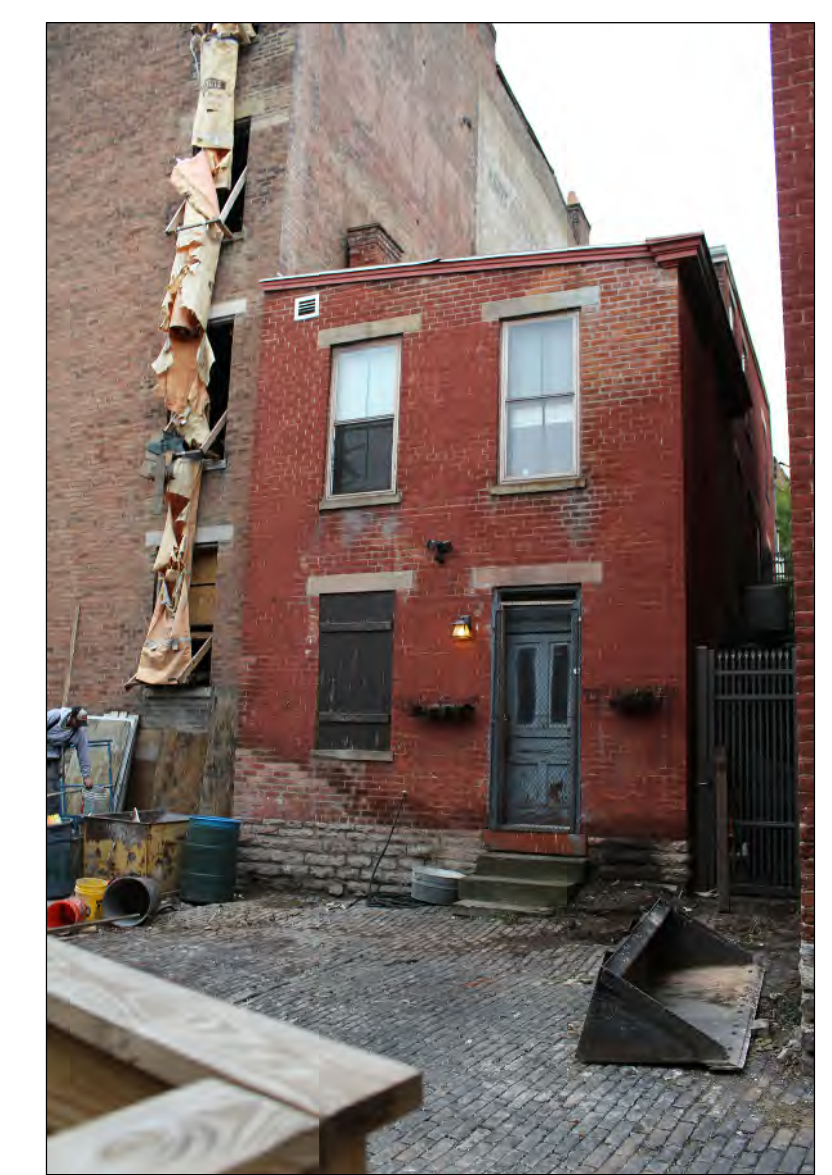
1923 VINE REAR/ SIDE FACADE
