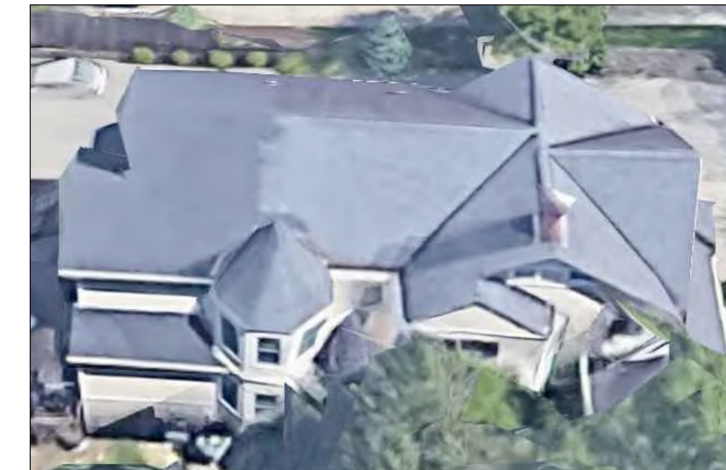
VIEW OF SOUTH FACADE AND ROOF
