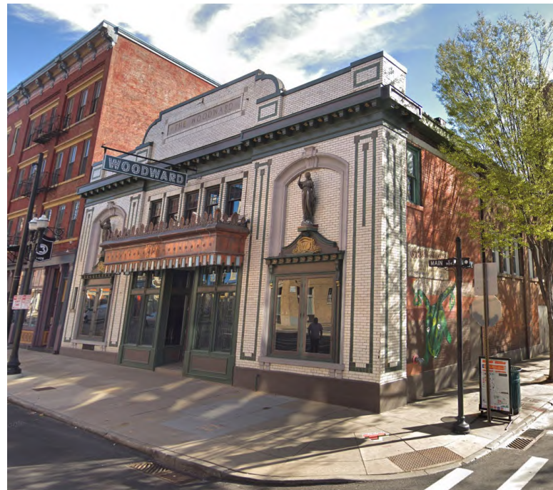
Woodward Theatre: 1.5 story at corner of 14th and Main
