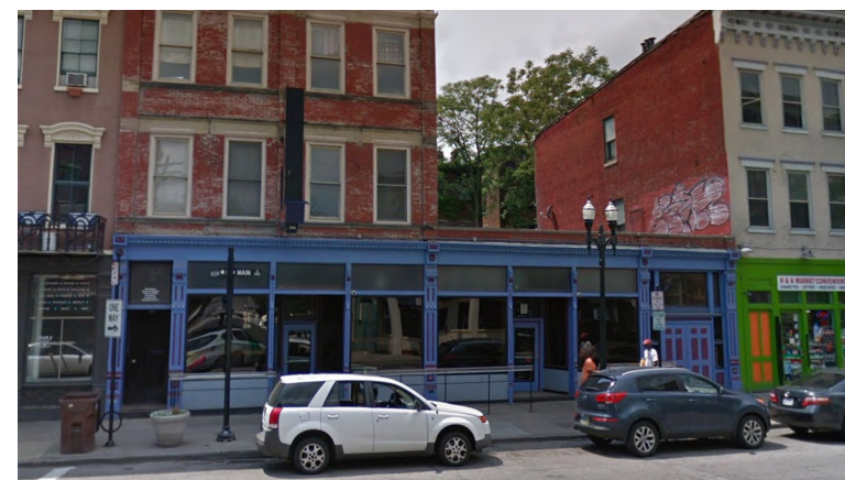
Mr. Pitiful's: 1 story mid-block building at Main St.
