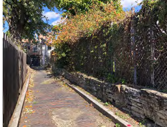
E. Retaining wall.
