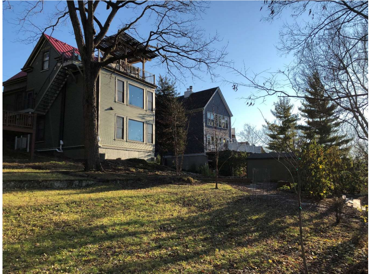
Rear of house. Existing shed at lower right. The highest point of the new shed will be approximately the same height as the deck beyond (with the white railing).
