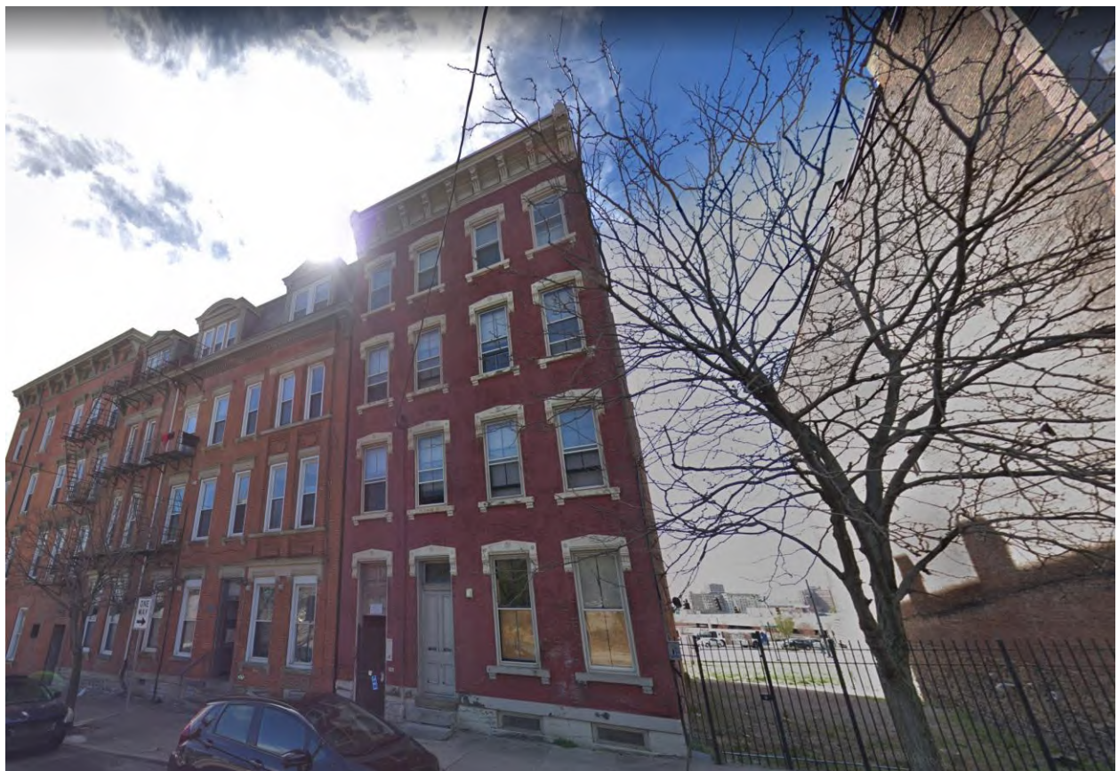
Figure 2. Street view of 555 E 13 th Street. Image from Google.
