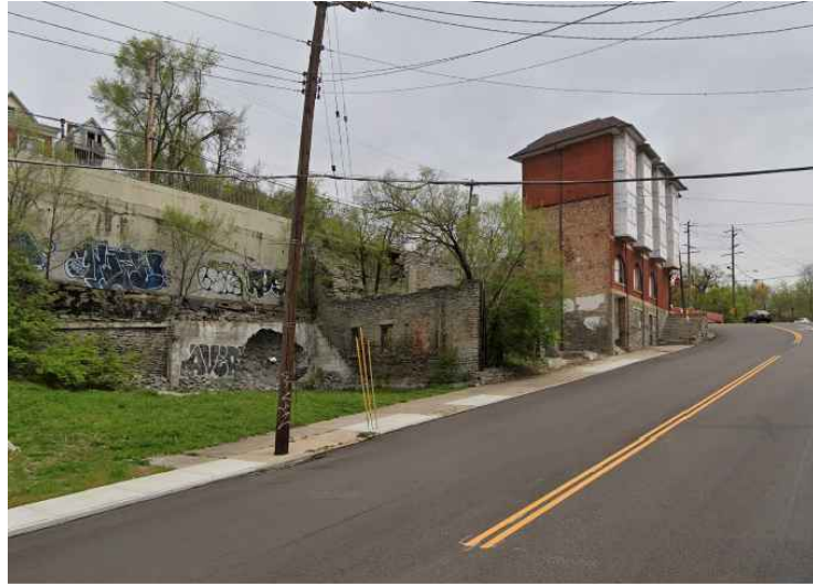
VIEW UP SYCAMORE STREET
