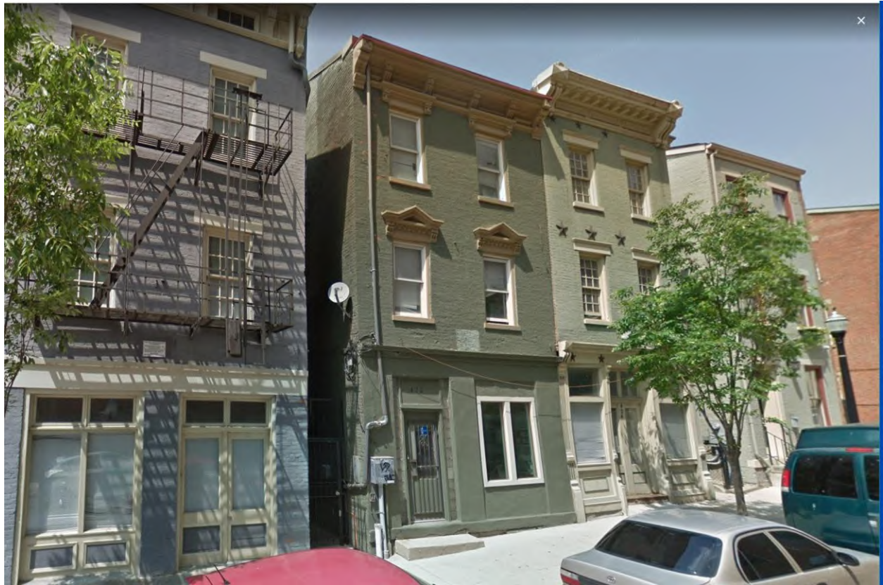
Figure 2. Street view of 422 E 12th Street. Image from Google.
