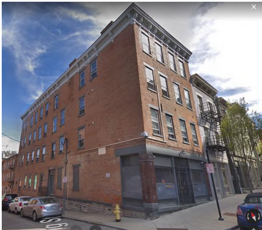
Figure 2. Street view of 418 E 12th Street. Image from Google.
