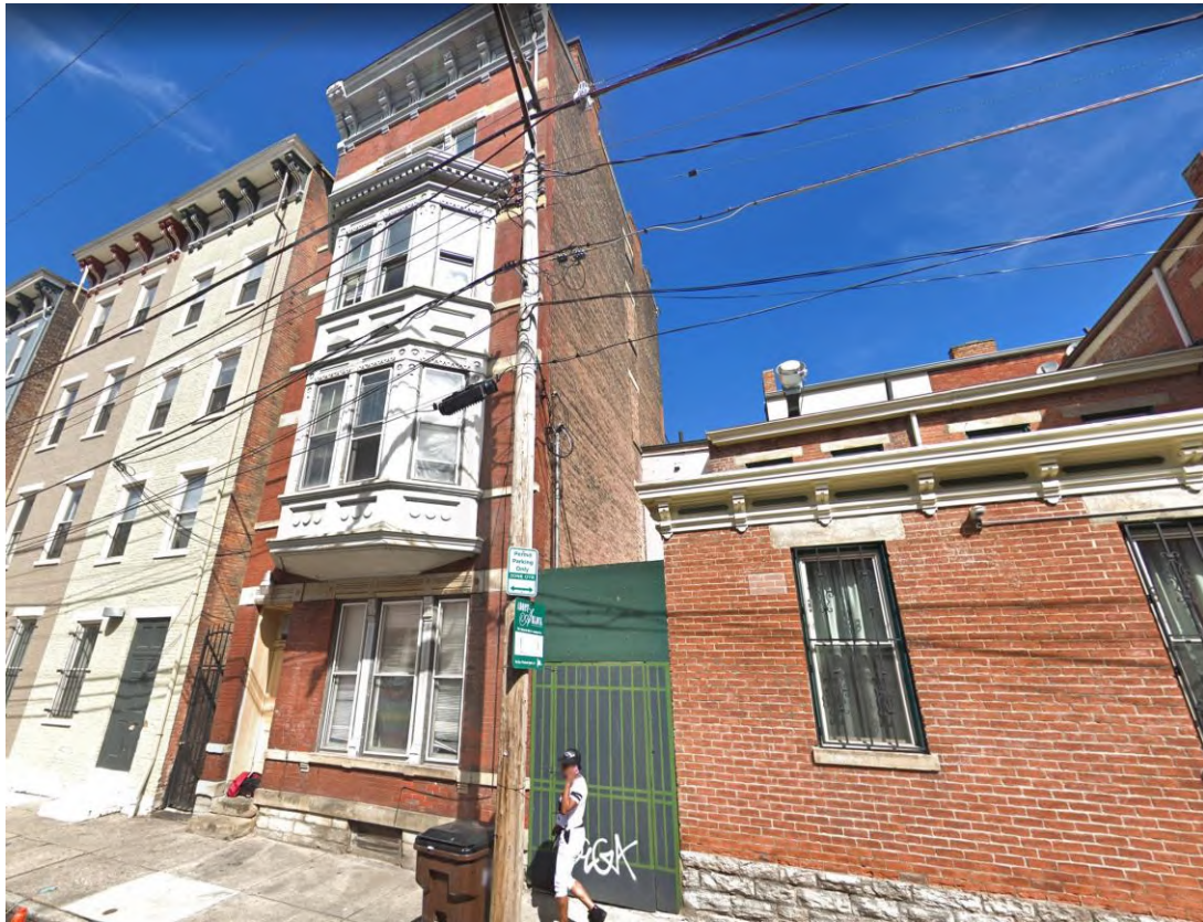
Figure 2. Street view of 30 E 15 th Street. Image from Google.
