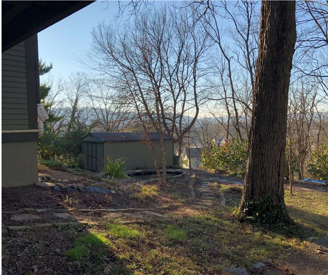
View of existing shed from north, looking south. Front and back of proposed covered parking structure will approximately align with the front and rear of this existing structure. Rear deck will sit beyond.
