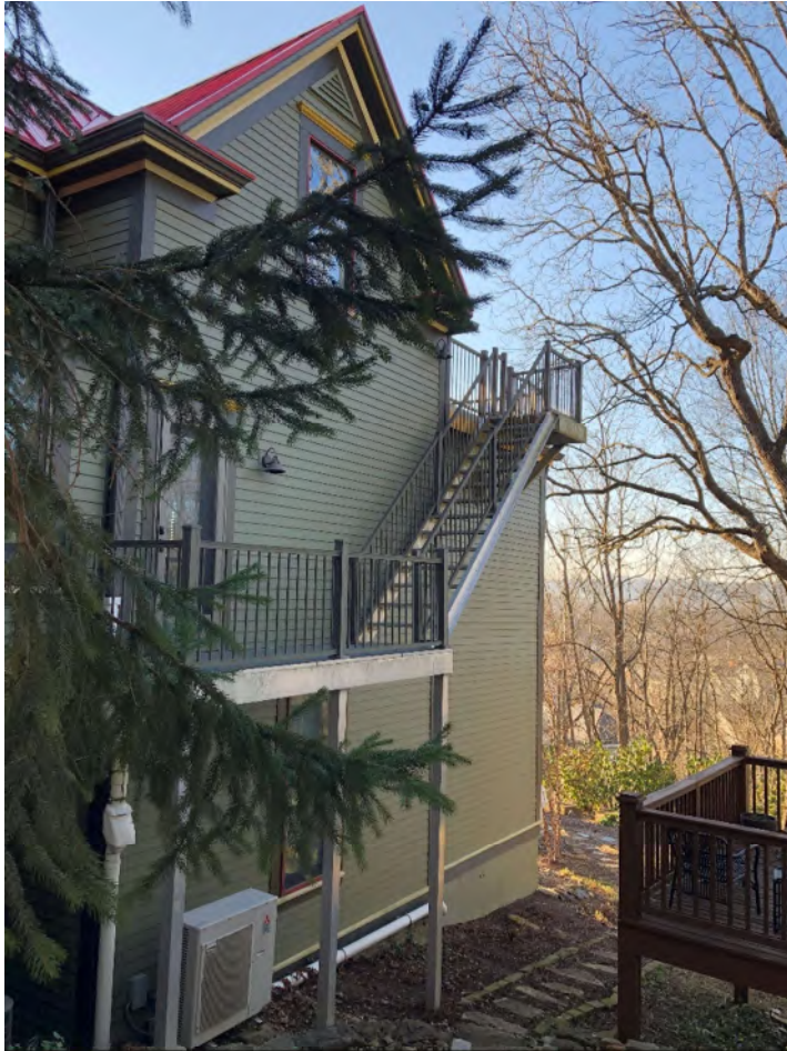
Existing aluminum structure at residence. Similar look proposed for shed posts.
