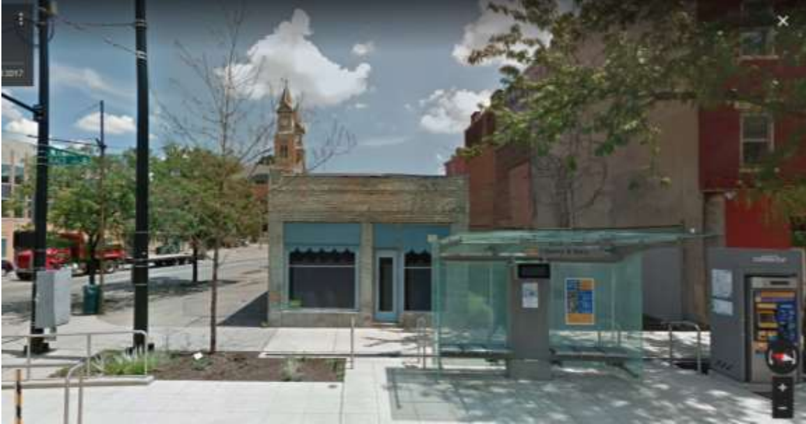
Figure 2: Front facade of existing 1538 Race Street, 2017 Google Street views.
