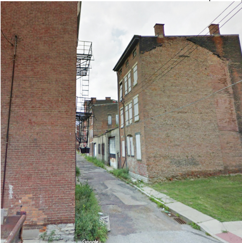
View North from Intersection of West Green Street and Campbell Alley
