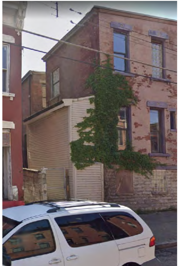
Figure 3. 1036 Dayton Street rear addition.
