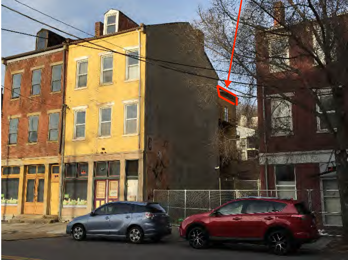
Roof deck view from McMicken Avenue
