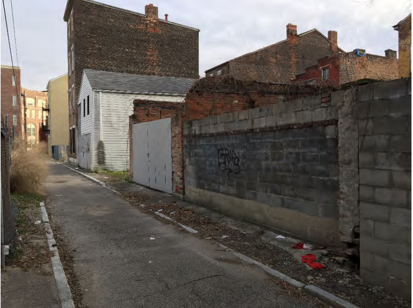
Existing walls (brick walls) from Hust Alley looking east
