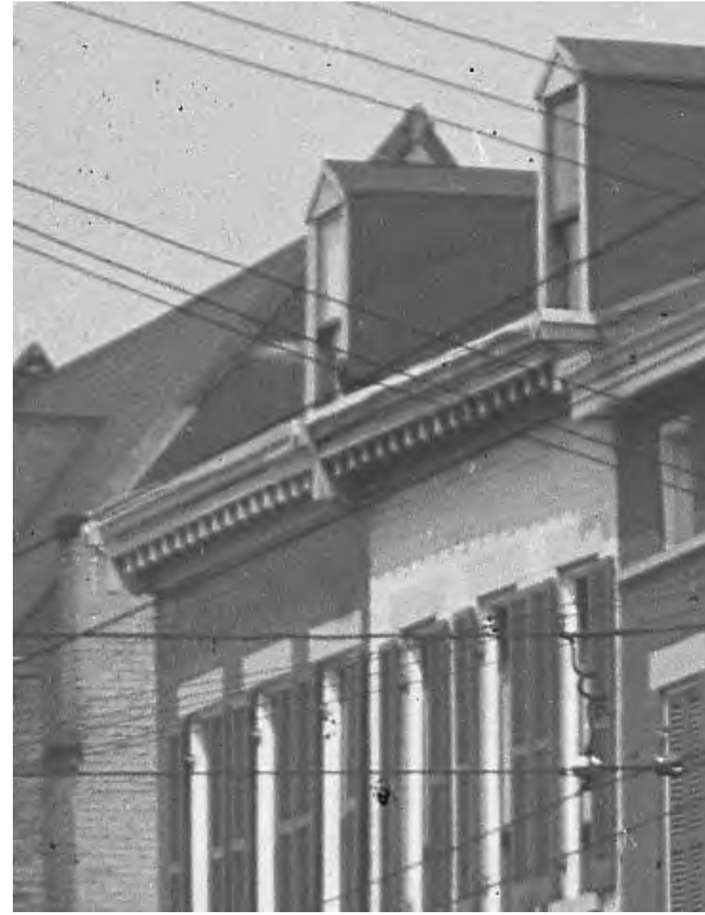
5 HISTORIC CORNICE PHOTO A3.0 Scale: NONE
