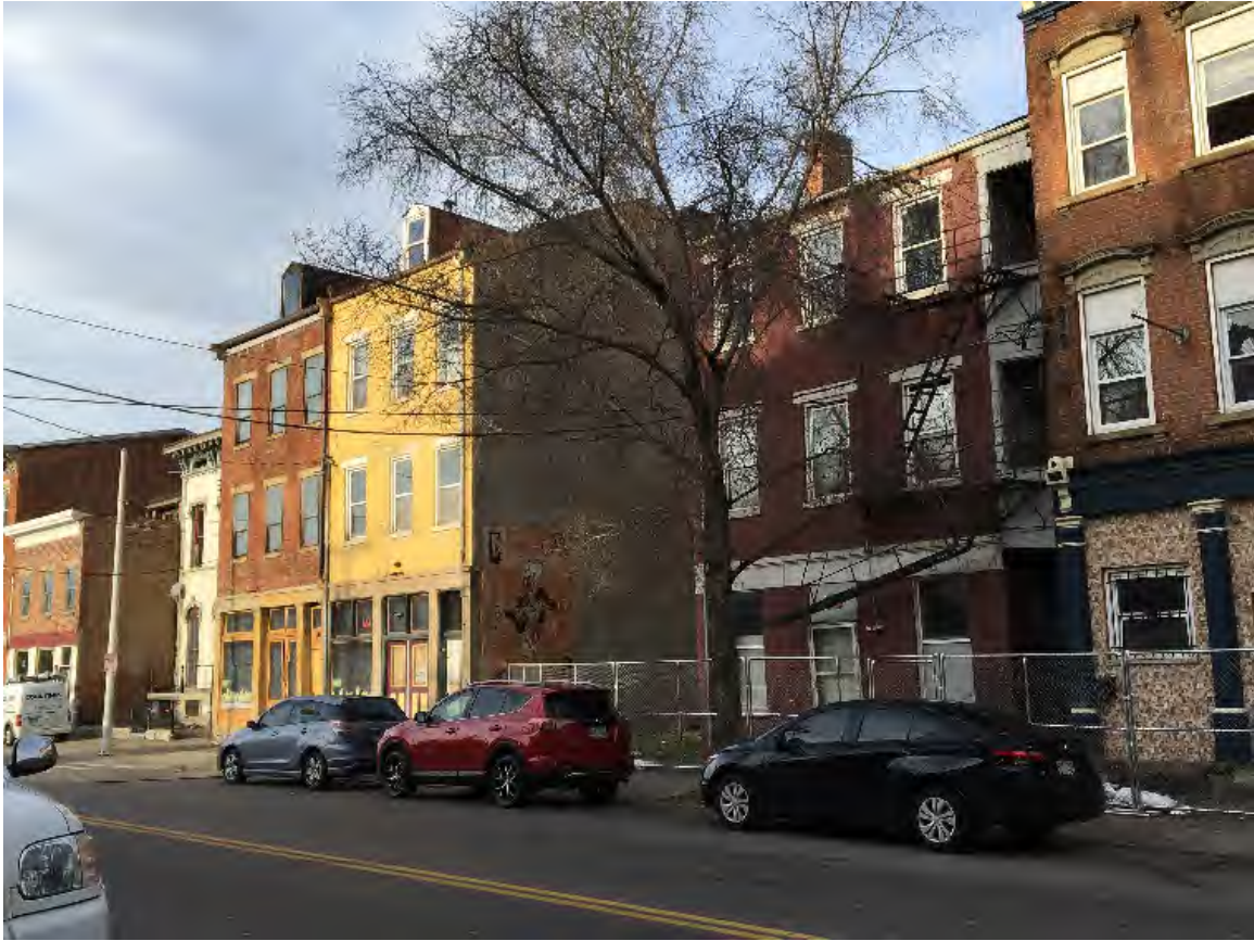
McMicken Avenue streetscape (looking west)
