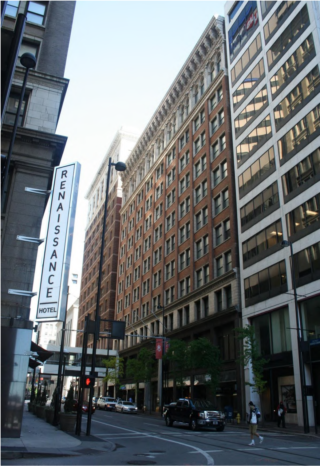
Mercantile Library Building, 414 Walnut Street, Front (West) elevation
