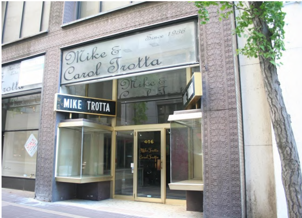
Storefront detail showing ornamental bronzed cast-iron facing
