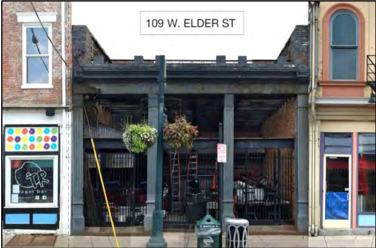
Figure 2: 109 W. Elder Street, facing south. Image from Applicant.
