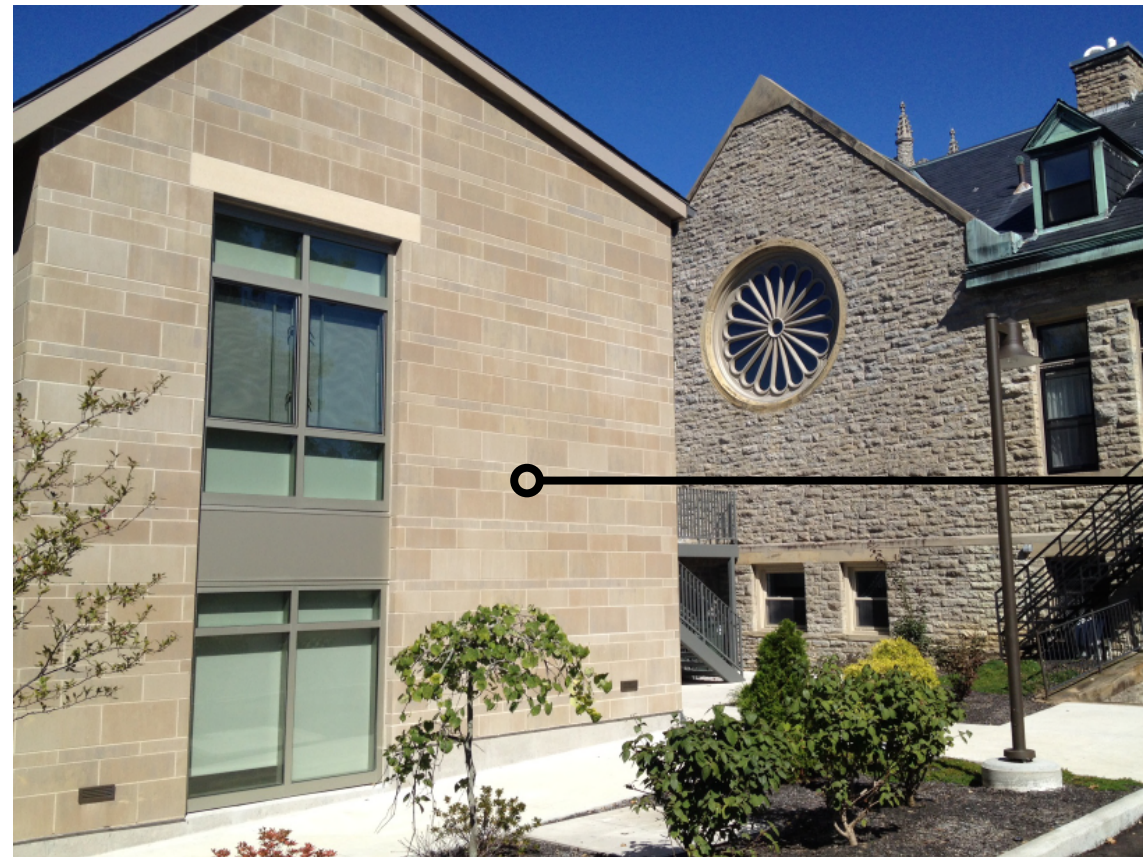
Stone - large scale block with stacked bond
