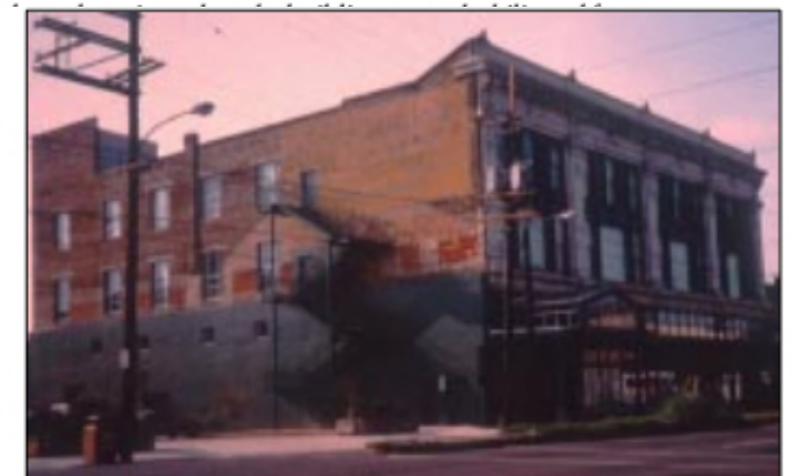
Although highly visible, because the wall is not important in defining the historic character of the building, it was possible to change the existing openings and to add several new windows to accommodate the new use.
