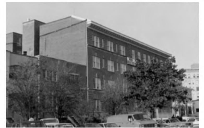
New rooftop addition and stairtower visible on the south elevation.
