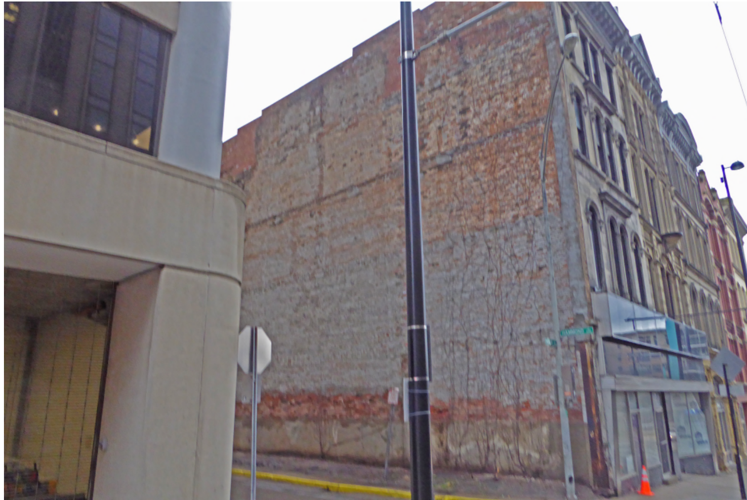
Existing street view
