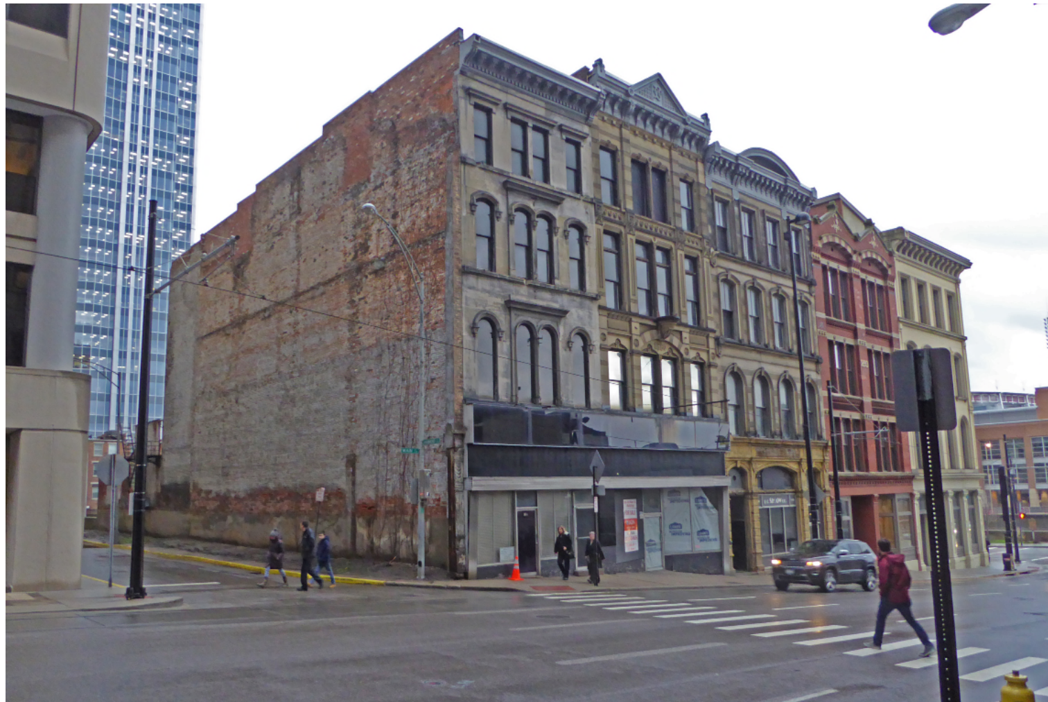
Existing street view
