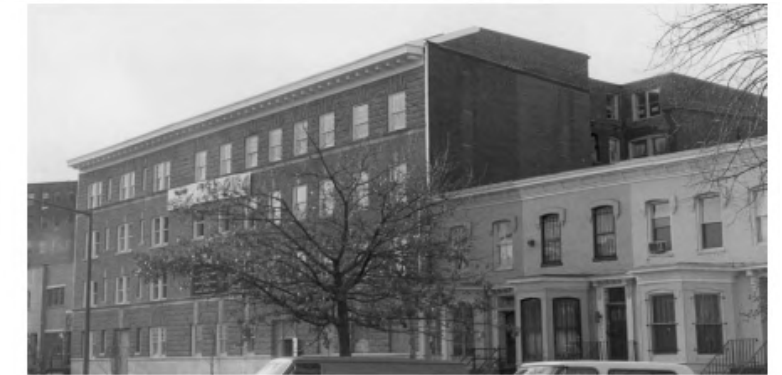
New rooftop addition and stairtower visible on the secondary north elevation, meets the Standards, and is compatible with the historic building.
