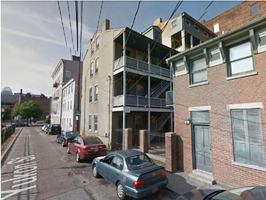
Figure 2. Street view of 215 Woodward. Image from Google.
