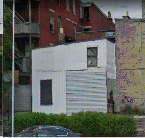
4 EXIST. SOUTHWEST PHOTO SCALE: NTS
