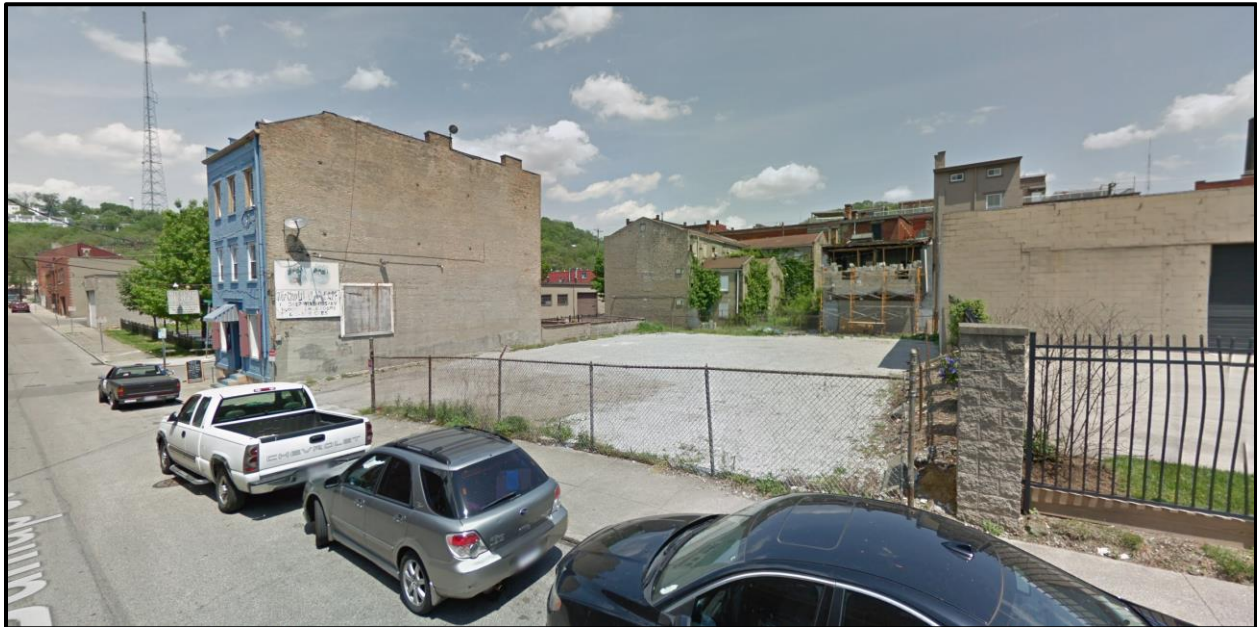
Figure 2: Image of 1920-1922 Dunlap Street. Image from Google. Note the fencing to the south, which is recommended to be continued along this frontage, including the column design.
