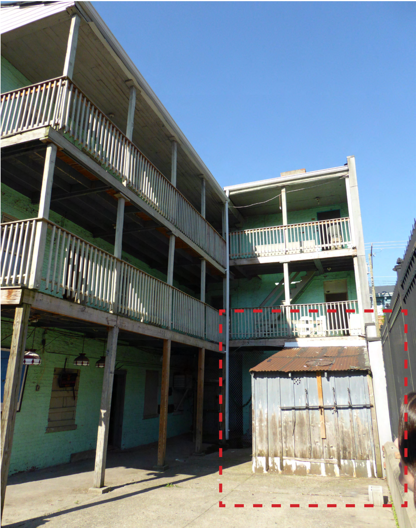
Existing Photo of shed from courtyard looking west
