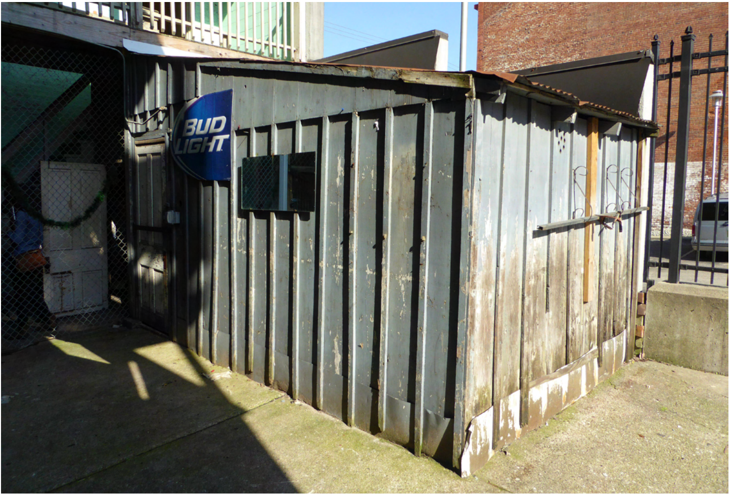
Existing Photo of shed from courtyard looking northwest
