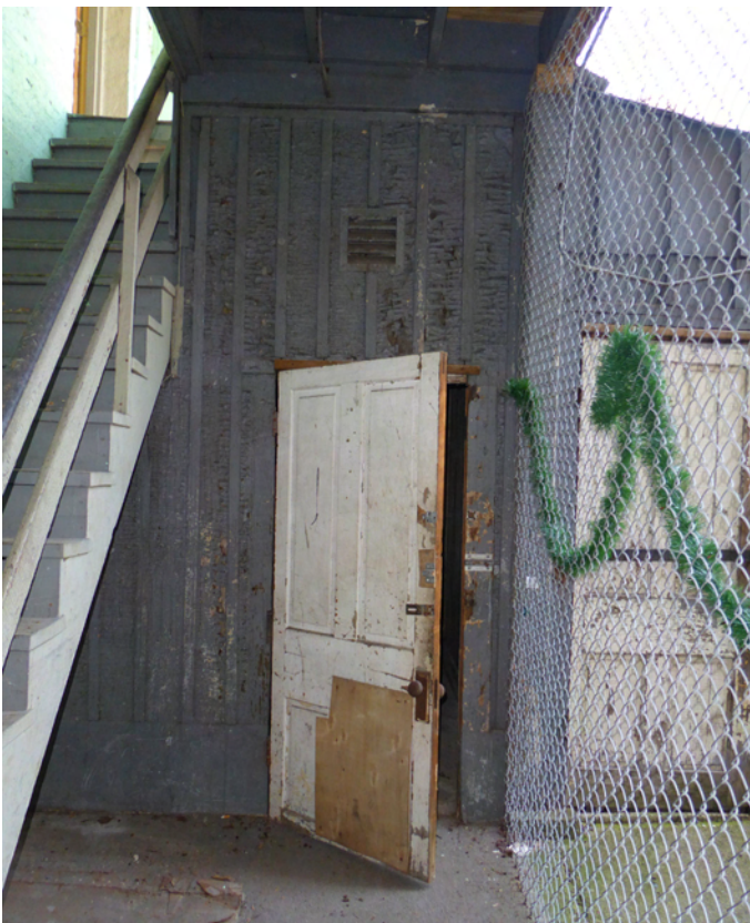
Existing Photo of shed from below deck, looking north
