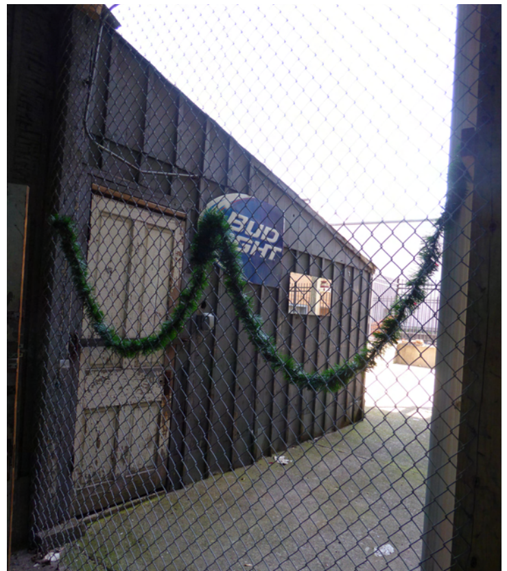
Existing Photo of shed from below deck, looking northeast
