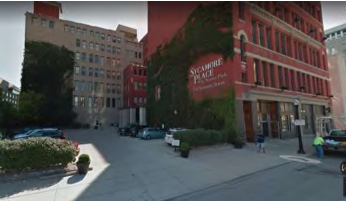
Figure 3. Image of 634 Sycamore Facades under review. Image from Google circa 2017.
