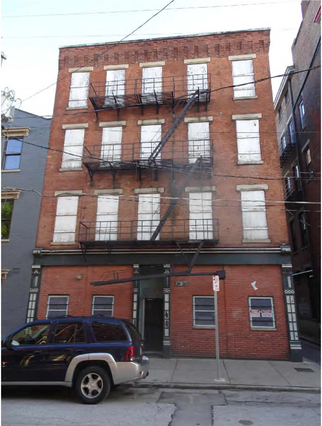
Existing South [15th Street] Elevation
