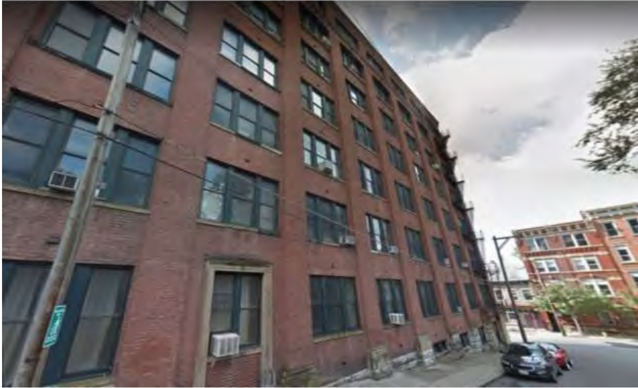
Figure 4: Pendleton Arts Center and former shoe manufacturing building.
