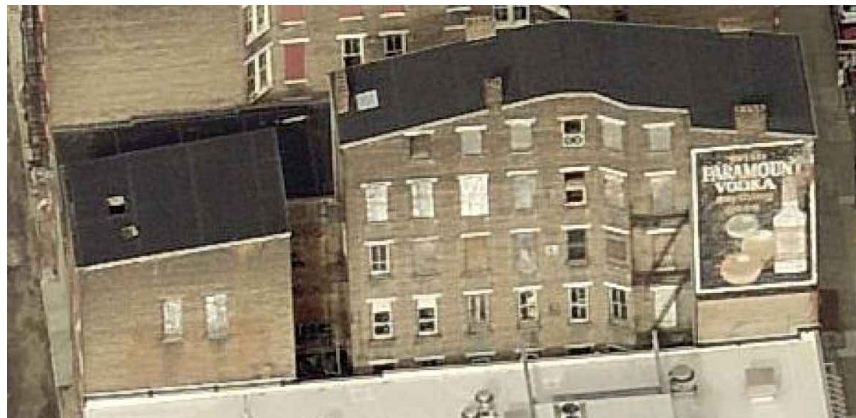
E SOUTH ELEVATION AERIAL VIEW FROM SOUTH
