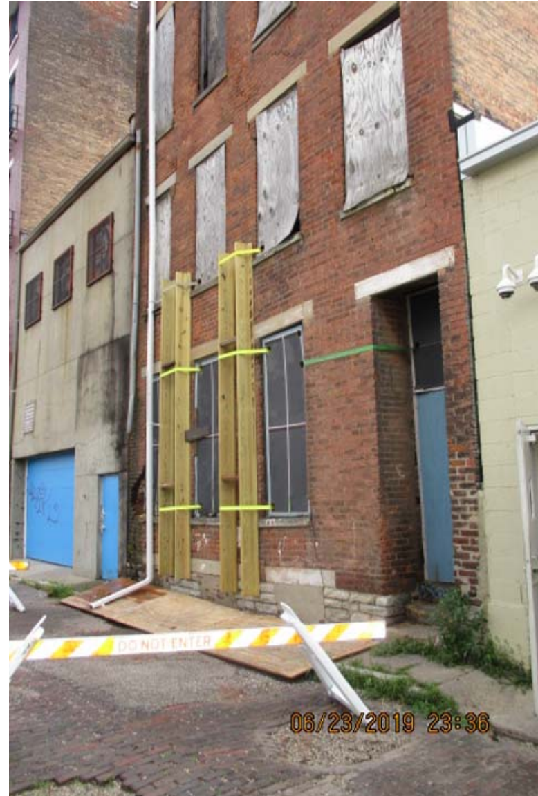
1725 Elm Rear Bldg West Facade
