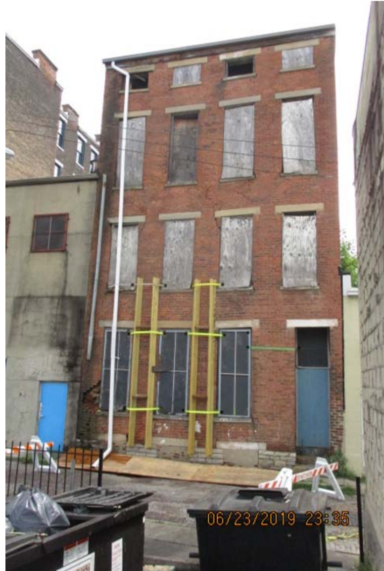
1725 Elm Rear Bldg West Facade
