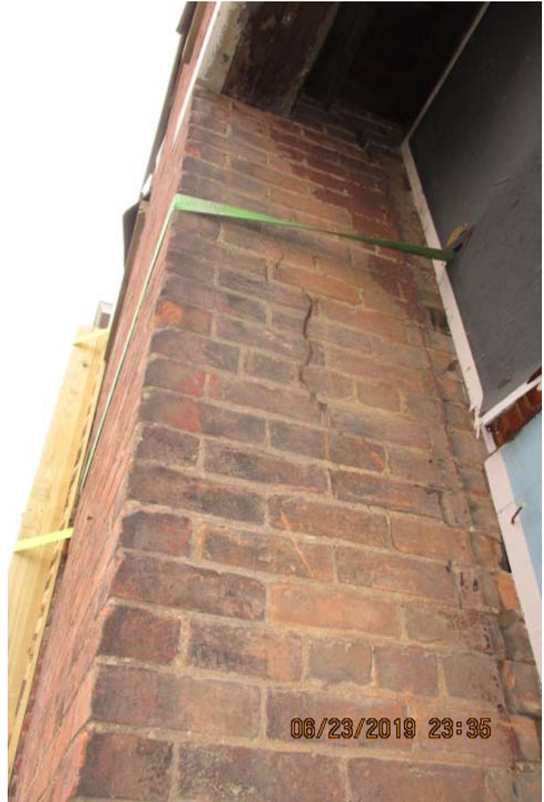
1725 Elm Rear Bldg West Facade
