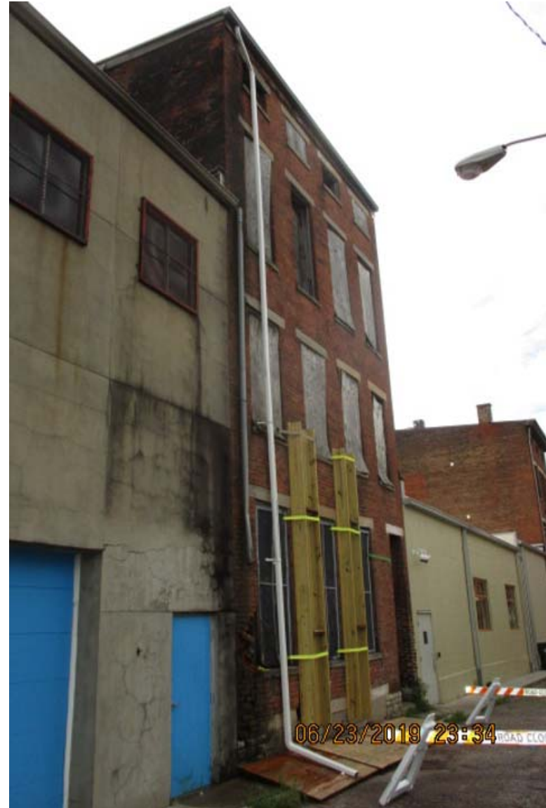
1725 Elm Rear Bldg West Facade
