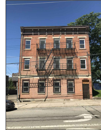
ELM STREET - PRIMARY FACADE
