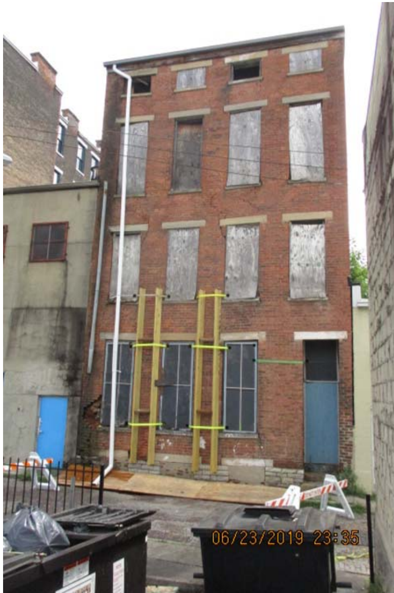
1725 Elm Rear Bldg West Facade
