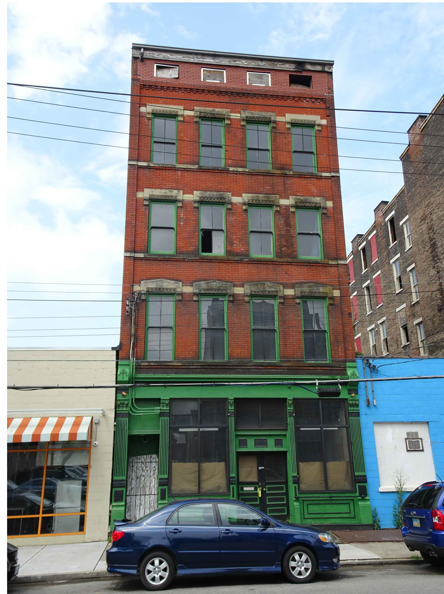
B EAST ELEVATION VIEW FROM ELM STREET
