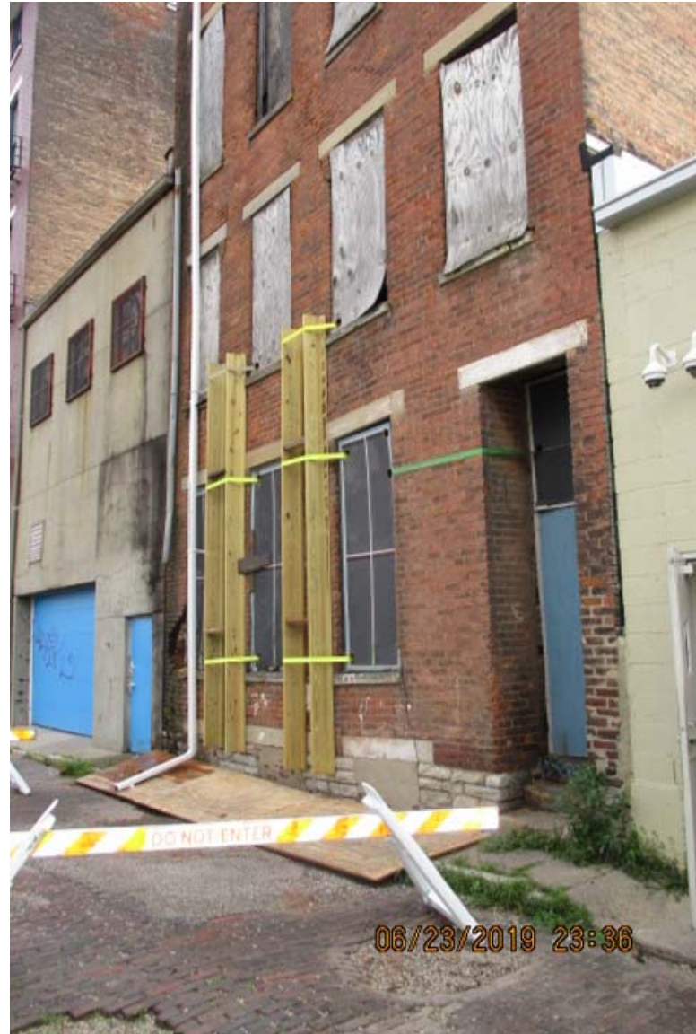
1725 Elm Rear Bldg West Facade
