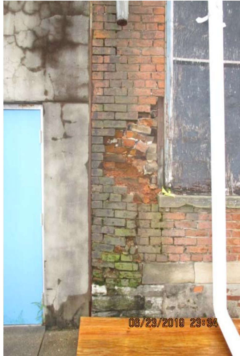
1725 Elm Rear Bldg West Facade
