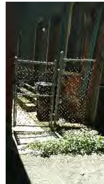
Existing non-locking Rear Gate (seen from Kirk Alley)
