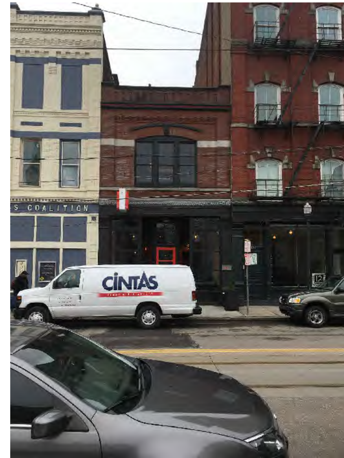
A. North facade [along 12th St.] as viewed from opposite sidewalk
