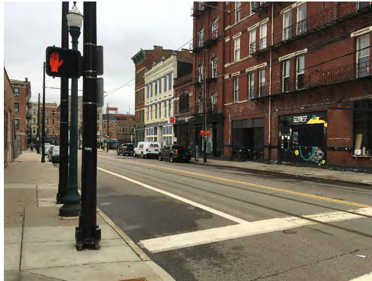
B. North Facade [along 12th St.] as viewed from West showing streetscape context
