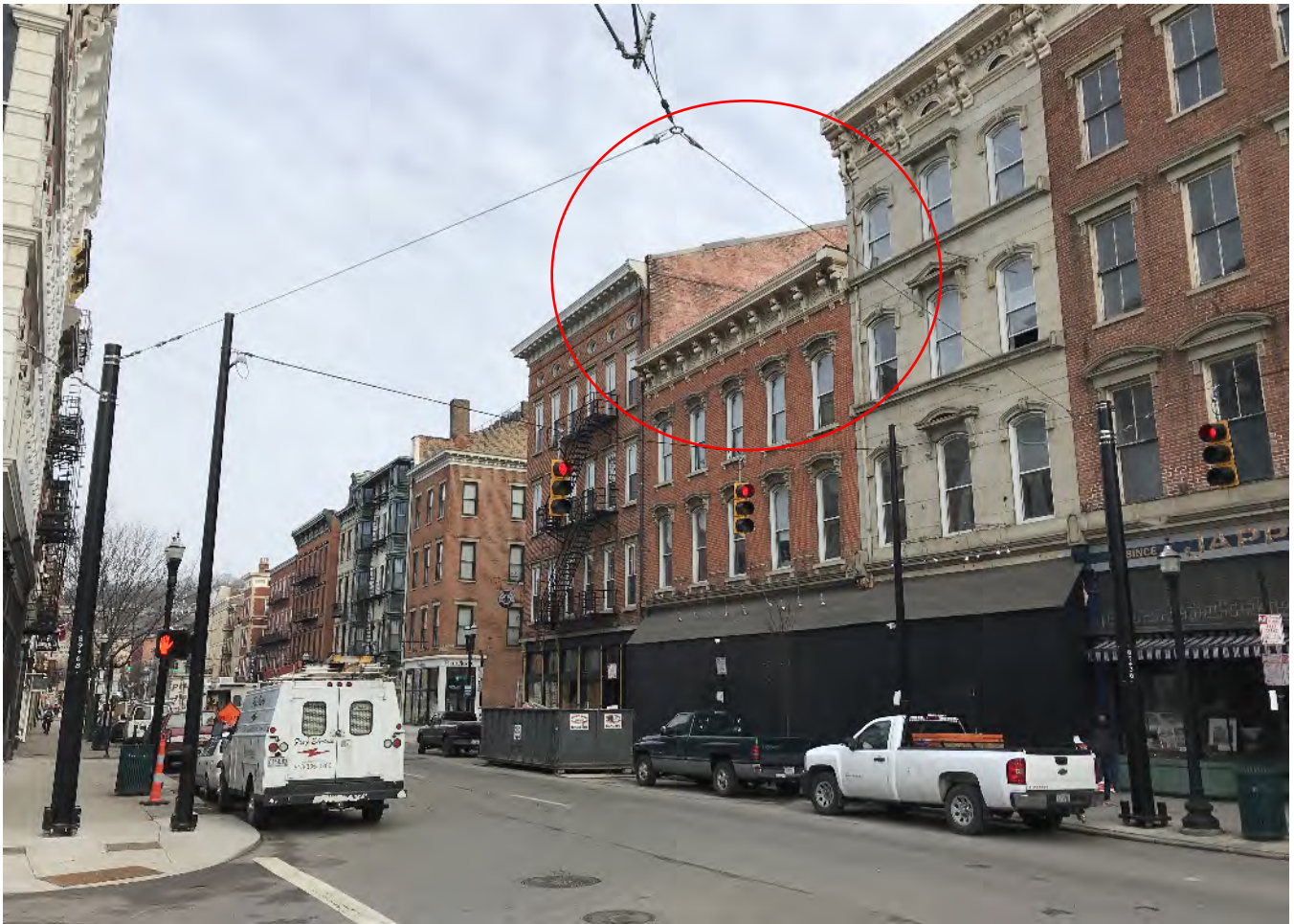
MAIN STREET LOOKING NORTH - MOCK UP NOT VISIBLE
