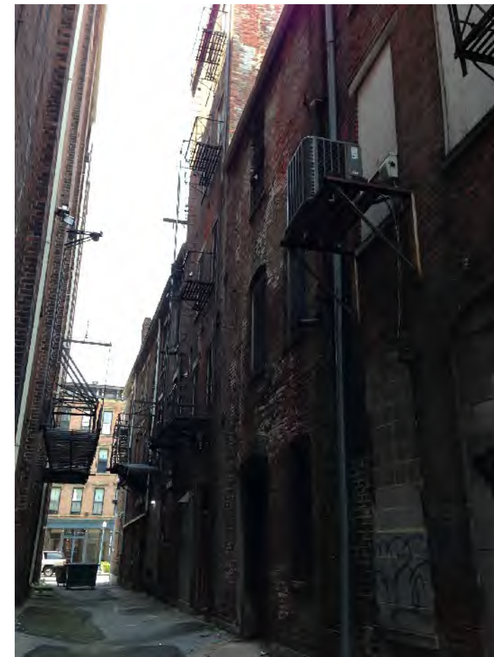
D. South Facade [from East along Wilkymacky Alley]
