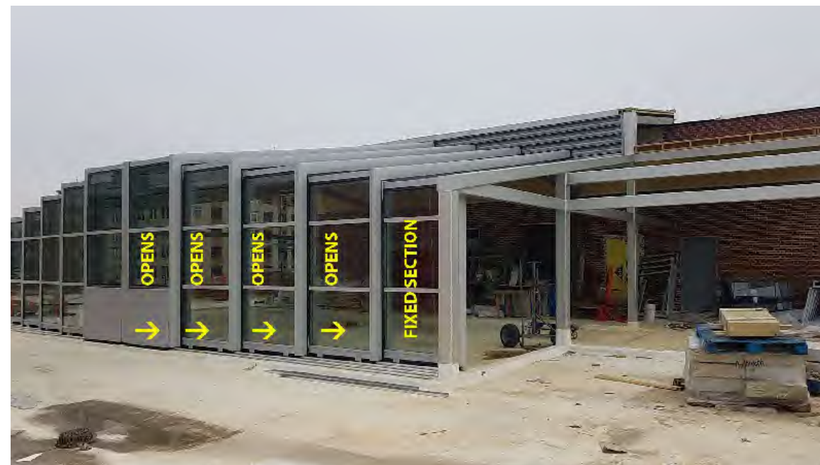
ROOFTOP LOOKING NORTH EAST
