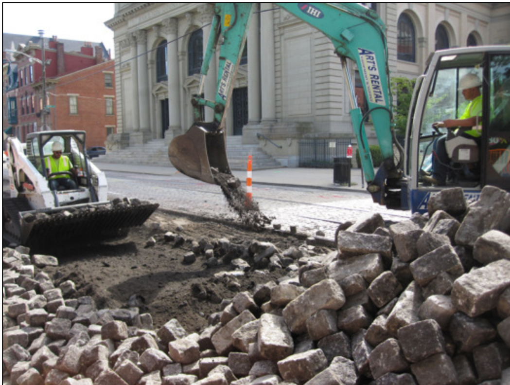
Photo 5 - Crews remove granite pavers for storage before resetting on Elm Street.
