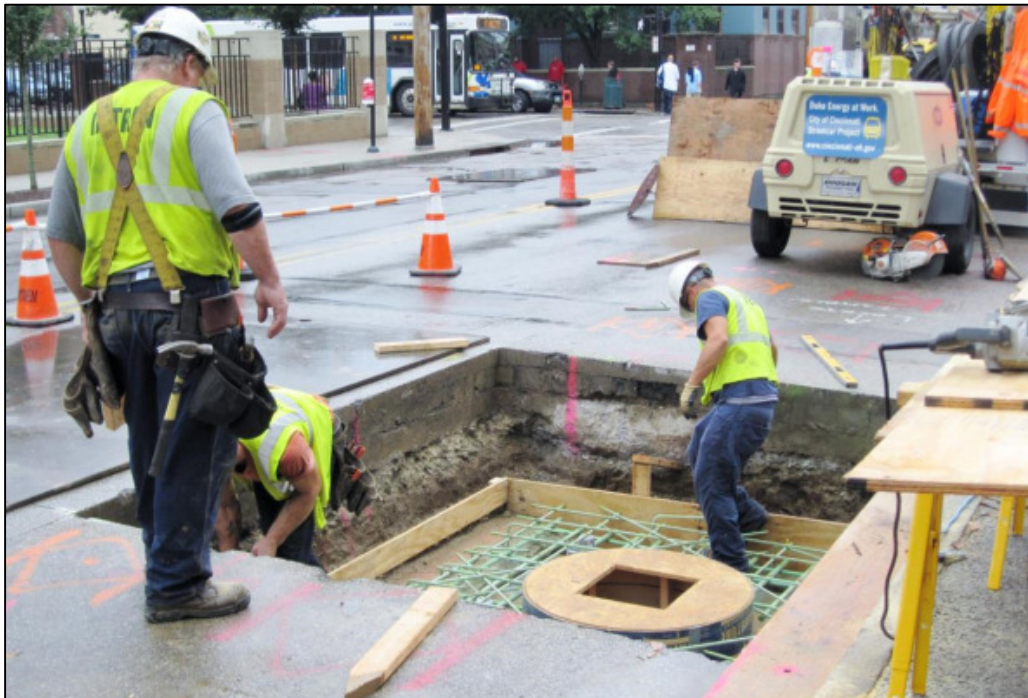
Photo 11 - Duke crews install a new manhole roof on 12th St.
