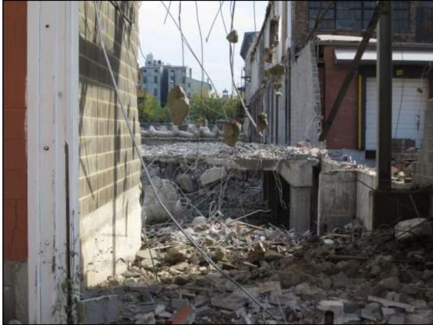
Photo 6 - Demolition at the MOF site
