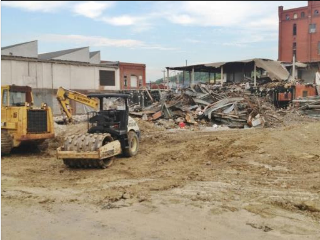
Photo 4 - Demolition work at the MOF site
