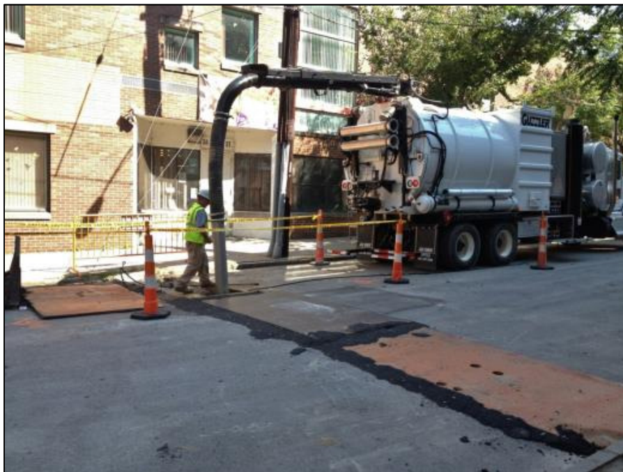
Photo 3 - Potholing crews perform exploratory excavations on Race St. near Green
