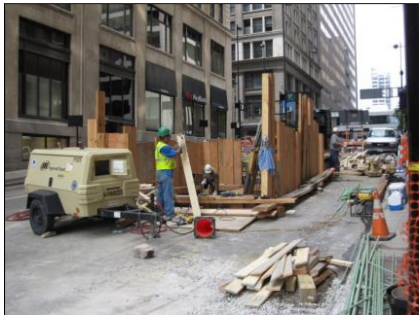
Duke Energy electric work on Walnut St. near 4 th St.
