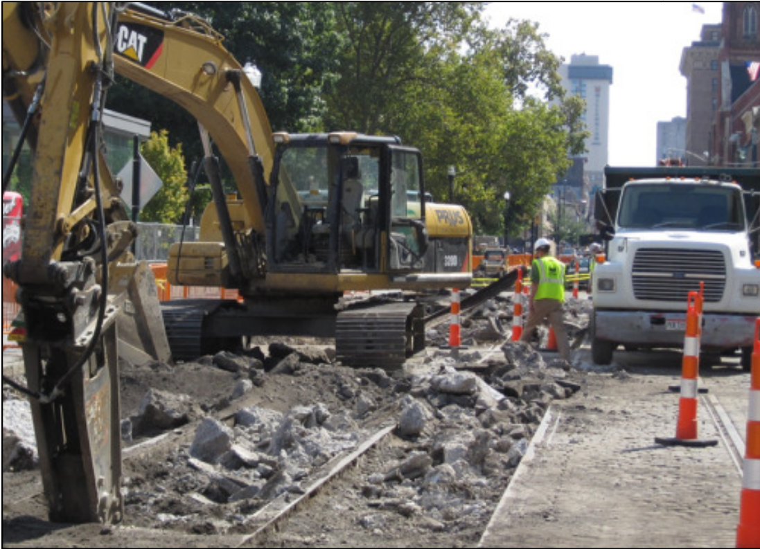
Photo 1 - Crews on Elm Street remove old streetcar rail and granite cobblestones
