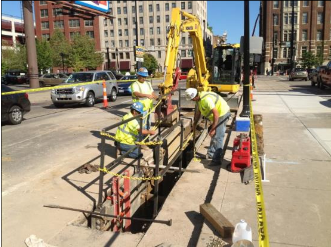
Photo 9 - Crews relocate water mains along Walnut St. near Central Parkway
