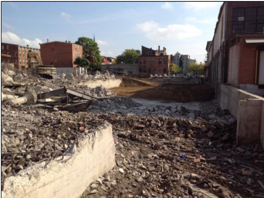
Photo 7 - Demolition at the MOF site
