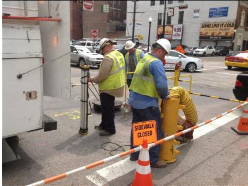
Duke Energy electric work on Walnut St. near 7 th St.
