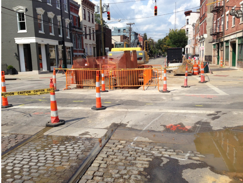
Photo 10 - Sewer manhole work at 14 th and Elm Streets
