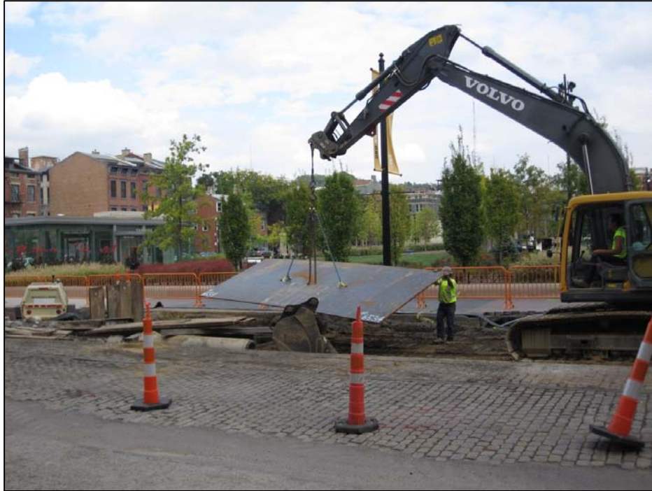
Photo 2 - Crews repair a collapsed sewer along Elm St.
