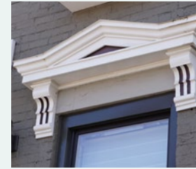
Decorative metal header at 1418 Elm Street.
