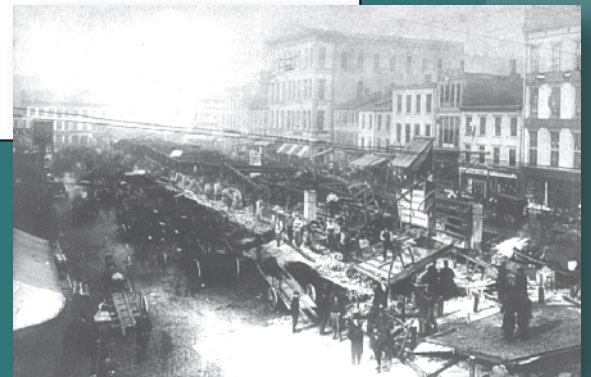
Demolition of the Market House
