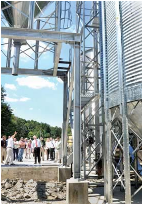
As he promoted his economic stimulus package in August 2008, Gov. Strickland visited the facilities under construction by bio-diesel producer Chieftain Biofuels.
