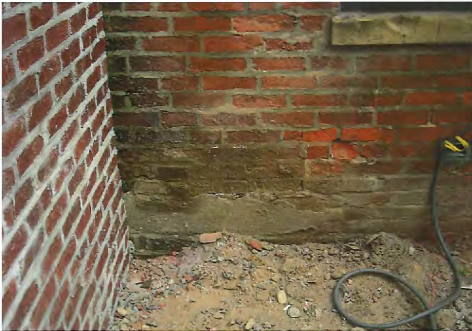
PHOTOS SHOWING MISMATCHED BRICK (COLOR, SIZE, MORTAR JOINTS, CONDITION)
