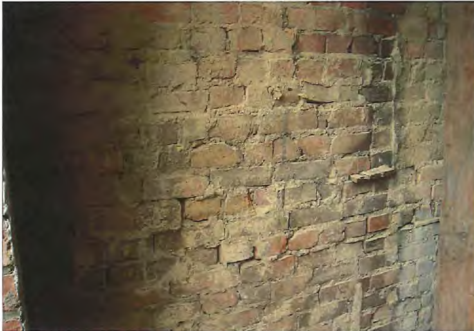
EXPOSED @ COVERED ENTRY
