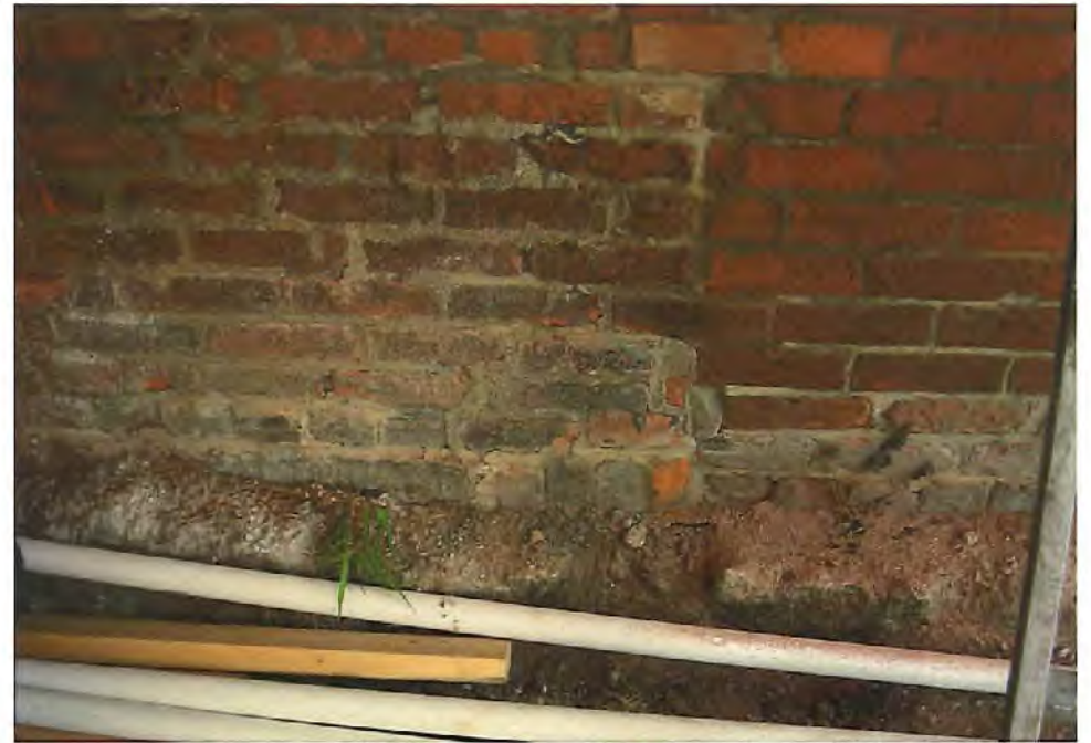
PHOTOS SHOWING MISMATCHED BRICK (COLOR, SIZE, MORTAR JOINTS, CONDITION)
