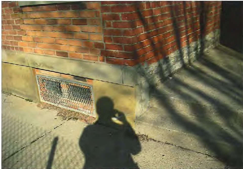
UNDER FRONT WINDOWS - FACING ELM
