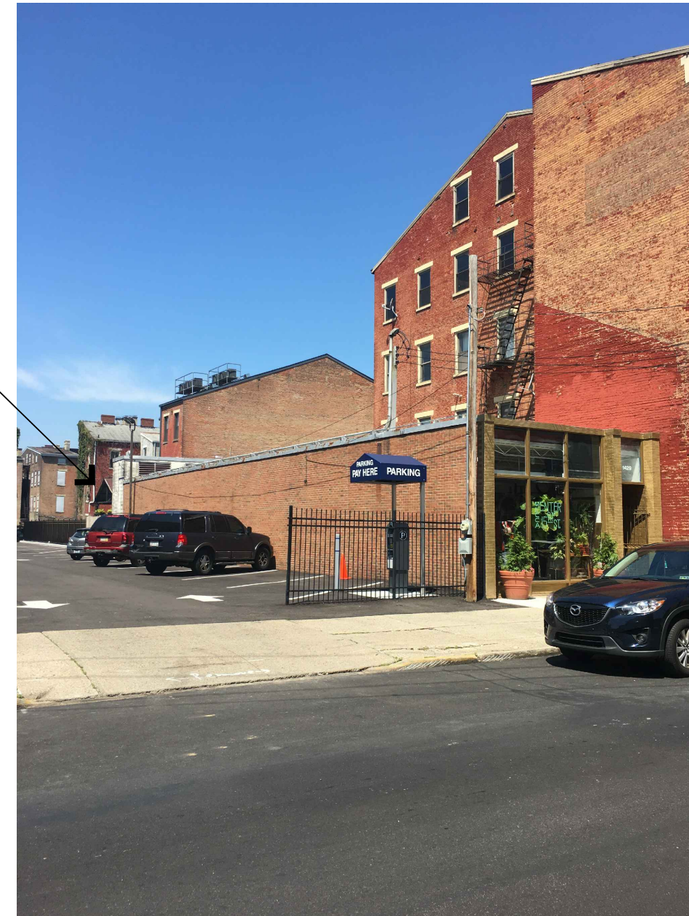
04 1423 WALNUT ST. (PARKING LOT)
