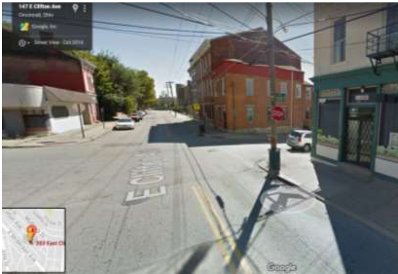
View of the building front west on Clifton
