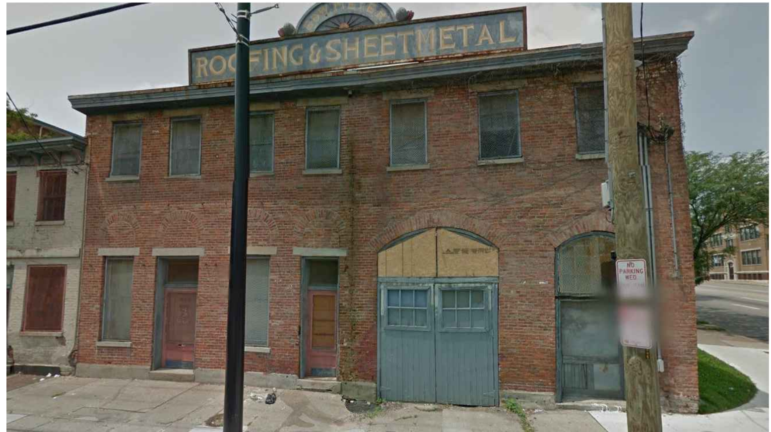
1541 ELM STREET DOUBLE DOOR OPENING NOT IN STOREFRONT
