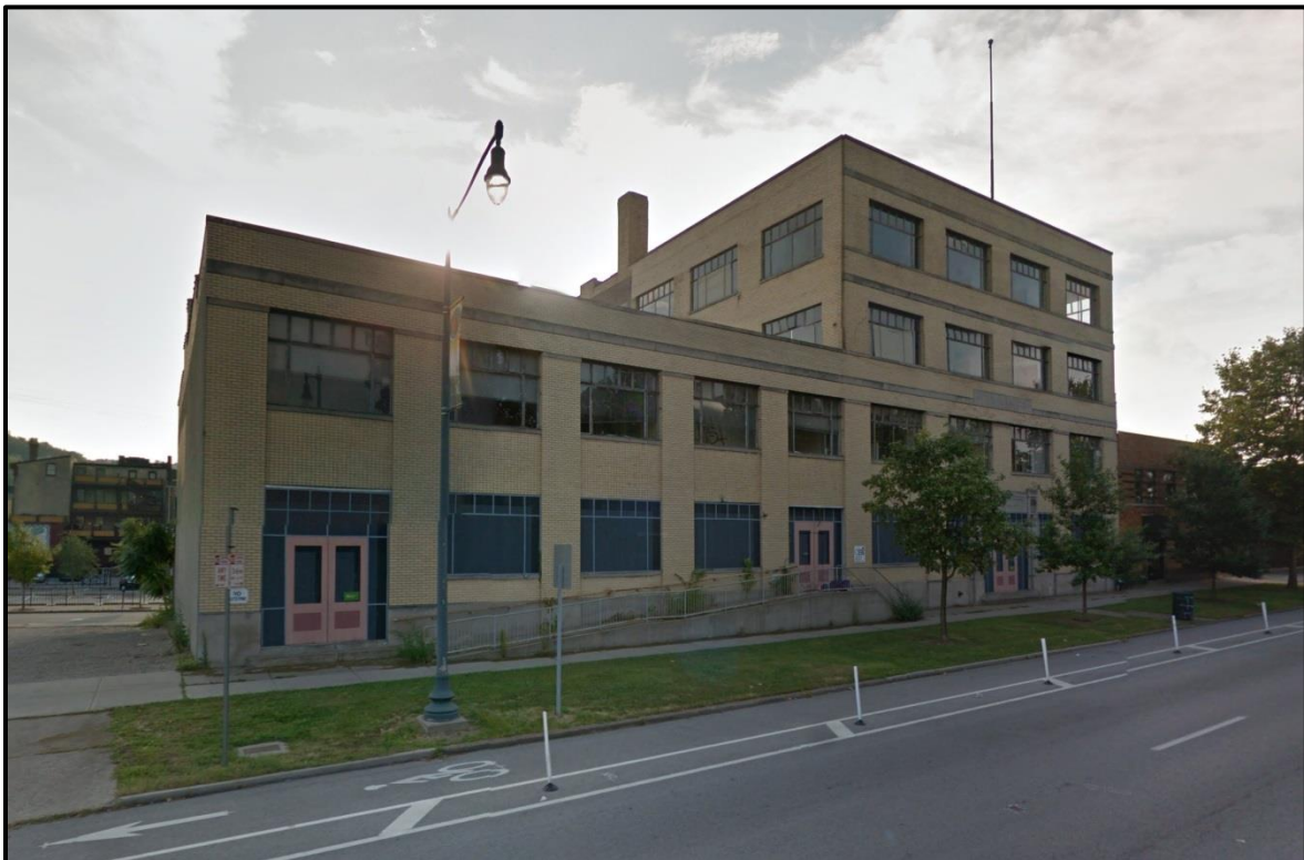
Figure 2. Existing condition of 1632 Central Parkway. Image courtesy of Google.
