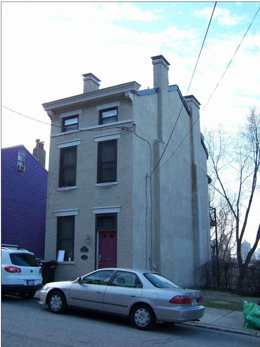
VIEW OF EXISTING BUILDING FROM MILTON STREET
