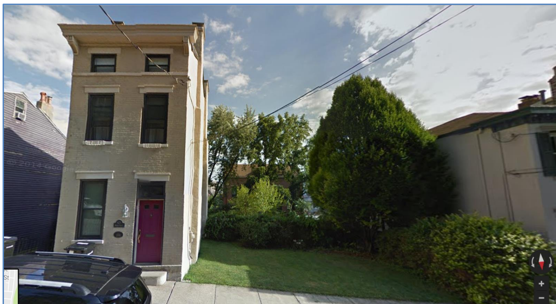
Figure 1: 423 Milton Street. Picture provided obtained from Google Street Views.
