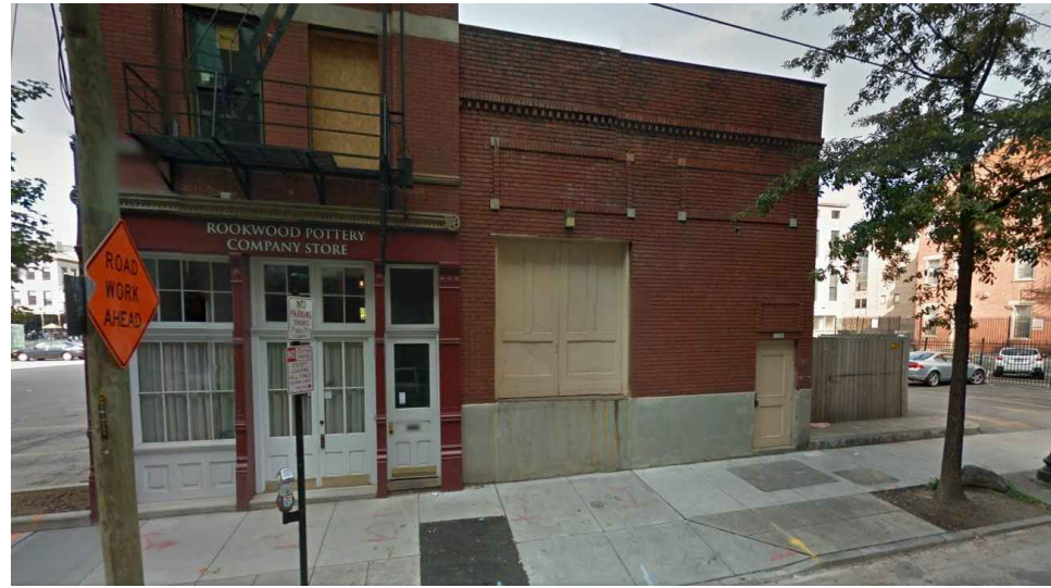
1209 JACKSON STREET DOUBLE DOOR OPENING NOT IN STOREFRONT
