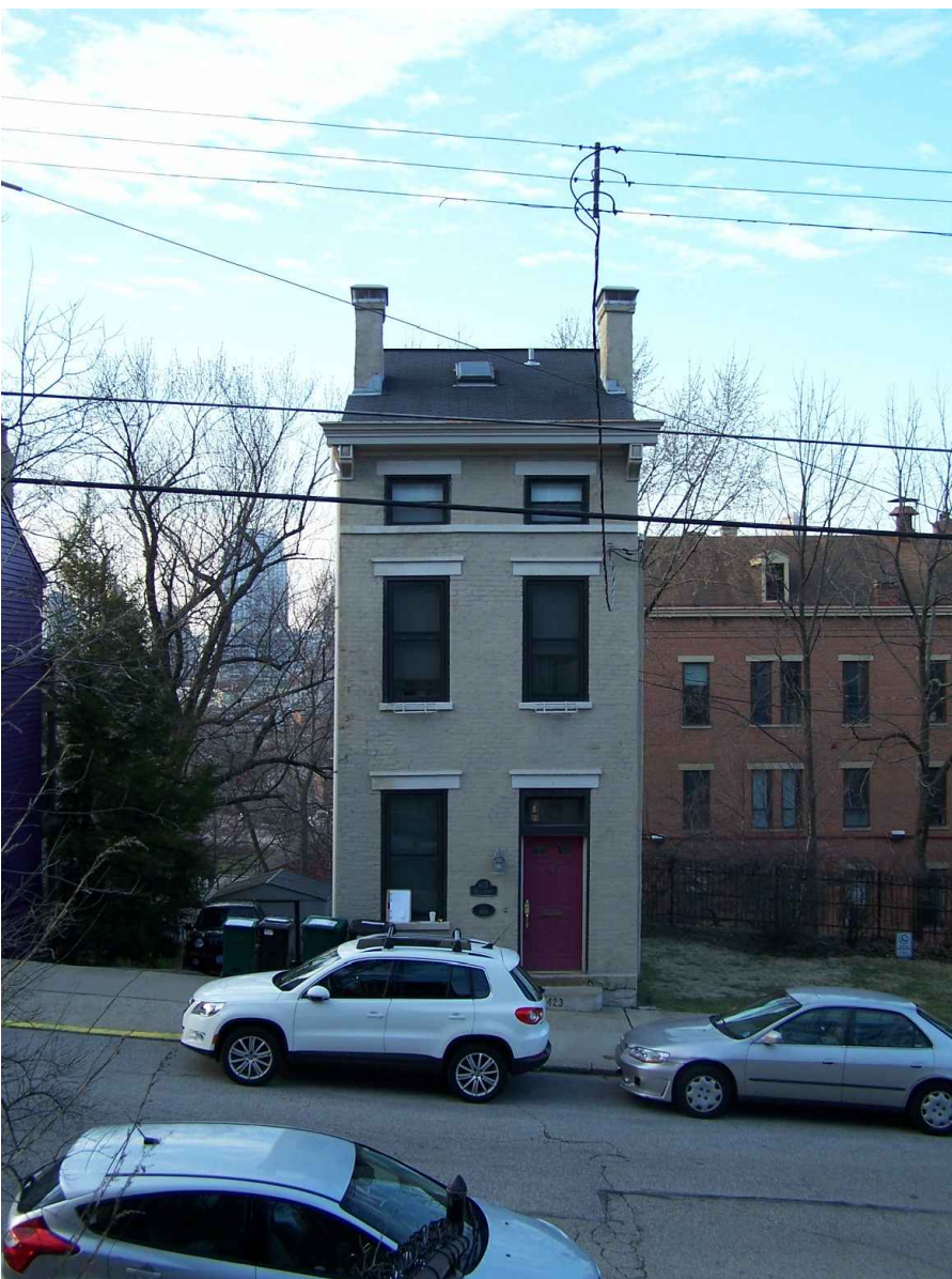
1 ELEVATION/PHOTO OF EXISTING NORTH FACADE A1.0 scale: not applicable
