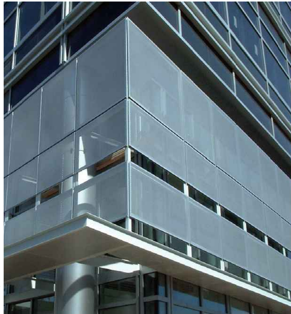
PERFORATED METAL ON OUTSIDE FACE OF GUARDRAIL FRAMING
