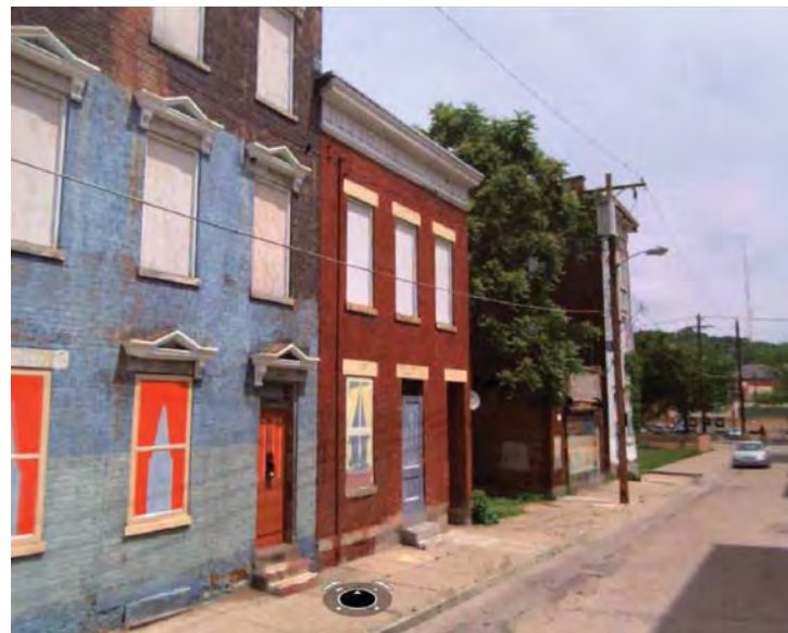
2 WADE STREET LOOKING EAST A0.2 OVERALL VIEW
