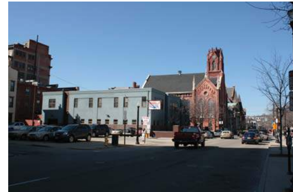
SOUTH ELEVATION - GANDOLFO ALLEY 217 W. 12th STREET 2 Story Masonry Structure
