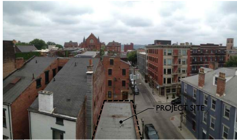
1 CONTEXT FROM ADJACENT ROOFTOP, LOOKING WEST
