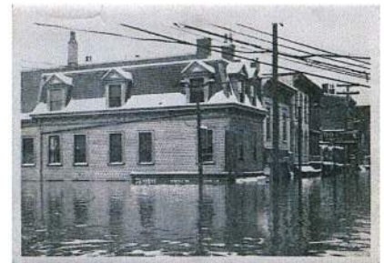
Figure 2. View of 4001 Hamilton Avenue During the Great Flood, 1937
