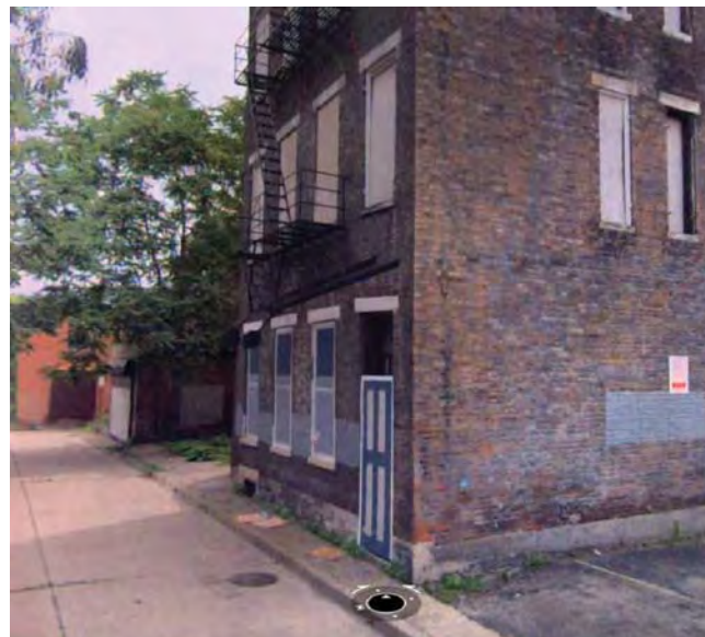
3 KEMP ALLEY LOOKING EAST A0.2 OVERALL VIEW
