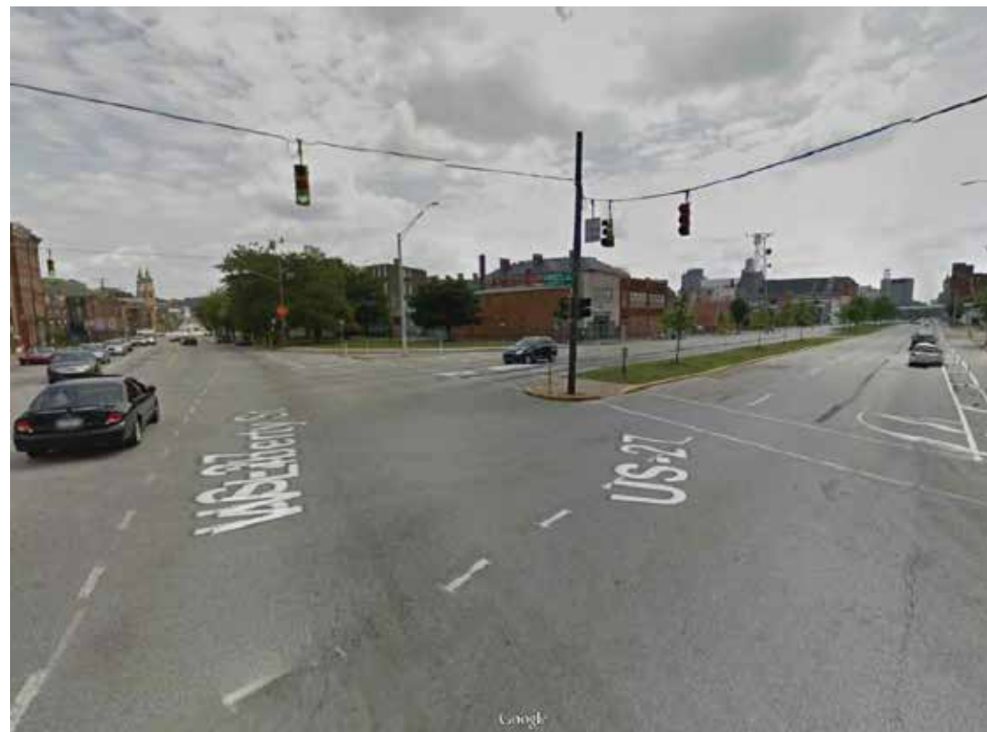
4 VIEW OF KEMP ALLEY LOOKING SOUTHEAST A0.3 FROM CENTRAL PARKWAY & LIBERTY
