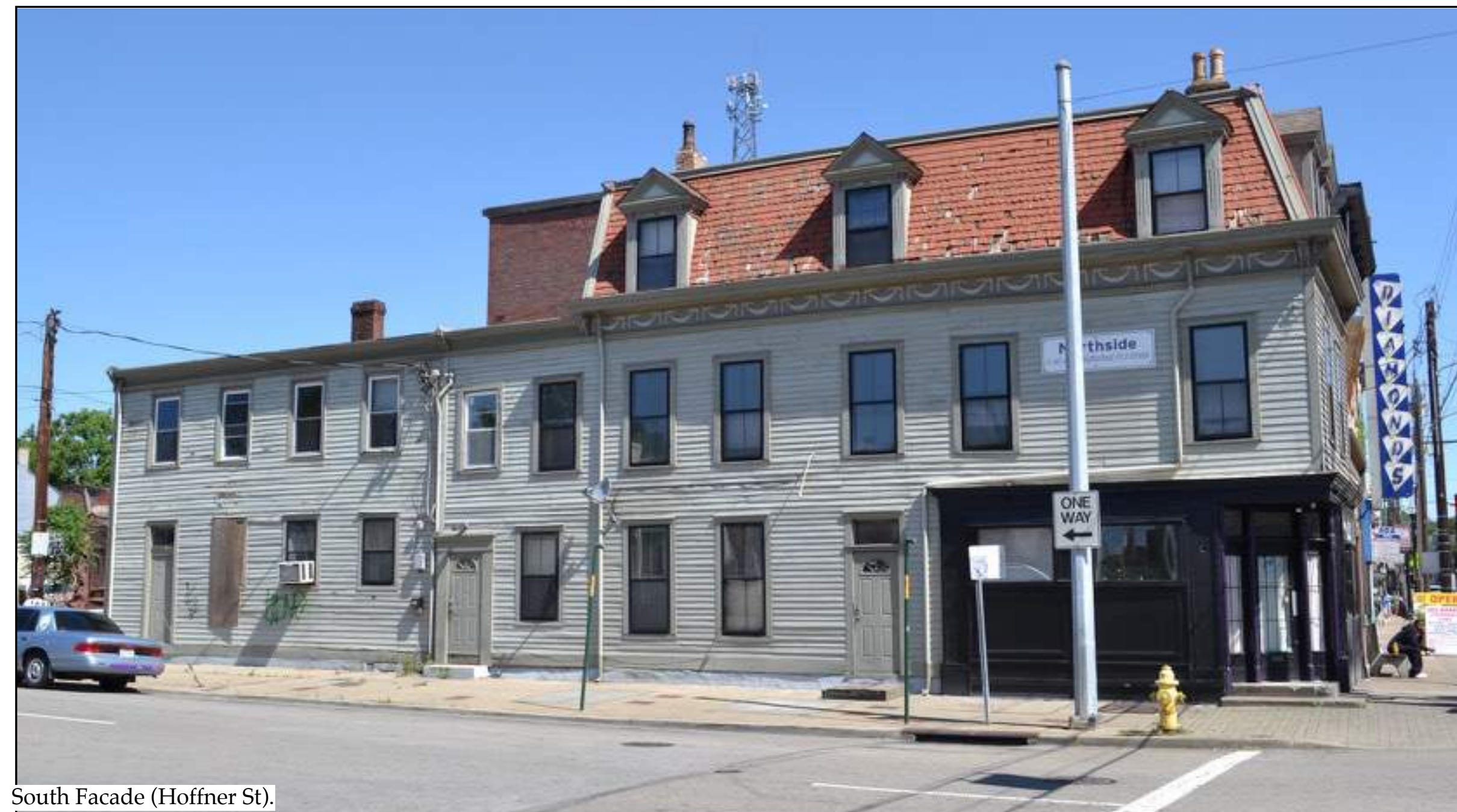
South Facade (Hoffner St).
