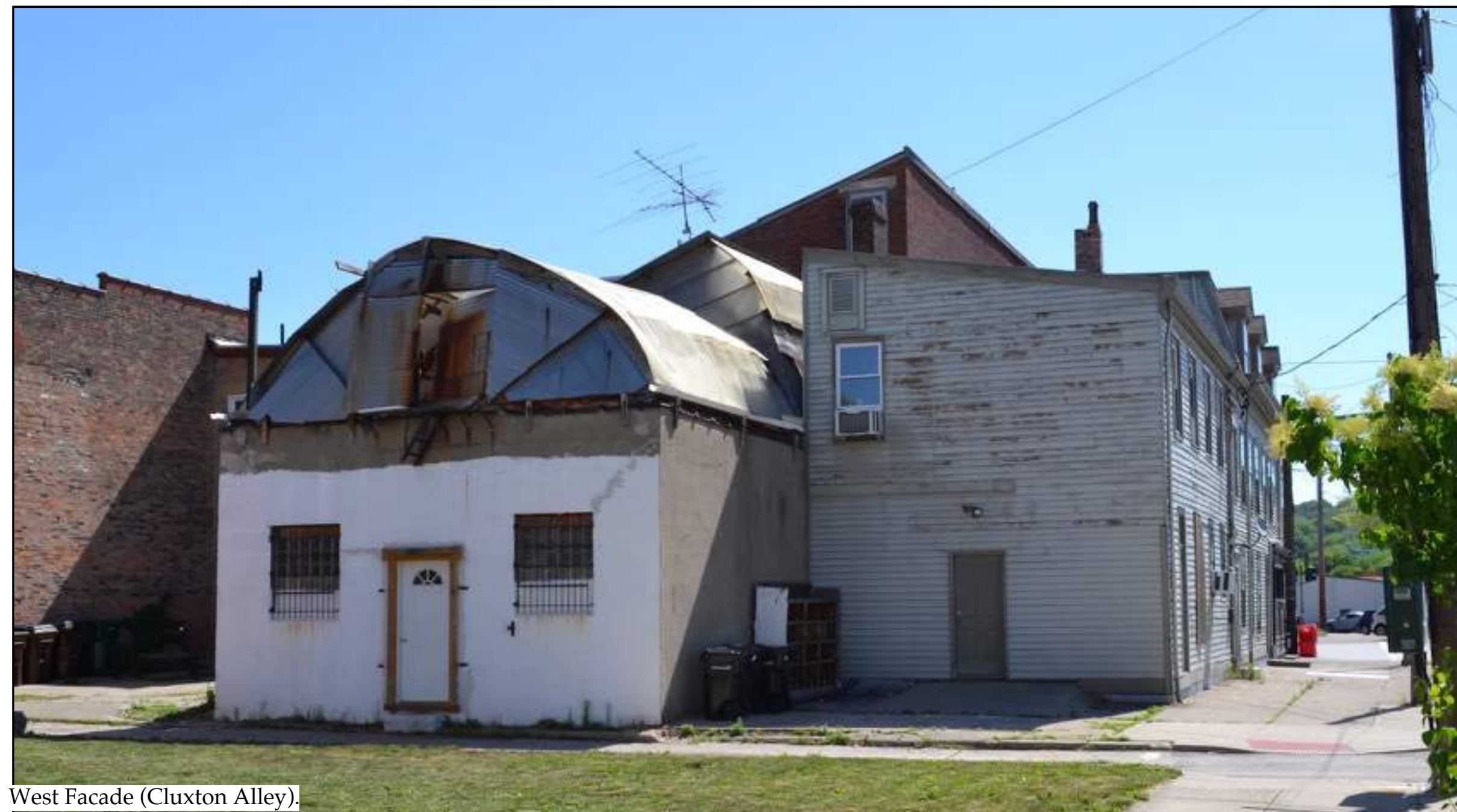
West Facade (Cluxton Alley).
