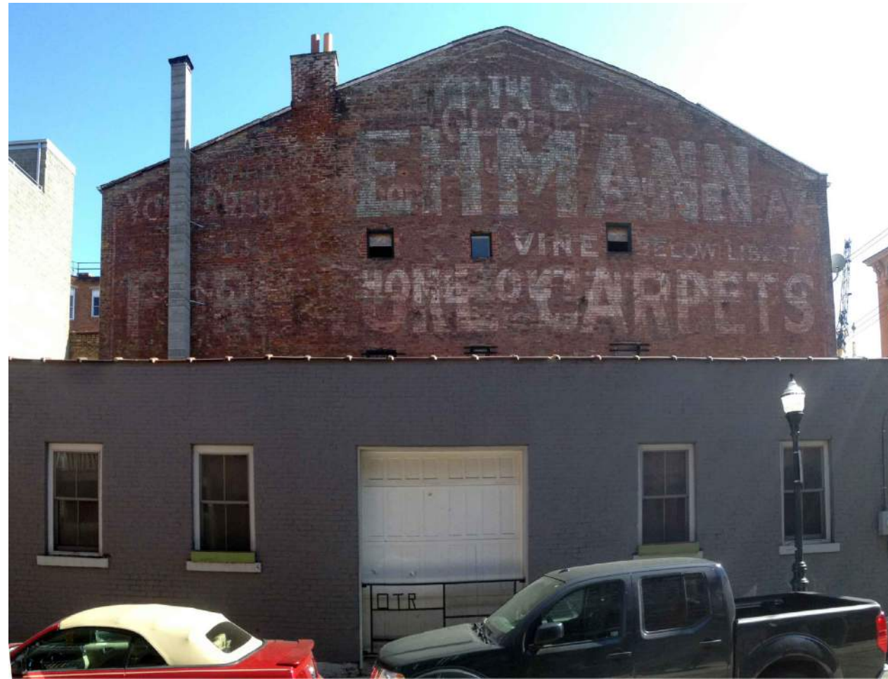
FACADE ALONG FOURTEENTH STREET
