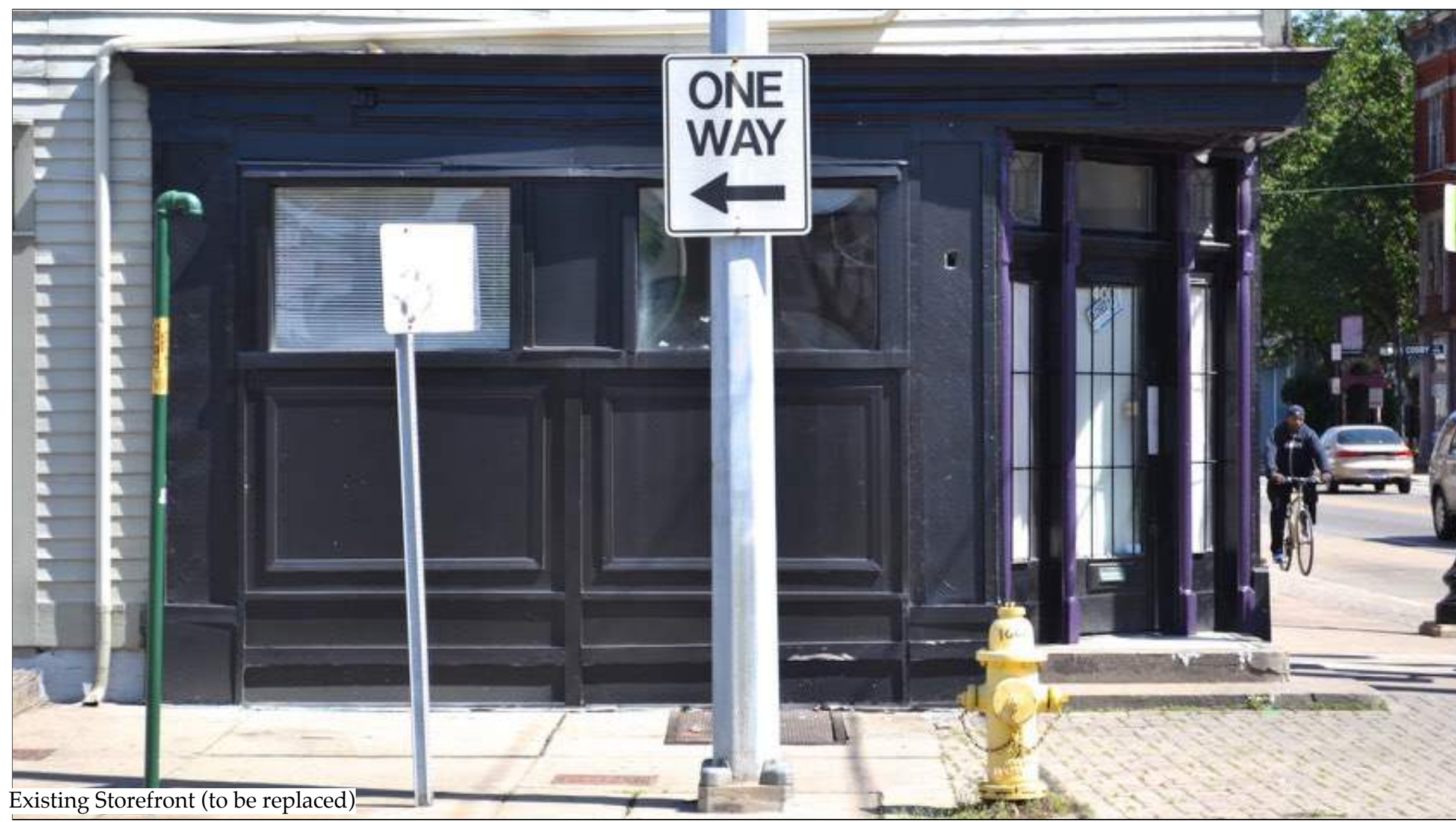
Existing Storefront (to be replaced)
