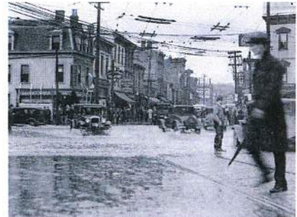
Figure 4. View of 4001 Hamilton Avenue (Stolz Pharmacy), late 1920s/early 1930s
