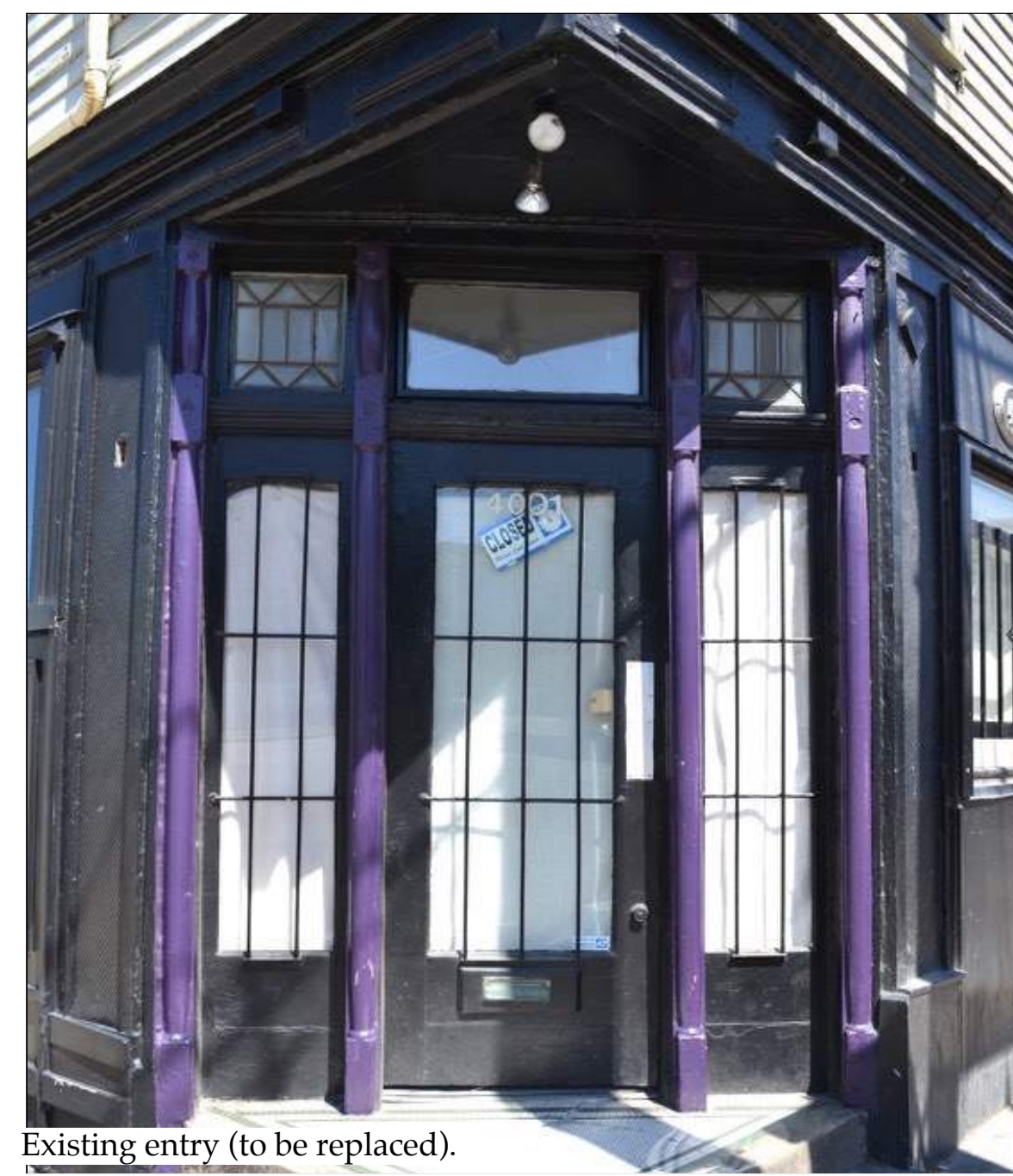
Existing entry (to be replaced).
