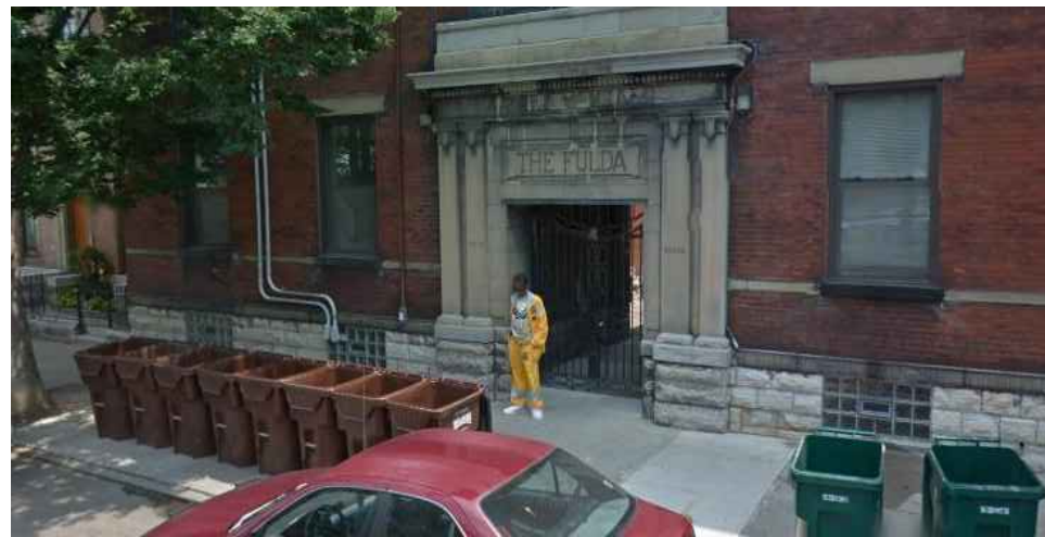
1514 ELM STREET DOUBLE GATE AT RESIDENTIAL FIRST FLOOR
