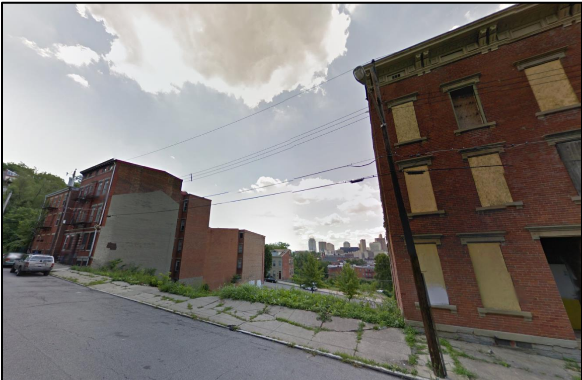
Figure 2. Existing condition of 305-309 Seitz Street (vacant lots). Image courtesy of Google.
