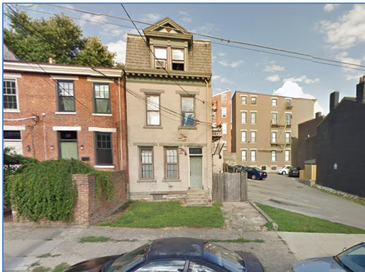
Figure 1: 1608 Mansfield. Image from Google Street Views.
