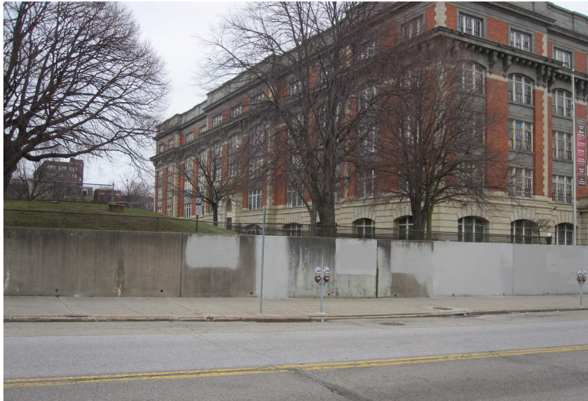
Retaining Wall Along Sycamore
