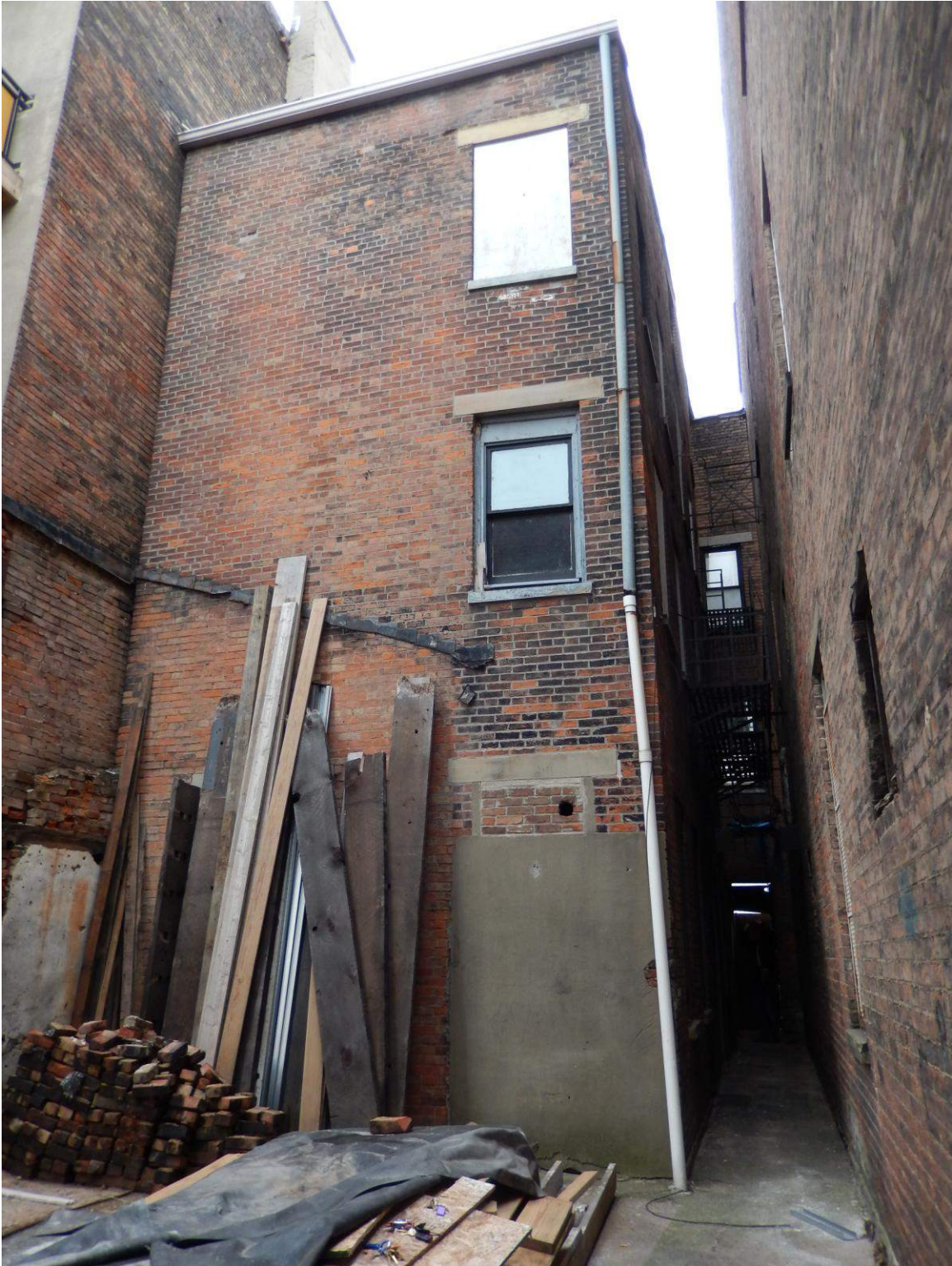
Front Building - Courtyard Elevation (West Elevation of Front Building)
