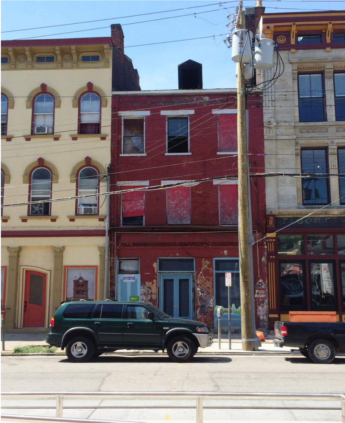
Front Building - Elm Street Facade (East Elevation of Front Building)
