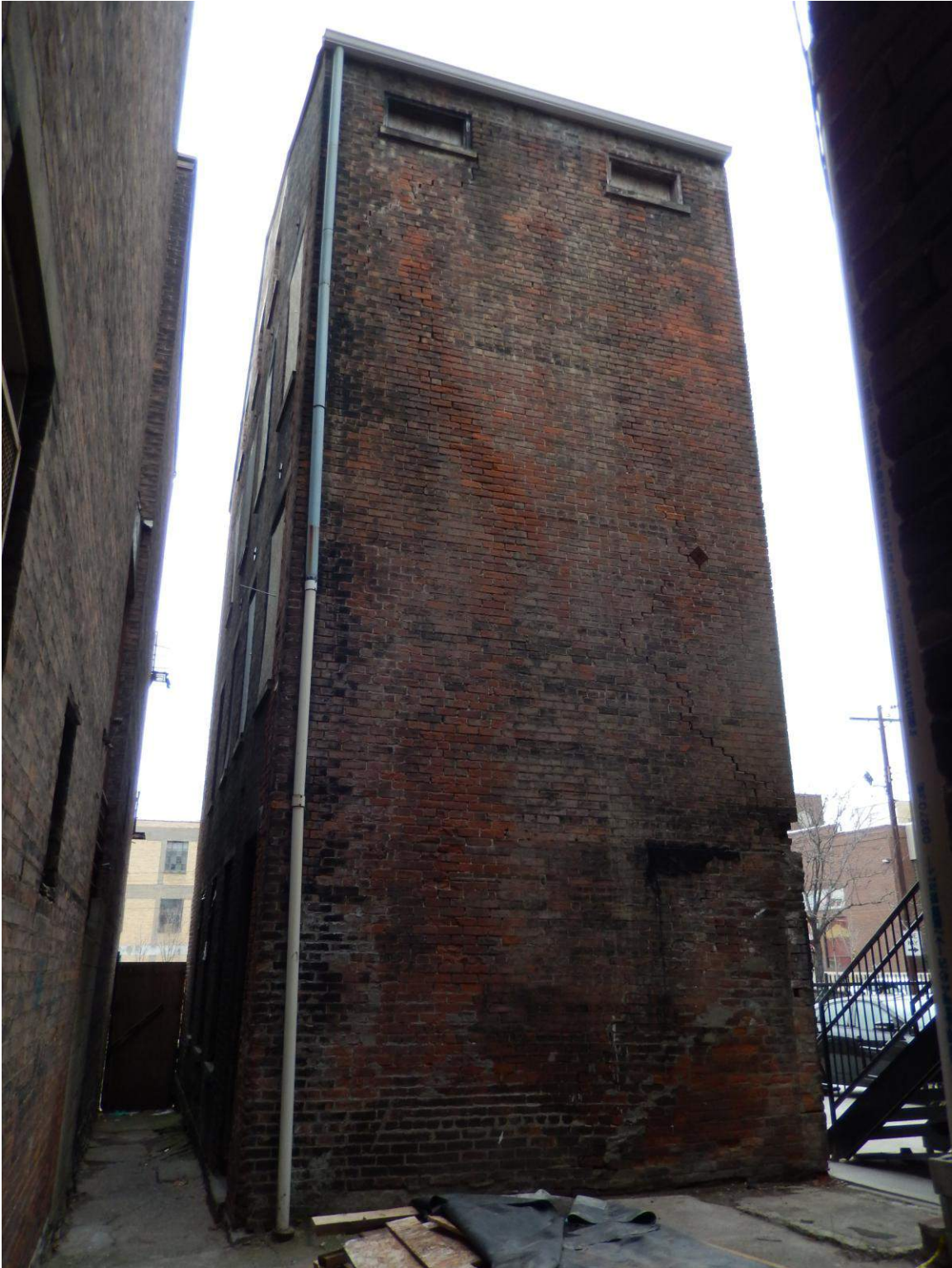
Rear Building - Courtyard Facing Facade (East Elevation of Rear Building)
