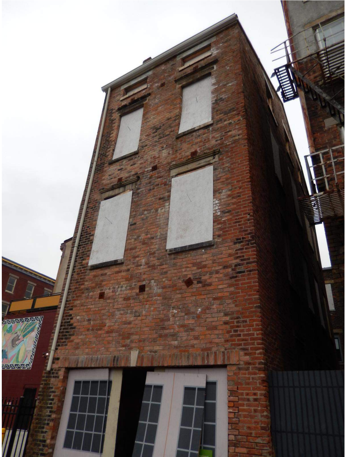
Rear Building - Facade Facing Campbell Alley (West Elevation of Rear Building)
