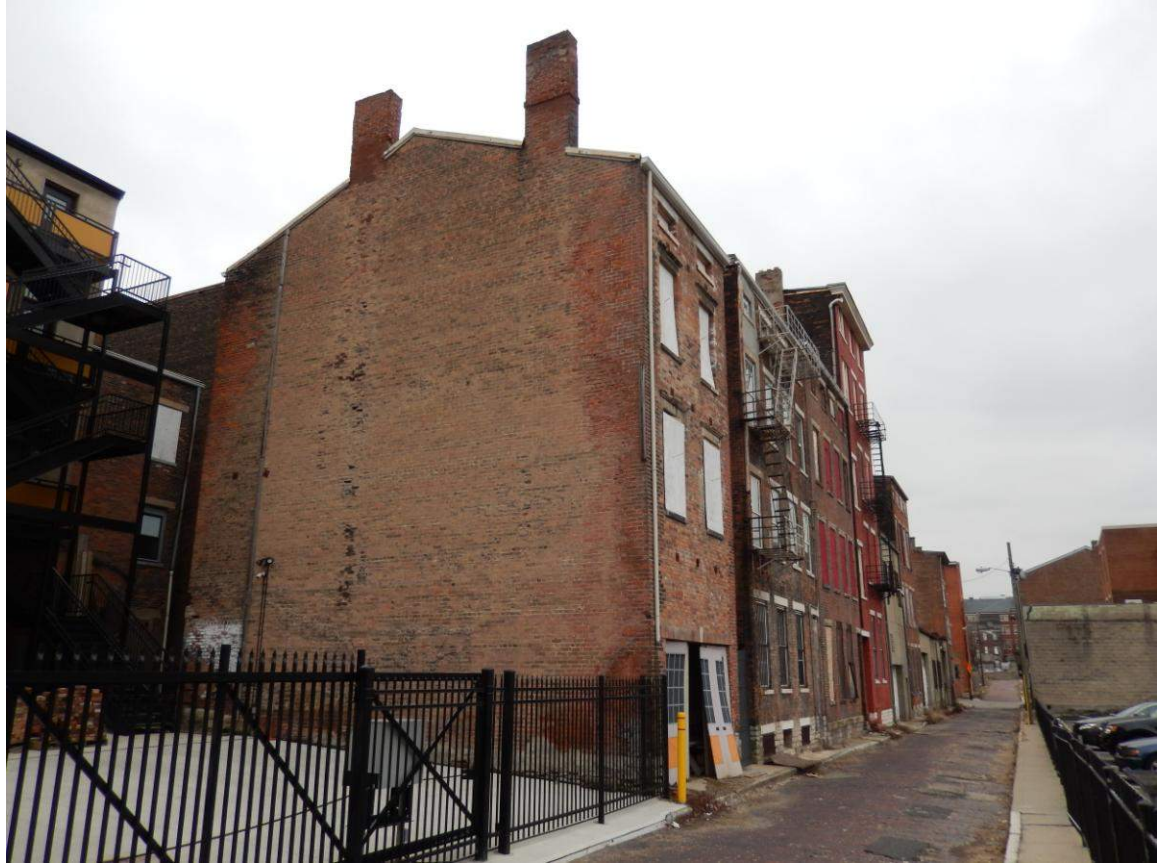
Rear Building - Along Campbell Alley (North & West Facades of Rear Building)
