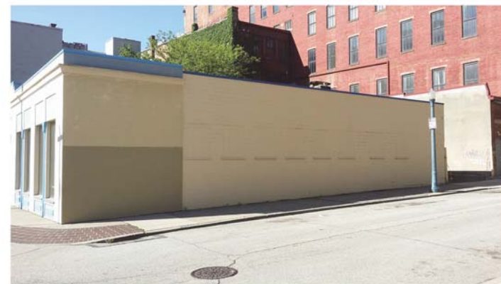
NORTH FACADE - PERRY STREET
