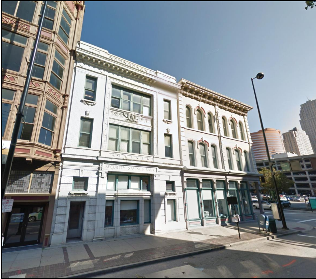
Figure 2. Image of 300 W. 4 th Street, facing northeast. Courtesy of Google.
