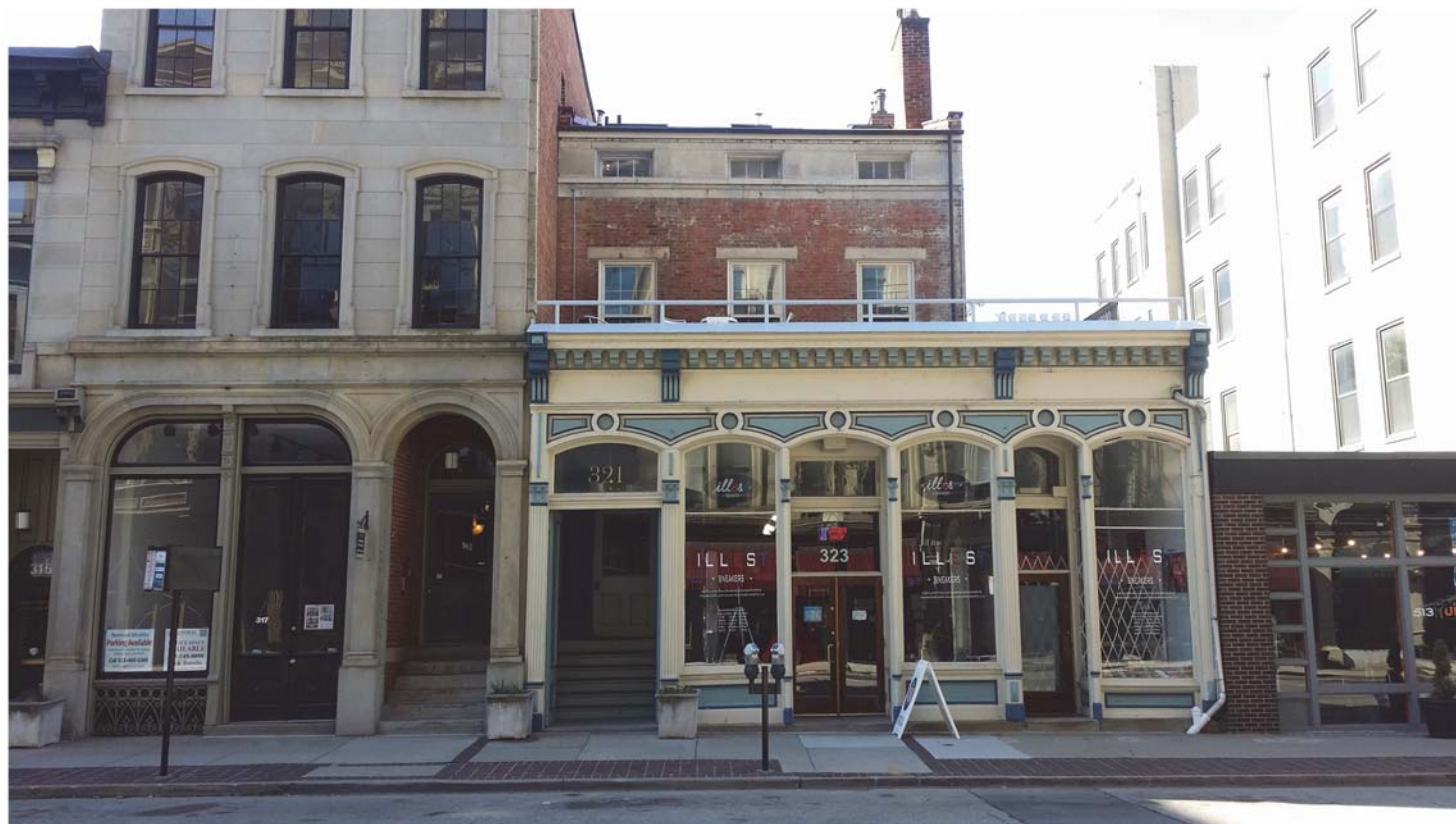
North Facade - 4th Street
