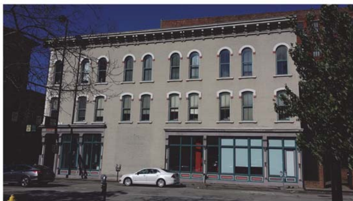
EAST FACADE - PLUM STREET
