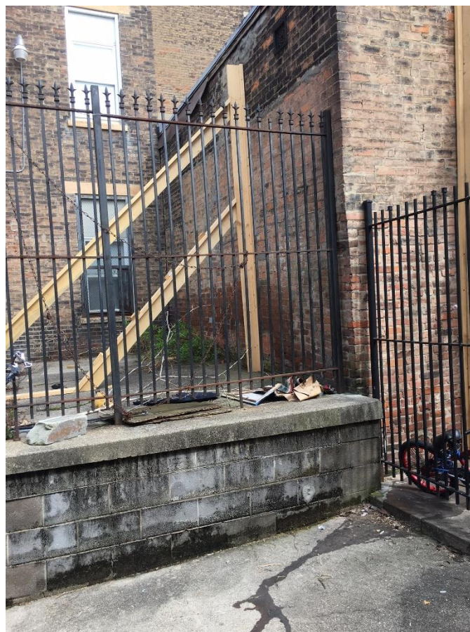
NW CORNER OF ADDITION
