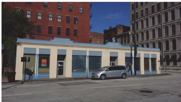
EAST FACADE - PLUM STREET
