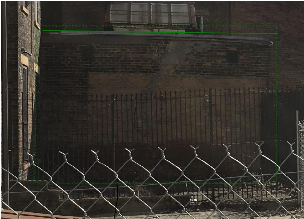
Elevation of the rear one story portion
