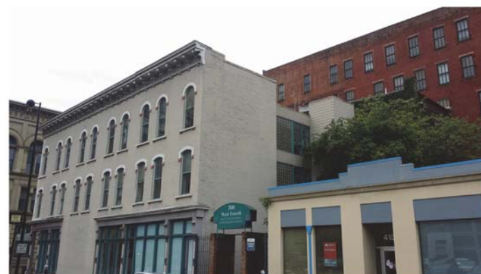
PARTIAL NORTH FACADE/ENTRY GATE
