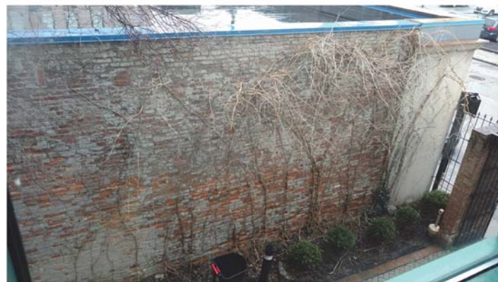
SOUTH FACADE / COURTYARD - PLUM STREET
