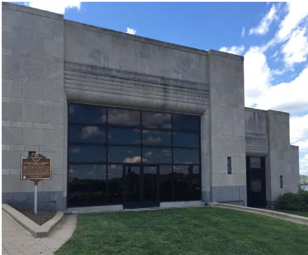
Existing view of north ramp portal.
