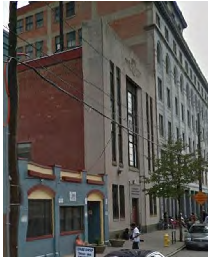
Teamsters building current Façade replacement believed to be circa 1940's
