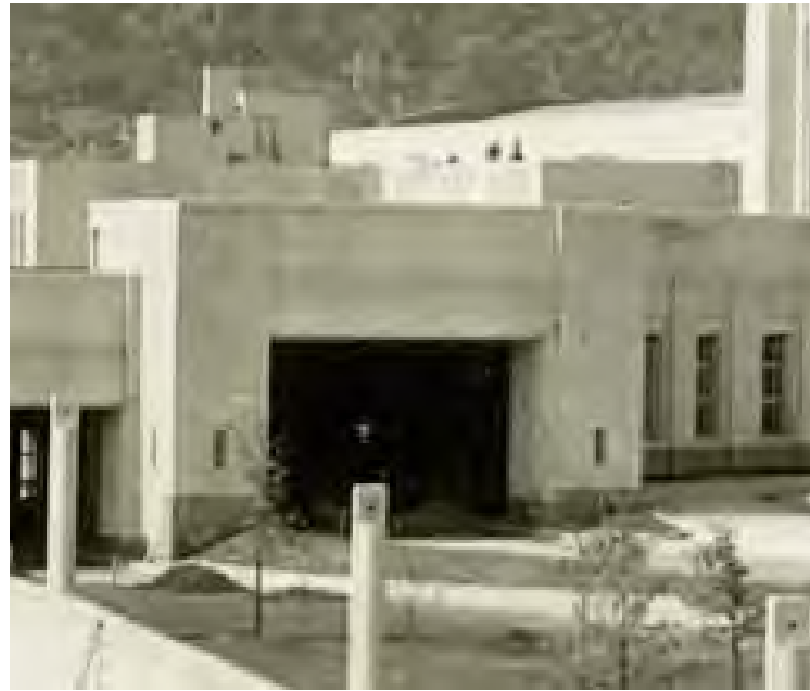
Historic view of south ramp portal
