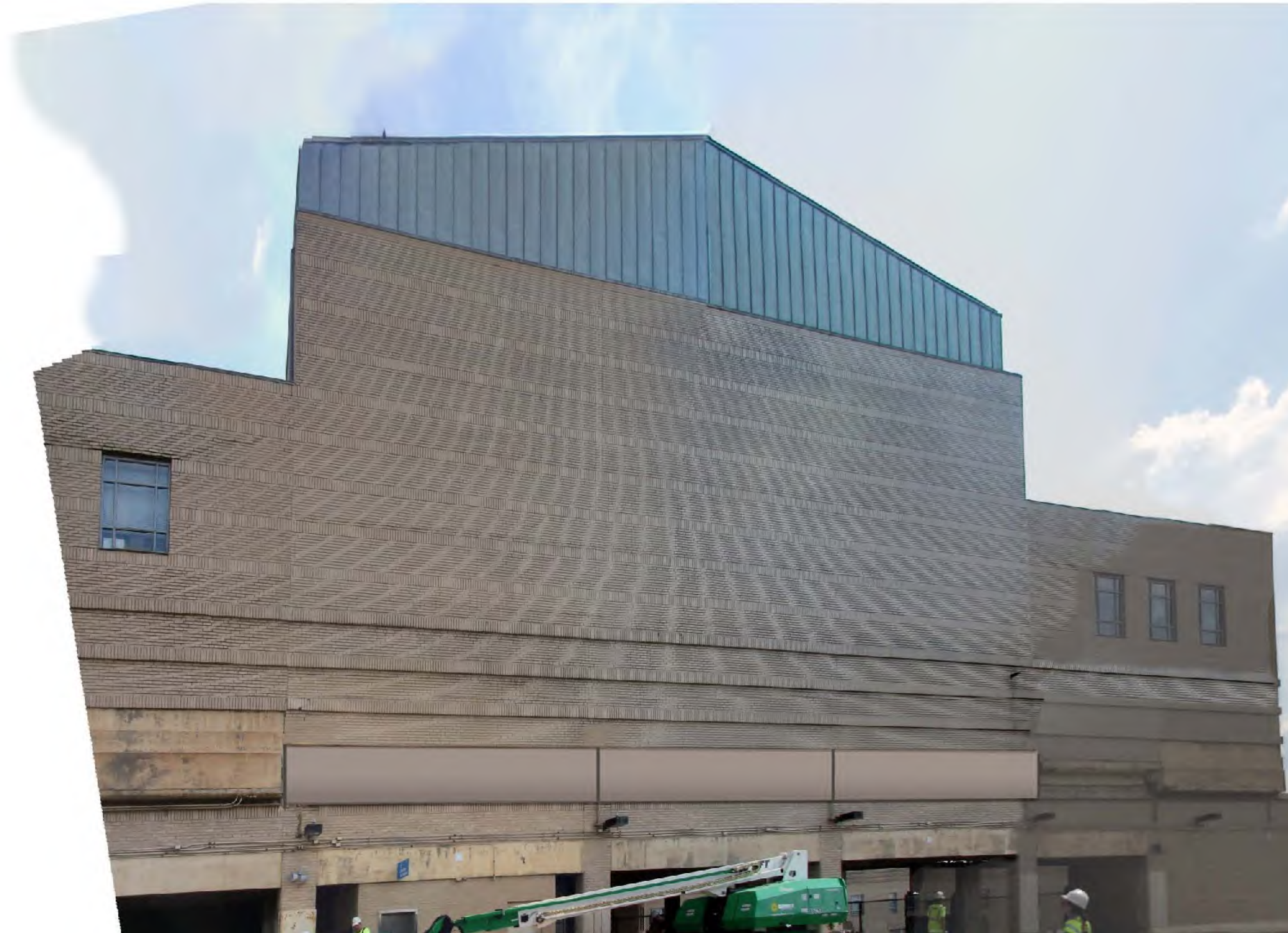
Rendering of rebuilt west elevation brick wall with existing metal west gable roof above.
