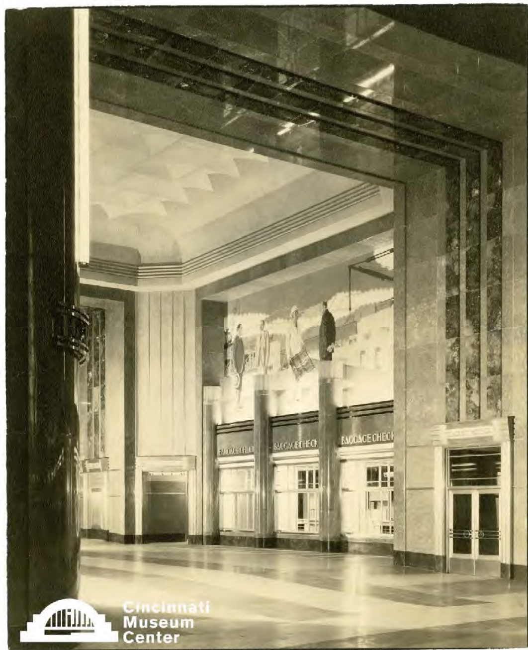
1930s photo of the Checking Lobby, looking northwest.
