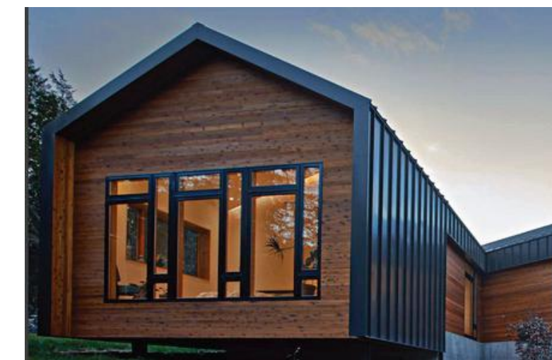
STANDING SEAM METAL CLADDING
