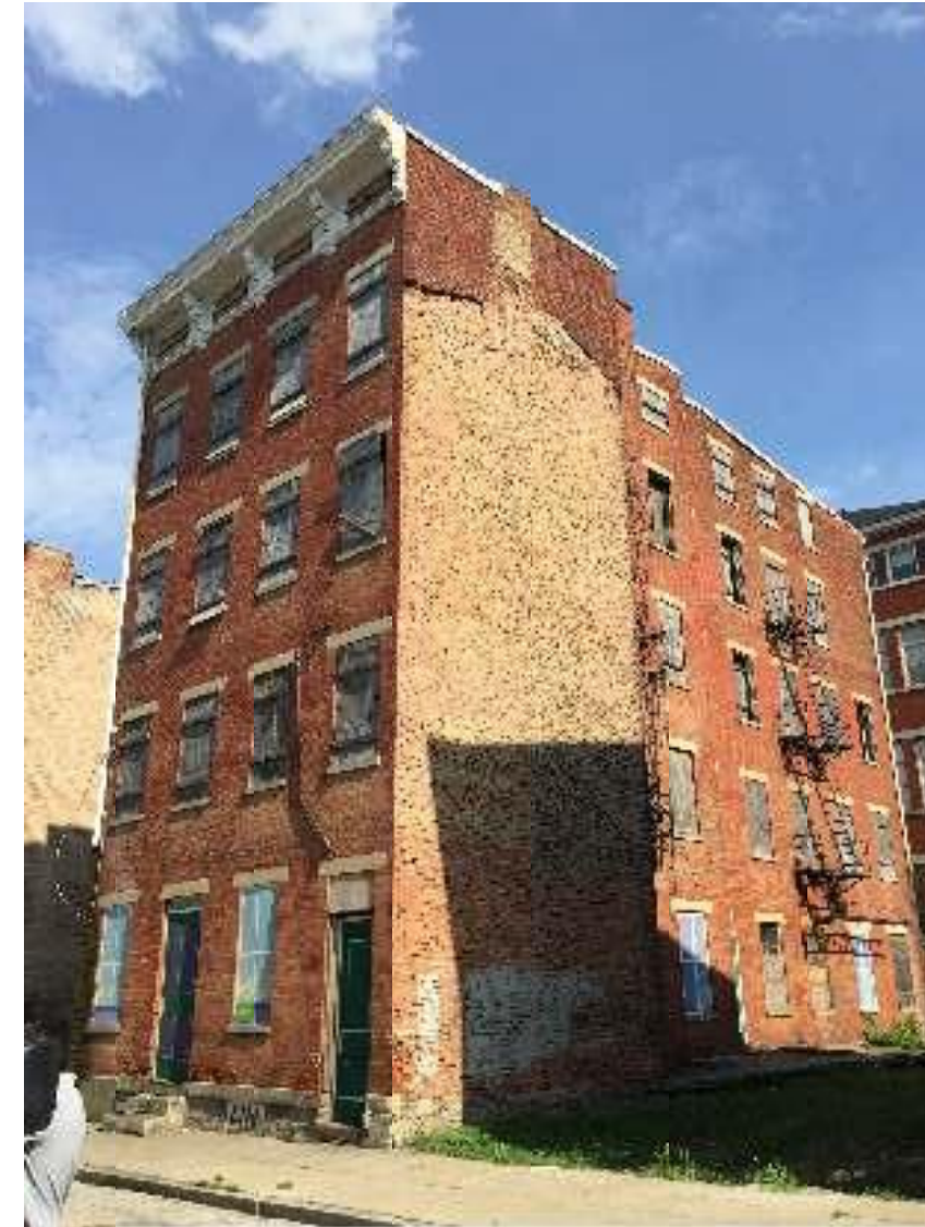
C WADE ST. PRIMARY FACADE
