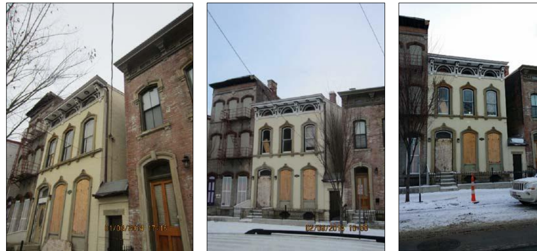
ELM STREET FRONT (WEST FACING)
