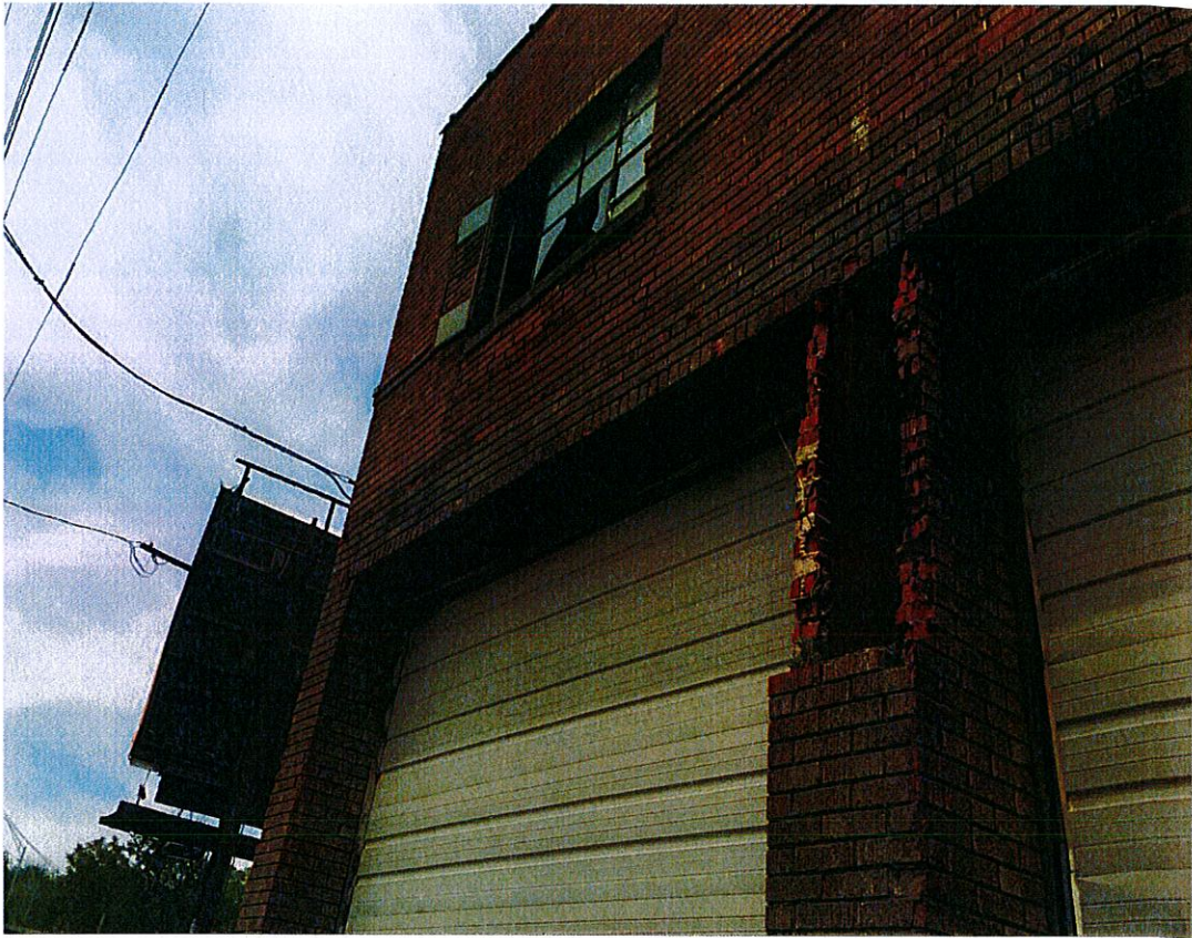
Photo 10 – Exterior West Building along Brewster.
