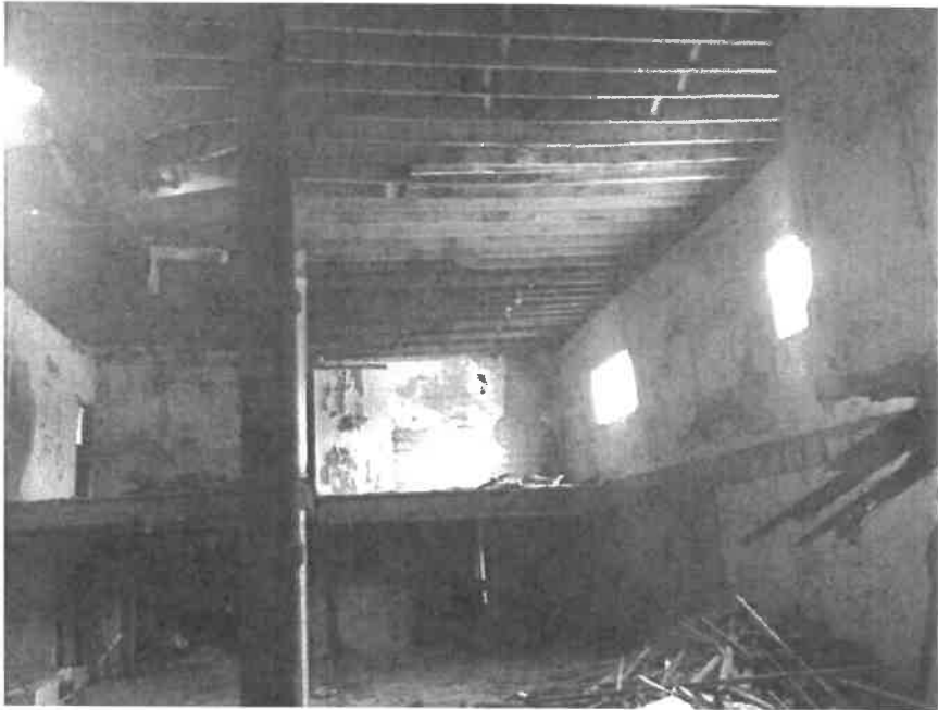
Photo 2 – West Building Interior.
