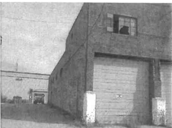
Subject South Elevation Wall (Photo Taken on September 23, 2015)
