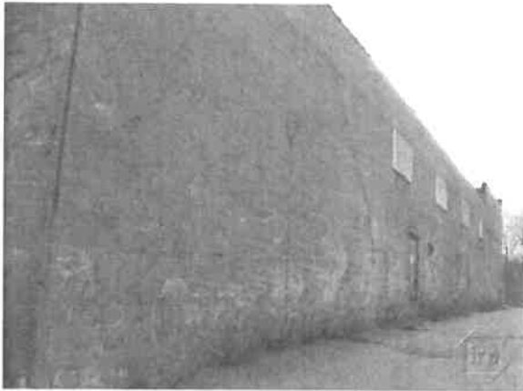
Exterior Elevation Facing NE (Photo Taken on January 20, 2017)
