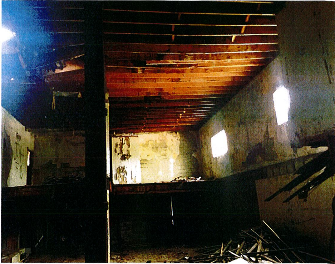
Photo 2 – West Building Interior.
