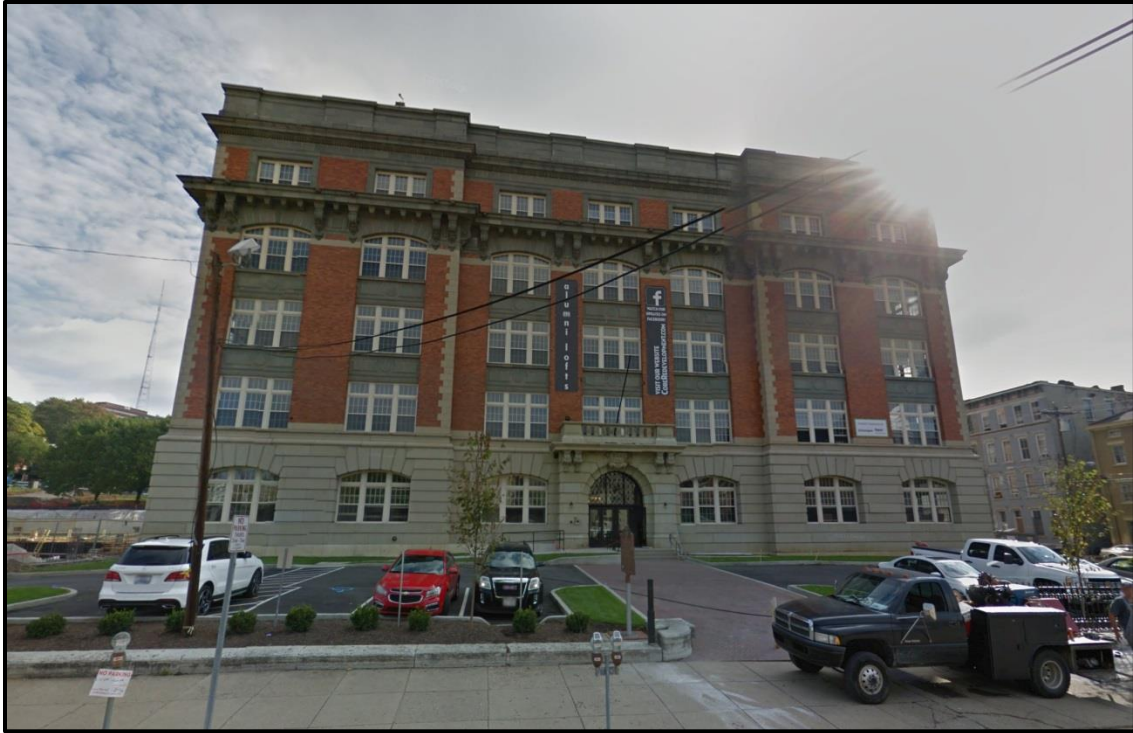
Figure 2. Existing condition of 1310 Sycamore Street. Image courtesy of Google.
