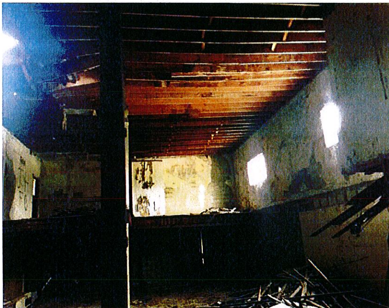
Photo 2 – West Building Interior.
