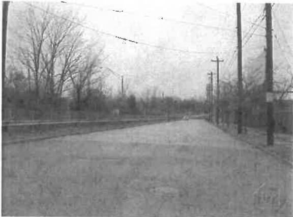
Brewster Avenue Facing South (Photo Taken on January 20, 2017)
