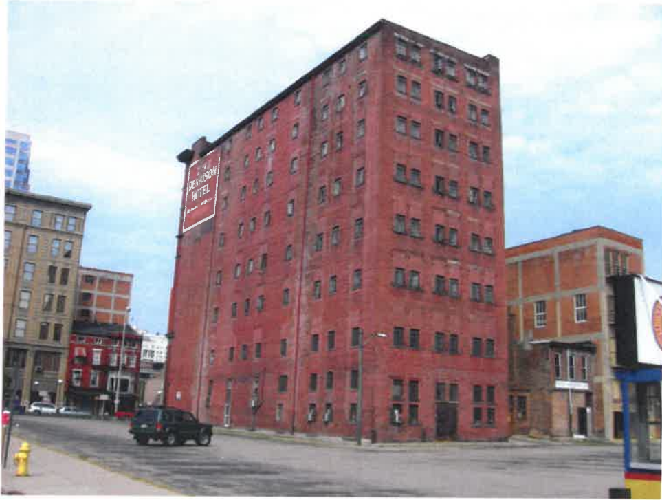
716-718 Main Street, South and East elevations
