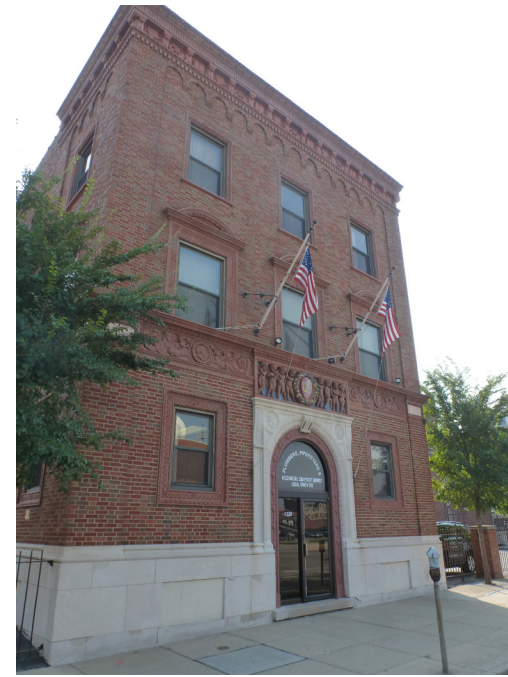
PLUMBER'S LOCAL UNION #392 (FORMERLY COLLEGE OF MUSIC ADMIN. BLDG.)
