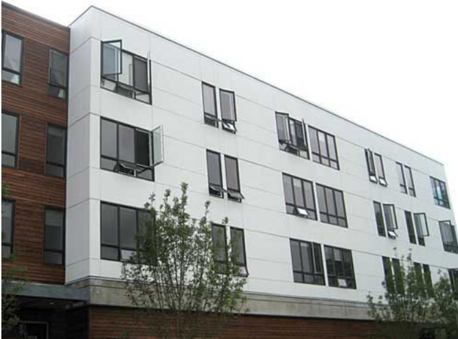
CEMENT FIBER PANEL (PAINTED) AND ALUMINUM WINDOWS
