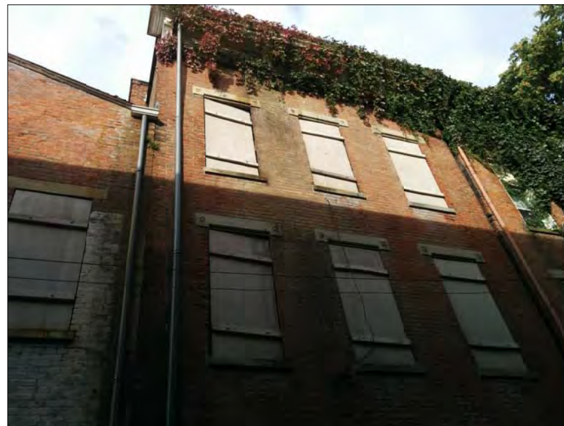
East Facade 2 - from Goose Alley
