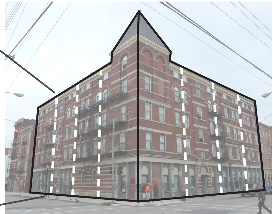
Typical corner OTR building
