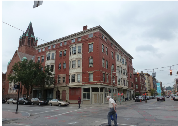
Typical corner OTR building
