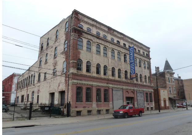
Typical commercial OTR building
