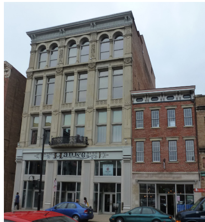
Variation in height and floor heights- Main St.
