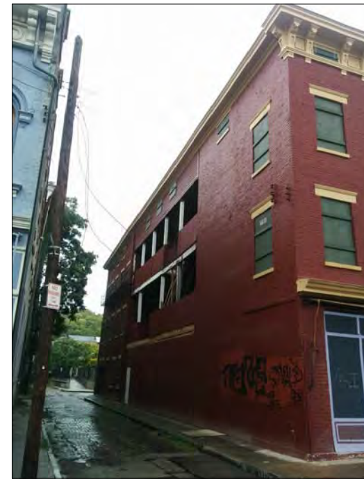
West Facade - NE View
