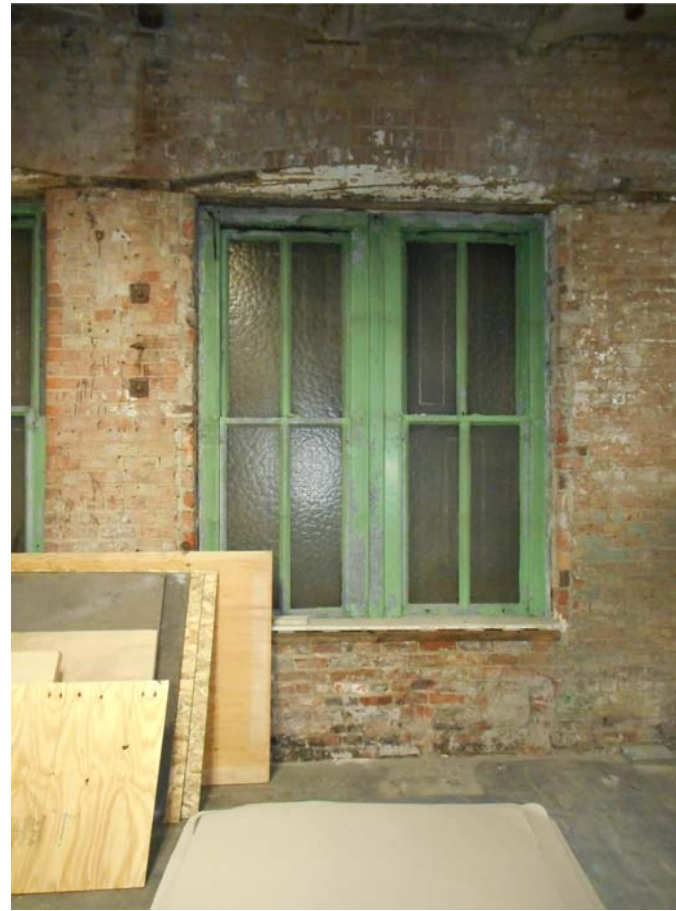
2 5 Existing Wood Window NTS
