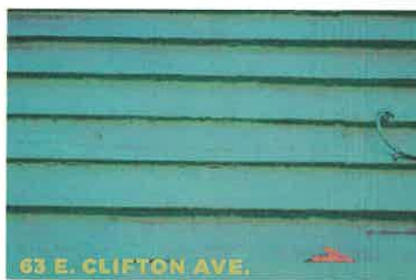
Horizontal Emphasis, shadow line, wood texture, variation in boards, approximately 1/2" thick boards typically 4-6" wide
