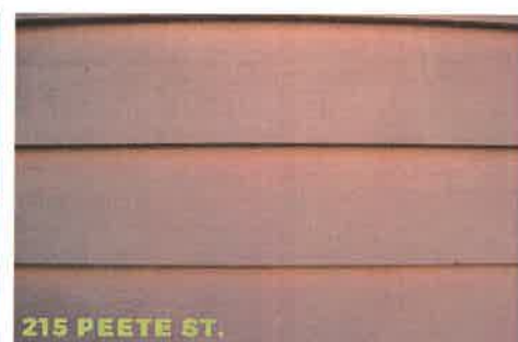
Horizontal Emphasis, shadow line, wood texture, variation in boards, approximately 1/2" thick boards typically 4-6" wide
