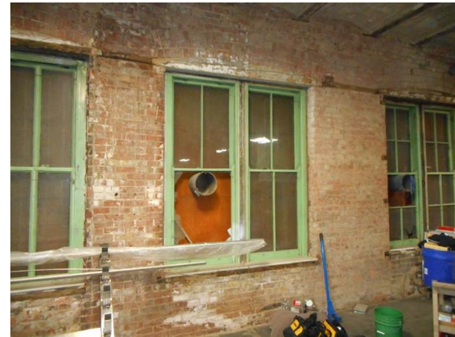
5 5 Existing Metal Window NTS
