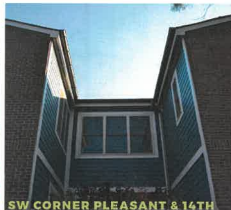
Horizontal emphasis, small shadow line, uniform look, typical smooth texture, 5/16" thick with various board widths
