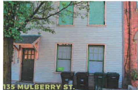
Horizontal emphasis, small shadow line, uniform look, typical smooth texture, 5/16" thick with various board widths
