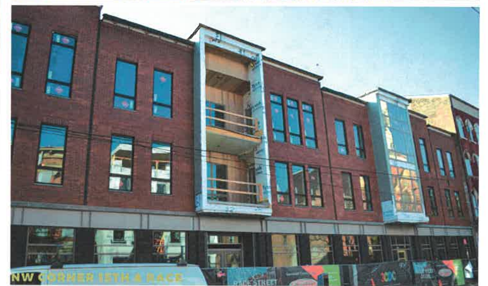
Brick with fiber cement lap siding & wood shiplap siding; metal panel with horizontal emphasis, brick with metal panel appearing as wide flat siding & vertical wood siding
