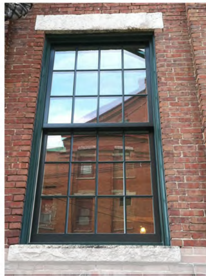
DOUBLE HUNG WINDOW SAMPLE INSTALLATION
