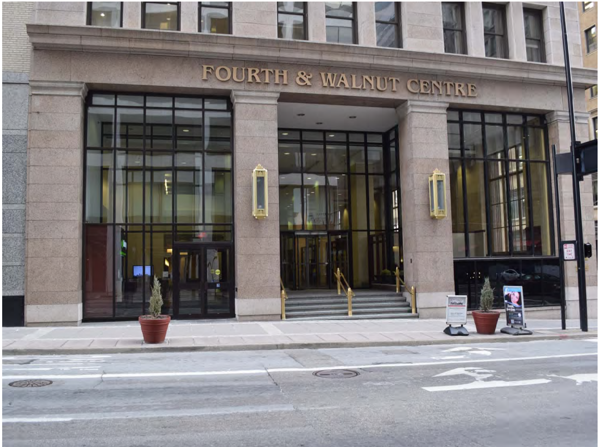
3. Detail of north facade on Fourth Street
