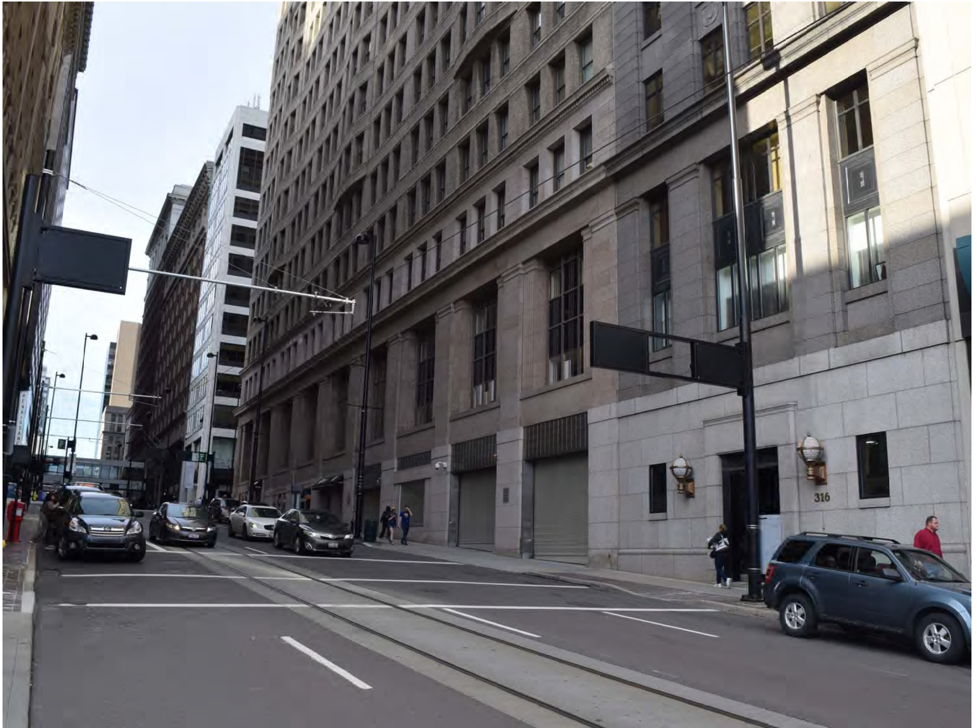
7. West facade looking northeast on Walnut Street
