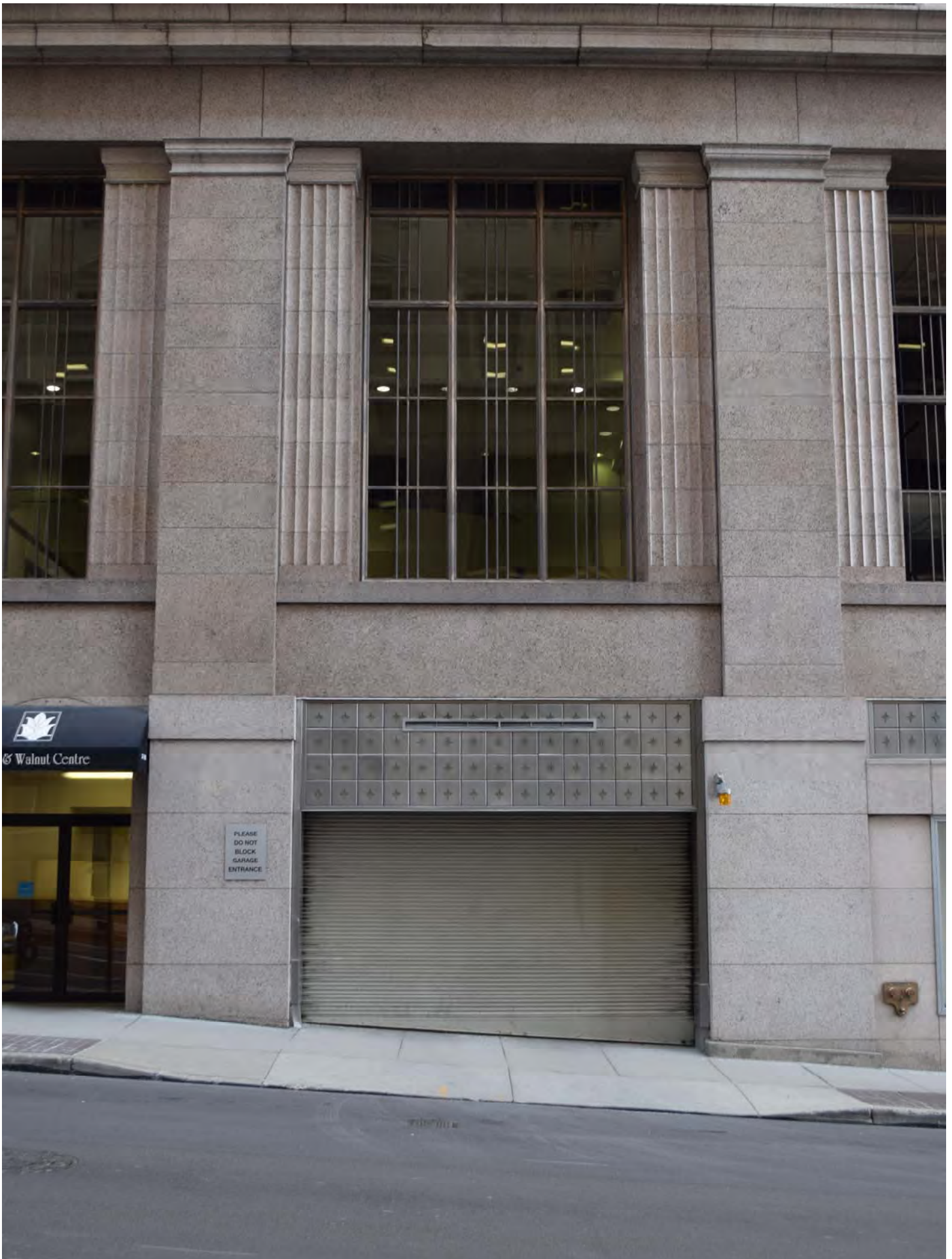
8. Detail of west facade bay at Walnut Street
