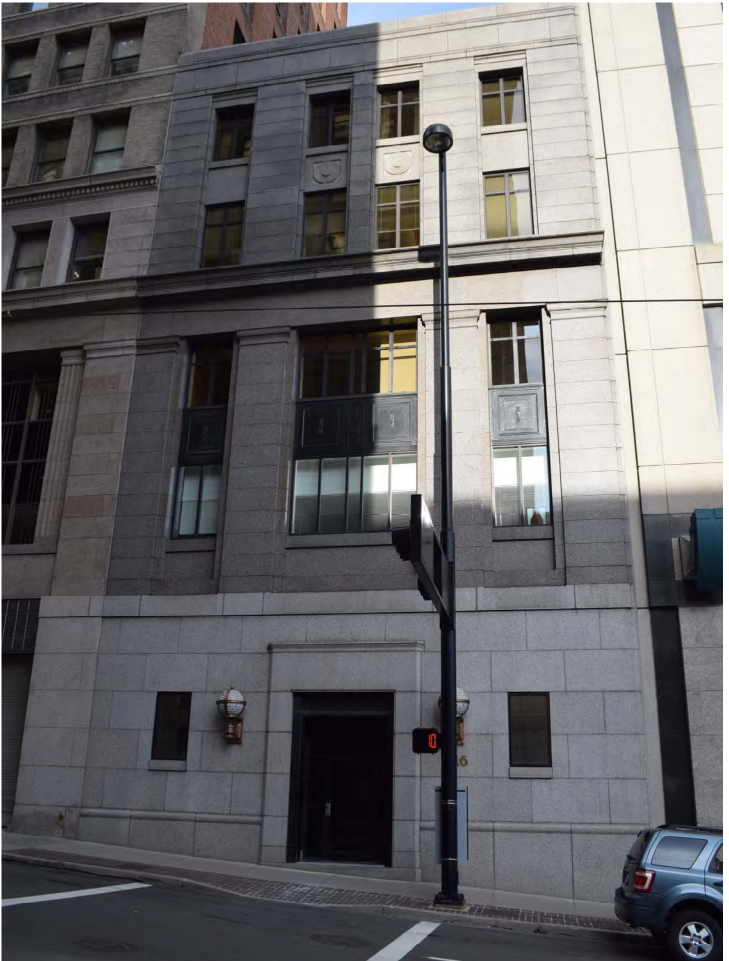
10. West facade of addition on Walnut Street
