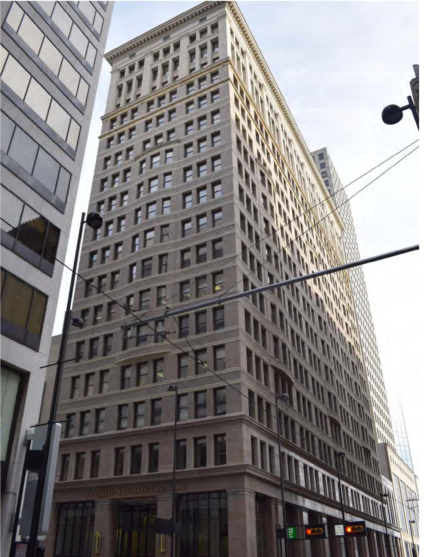
1. North and West facade looking south on Walnut
