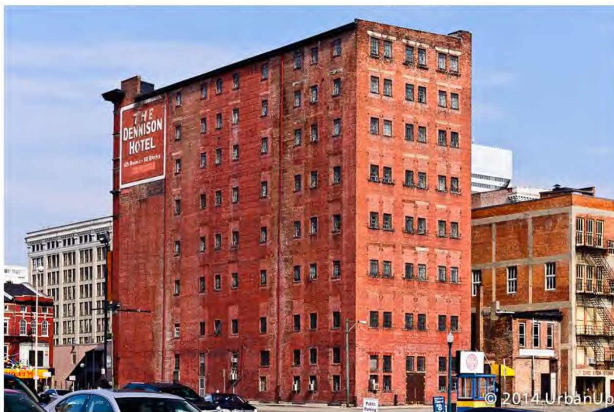
Rearview of the Dennison Hotel building
