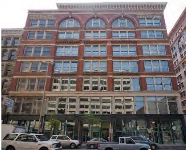
Hopper Building 139-151 W 4 th St: Samuel Hannaford Designed Building.
