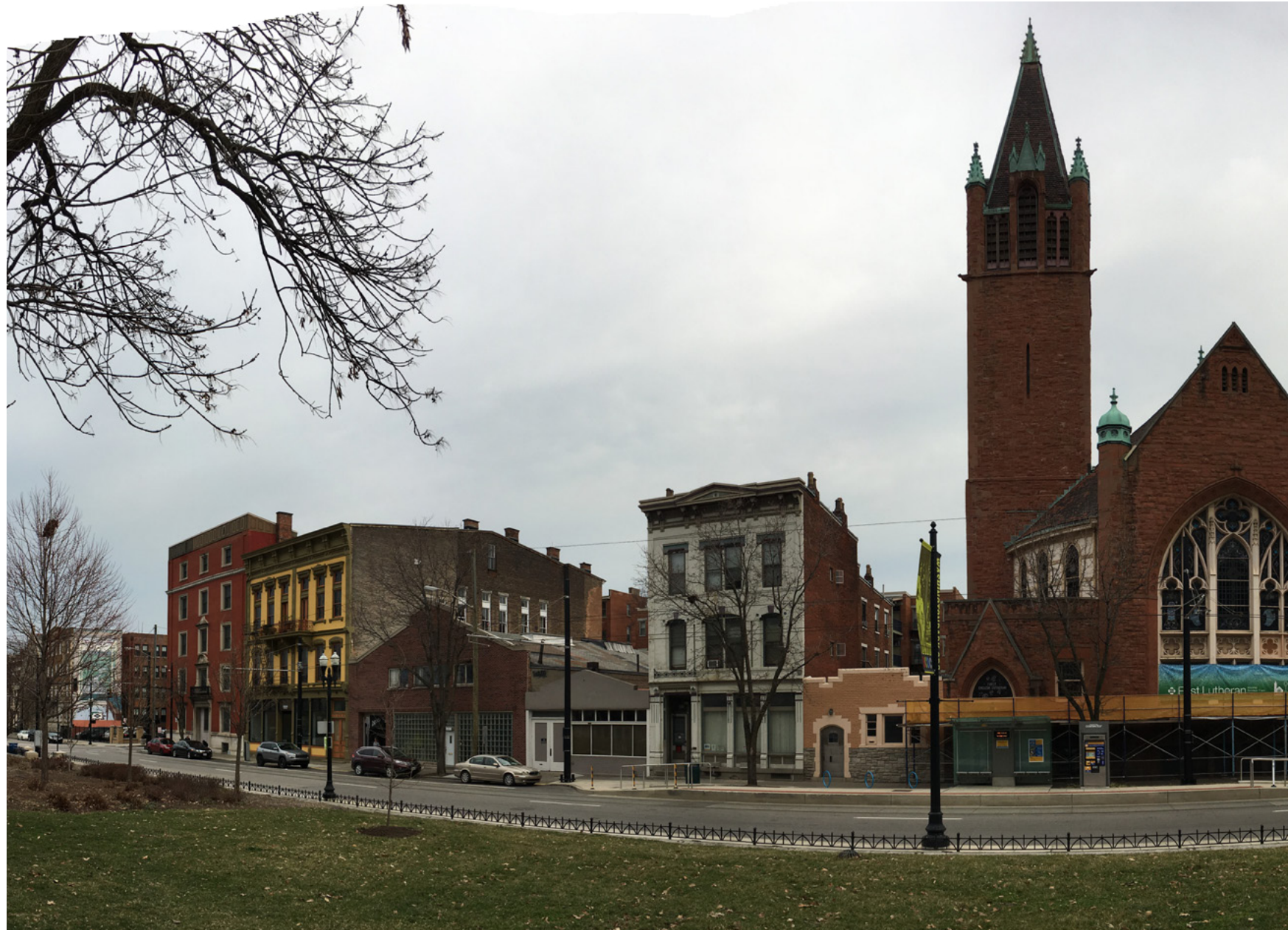
FRONT-OF-SITE PHOTO COLLAGE - Looking NE
