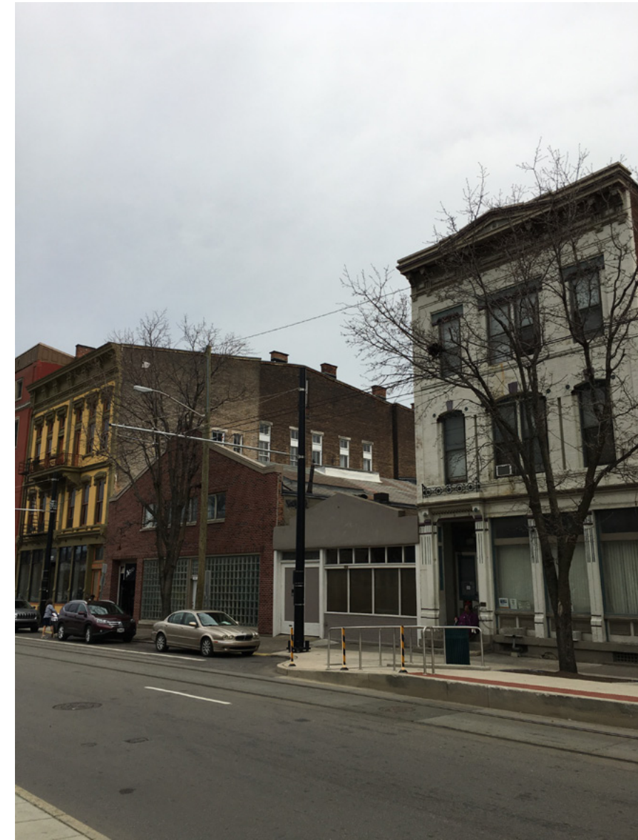
FRONT-OF-SITE PHOTO - Looking N
